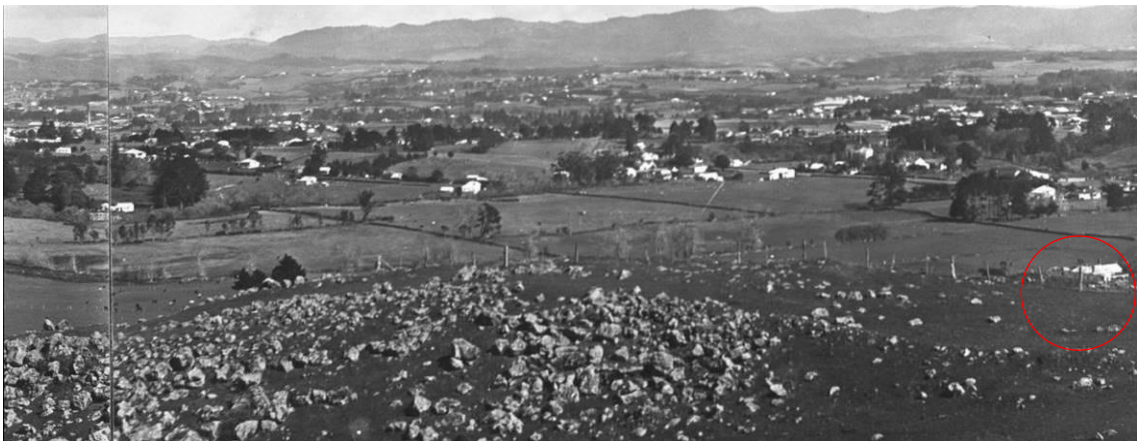
Figure 10: 3 Sep 1920. Panoramic view looking west south west from Mount Albert showing Owairaka in the background. Image source: Sir George Grey Special Collections, Auckland Libraries, 4-4421
