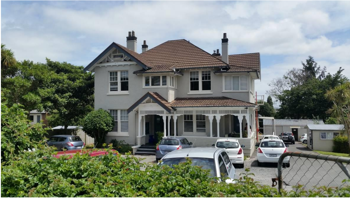
Figure 16: Showing the street (east) façade of the house at 103 Richardson road. Image source: Burgess Treep & Knight 2016
