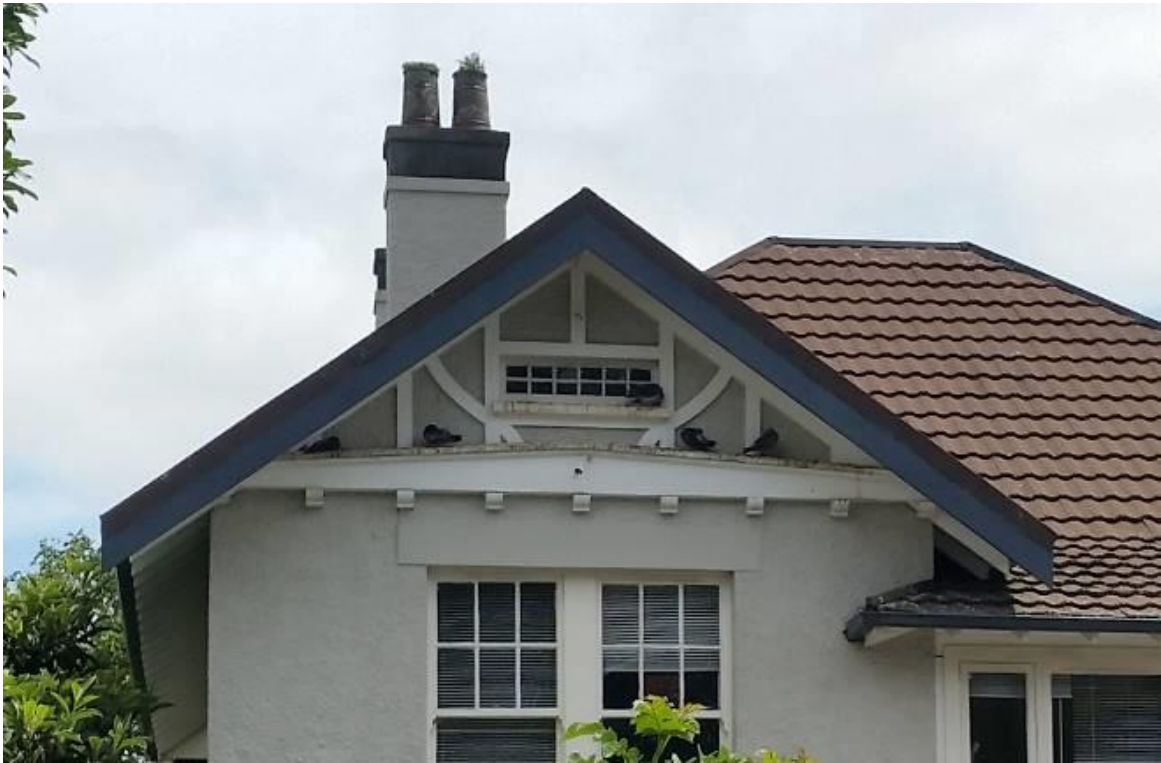
Figure 20: Showing the gable end detail on the east (street) façade of the house at 103 Richardson road. Image source: Burgess Treep & Knight 2016
