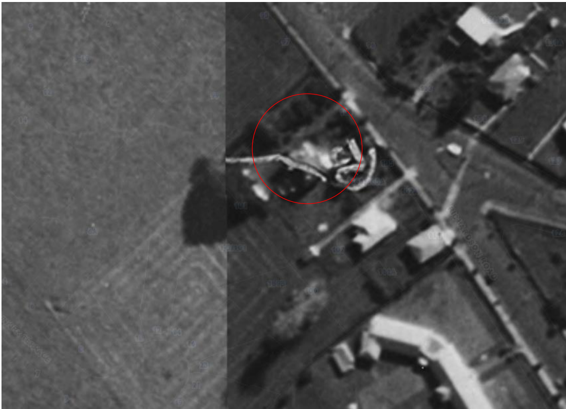
Figure 13: 1940 aerial photograph of the property. Image source: Auckland Council GIS Viewer 2016
