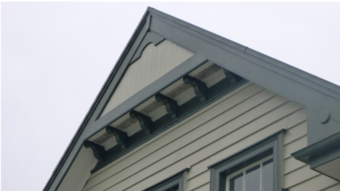
Figure 45: In-filled gable detail with tongue and groove panels (Auckland Council; 24/08/2016)
