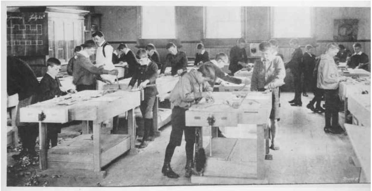
Figure 56: Boys during a woodwork class at Richmond Road Manual Training School 1903 (NZ Graphic 1 August 1903 P. 322)
