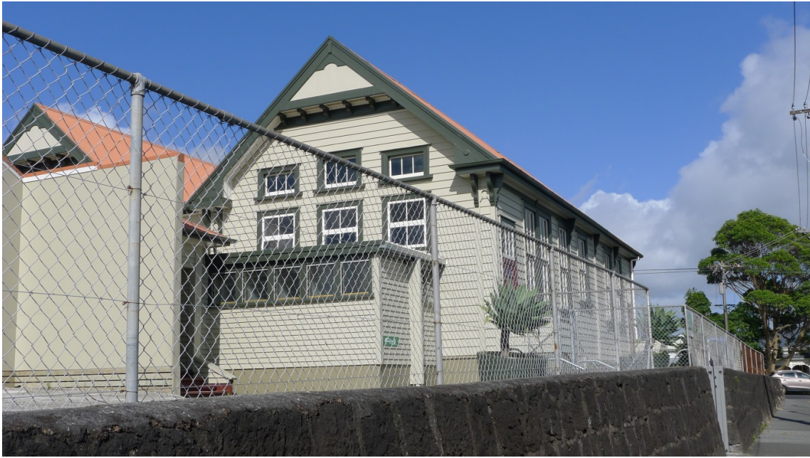
Figure 48: Eastern elevation and toilet block extension (Auckland Council; 05/10/2016)
