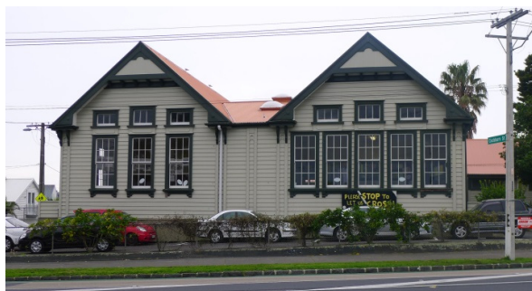
Figure 5: Western elevation showing sashes and fanlights (Auckland Council; 24/08/2016)
