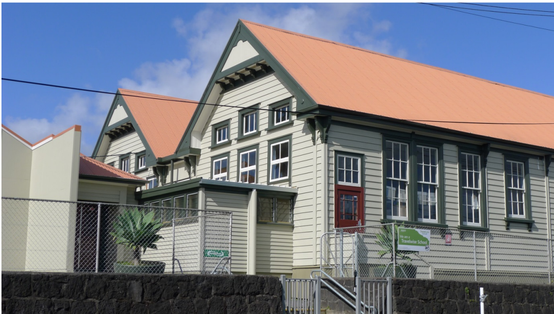
Figure 47: Eastern (rear) elevation (Auckland Council; 05/10/2016)
