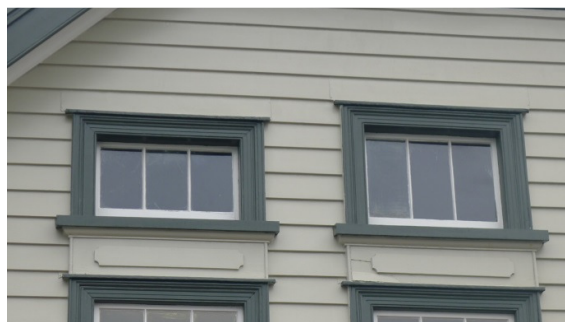
Figure 6: Detail of fanlights (Auckland Council; 24/08/2016)
