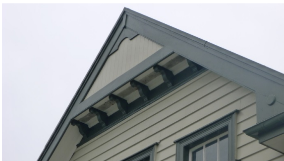
Figure 3: Detail of gable (Auckland Council; 24/08/2016)
