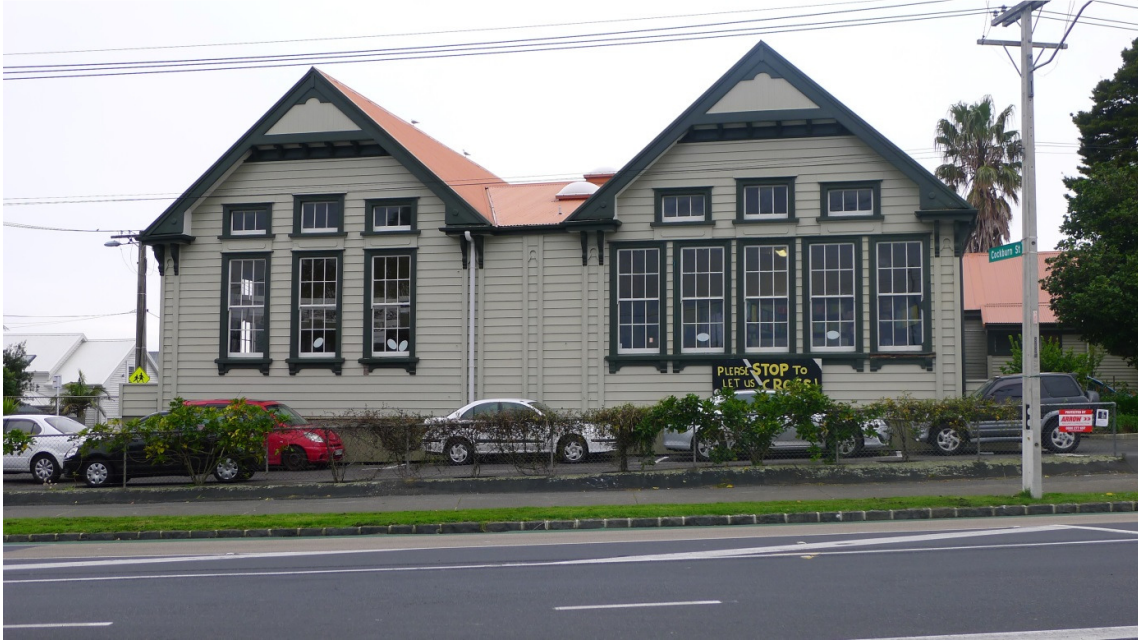
Figure 42: Richmond Road Manual Training School, western elevation (Auckland Council; 24/08/2016)
