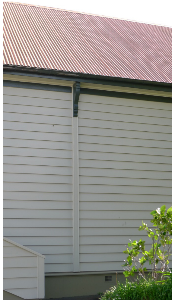
Figure 52: Detail of vertical battens and eaves bracket) (Auckland Council; 05/10/2016)
