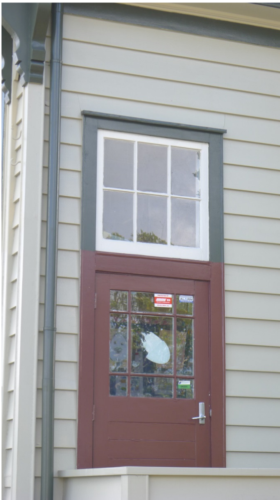
Figure 51: Detail of door (Auckland Council; 05/10/2016)
