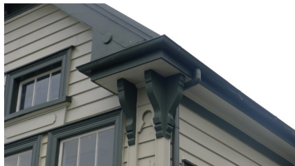
Figure 4: Detail of boxed, brackets eaves and roundels (Auckland Council; 24/08/2016)
