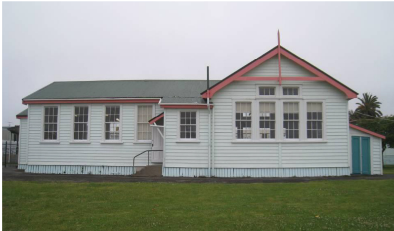
Figure 15: Otahuhu Primary School Technical Block located at 41 Station Road, Otahuhu (Matthews & Matthews; 08/2013)
