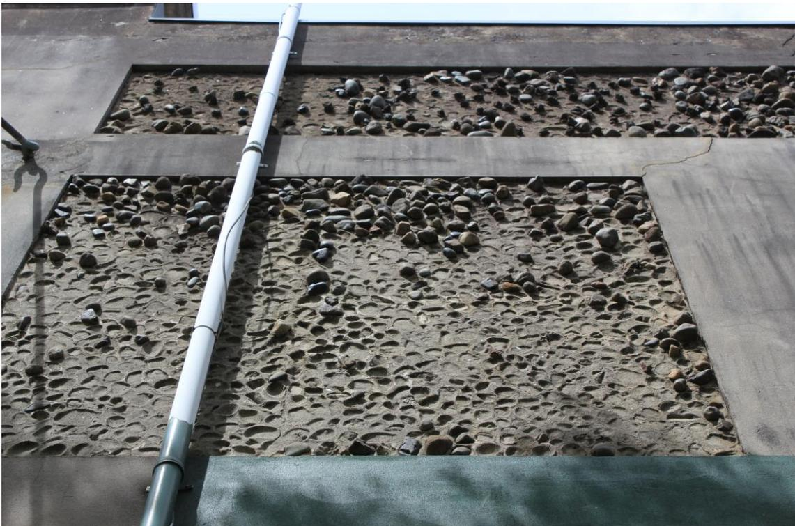
**Figure 20:** North elevation showing condition of river stone stucco panels where about 75% of cobbles have detached.
