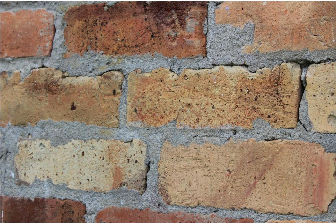
**Figure 24:** South elevation, typical buff brickwork condition. Small areas have been repointed in Portland cement.
