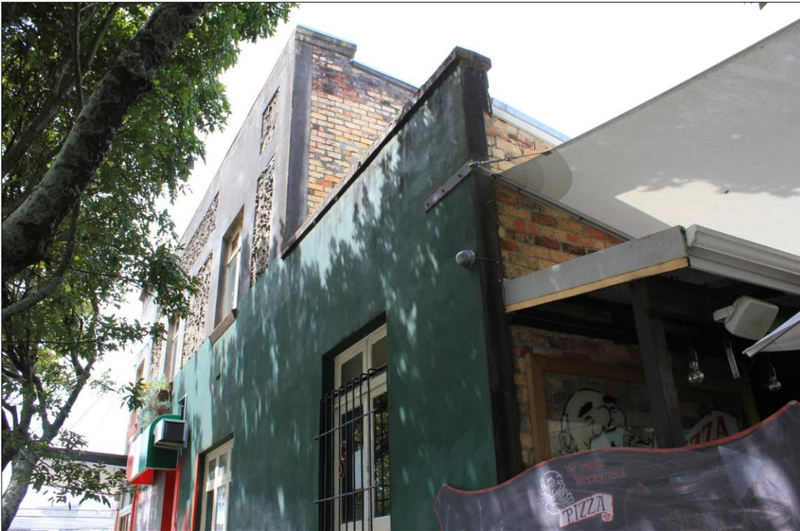
**Figure 19:** North elevation looking towards Eden Park showing the step down to single storey section and un-rendered brick construction at rear.
