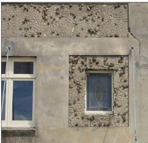
**Figure 15:** Detail, east elevation showing river stone stucco panels on parapet and surrounding a leaded glass window.
