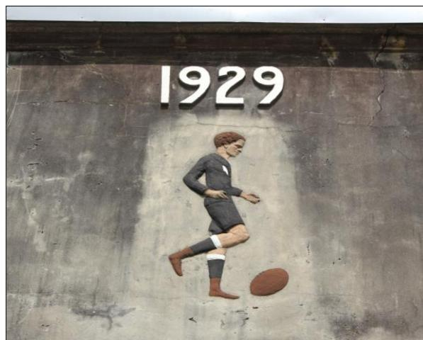
**Figure 16:** Stucco All Black on the corner elevation. The surrounding pale buff mortar background was cleaned for the 2011 Rugby World Cup and the relief figure re-painted.
