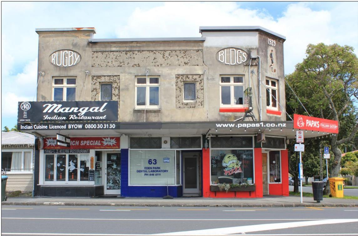
Figure 17: East elevation to Sandringham Road. Note stucco repairs on right side of parapet.
