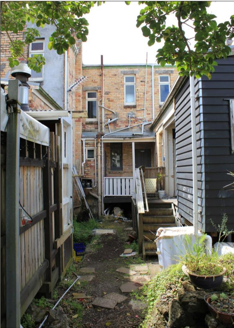
**Figure 21:** Looking east at rear wall of central tenancy showing original rear verandah entrance and later timber addition.
