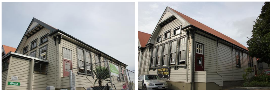
Figure 8: Above, views from the northeast (left) showing rear lean-to and southwest (right) showing additional doors and windows on gable end and south elevation. Photo: Reynolds & Associates.
