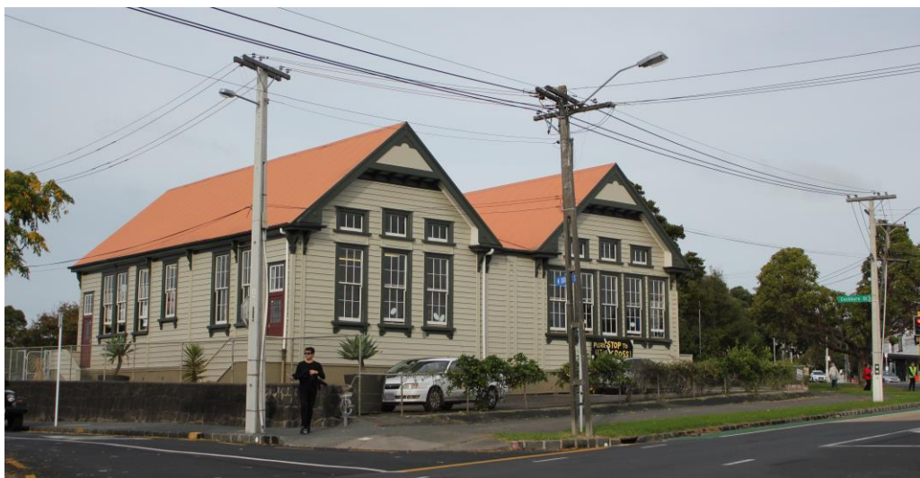
Figure 6: The former Richmond Road Manual Training School building, on the corner of Douglas Street and Richmond Road in May 2016. Photo: Reynolds & Associates.
