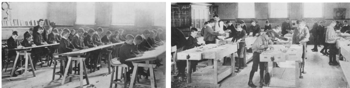
Figure 13: Two views inside the woodwork room at Richmond Road Manual Training School shows a drawing class at work (left) and boys at workbenches. Source: NZ Graphic 1 August 1903 pg. 322
