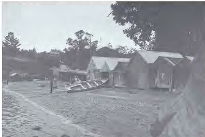
View in 1896 of boatsheds in Judges Bay, Auckland. While these particular sheds no longer exist the typical building form remains a familiar sight in many other locations. Auckland City Libraries 1-W 188.
