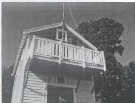
West elevation. Note bungalow features including exposed rafters at the eaves and timber shingles in the gable end. The deck has been reconstructed but is similar to the original (DPAL).
