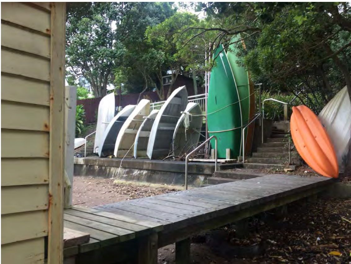
Figure 31: View of the wooden boardwalk connecting the building to the embankment. 15 November 2016, Anna Boyer.
