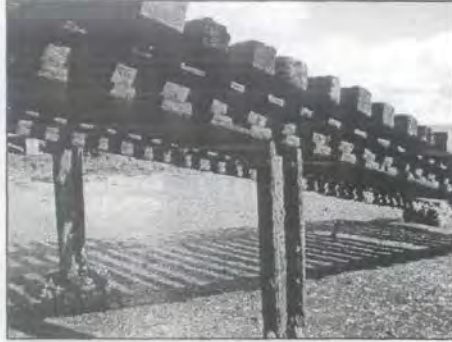
Ramp. Note railway line runners and supports (DPAL).
