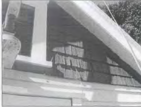
Deteriorated shingles in west gable end.
