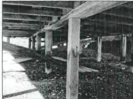
Subfloor. Note diagonal braces (DPAL).
