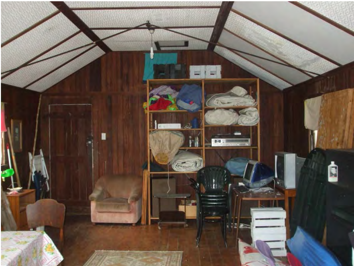
Figure 21: First floor interior, 2009. Images from ARC property file
