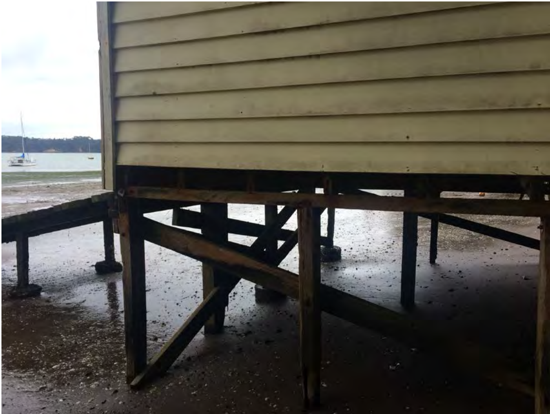
Figure 30: Detail showing piles and struts. 15 November 2016, Anna Boyer.
