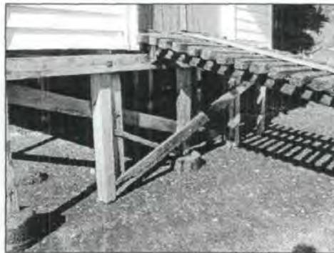
Timber piles and braces. Note replacement piles. Brace has decayed.
