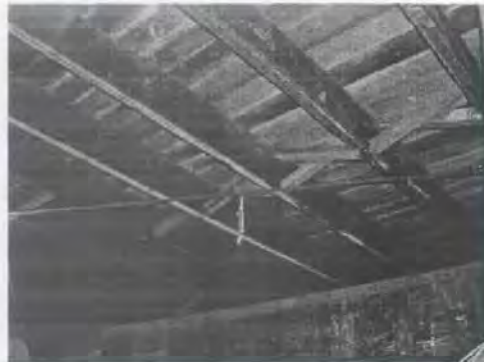
Upper floor framing. Note herring bone strutting (DPAL).
