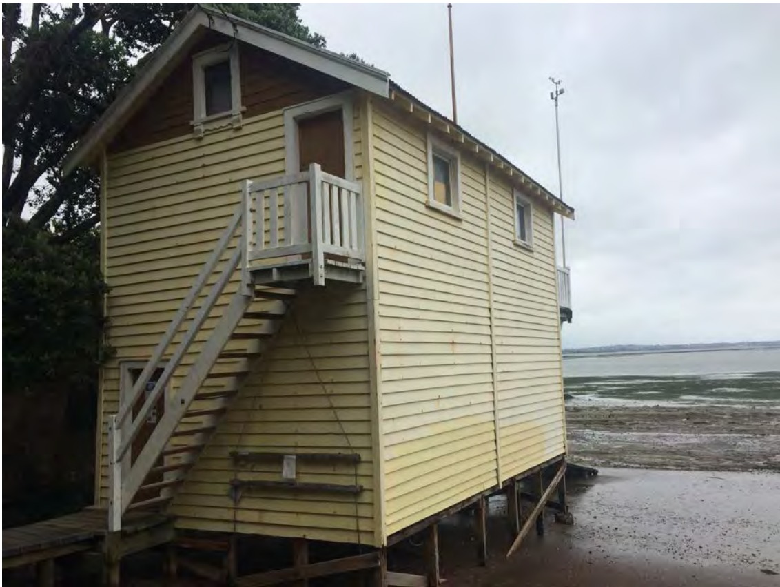
Figure 33: View of the boatshed from the embankment. 15 November 2016, Anna Boyer.
