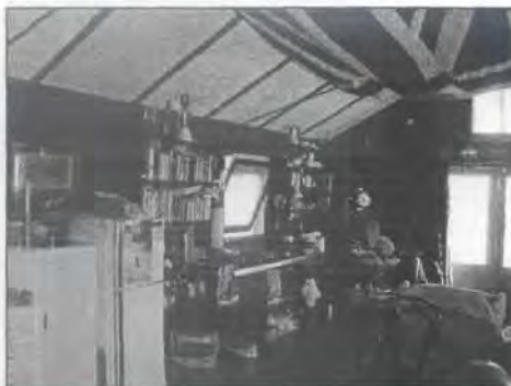
Upper level interior. Note tongue and groove wall linings (DPAL).
