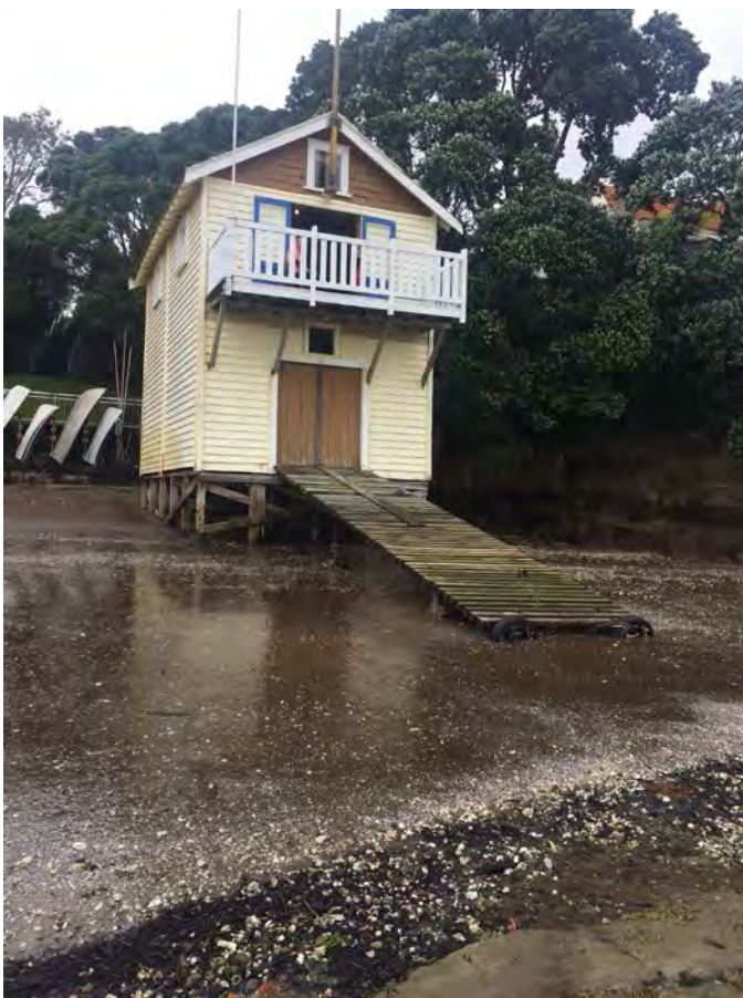
Figure 27: View of the north west elevation of the boatshed. 15 November 2016, Anna Boyer.
