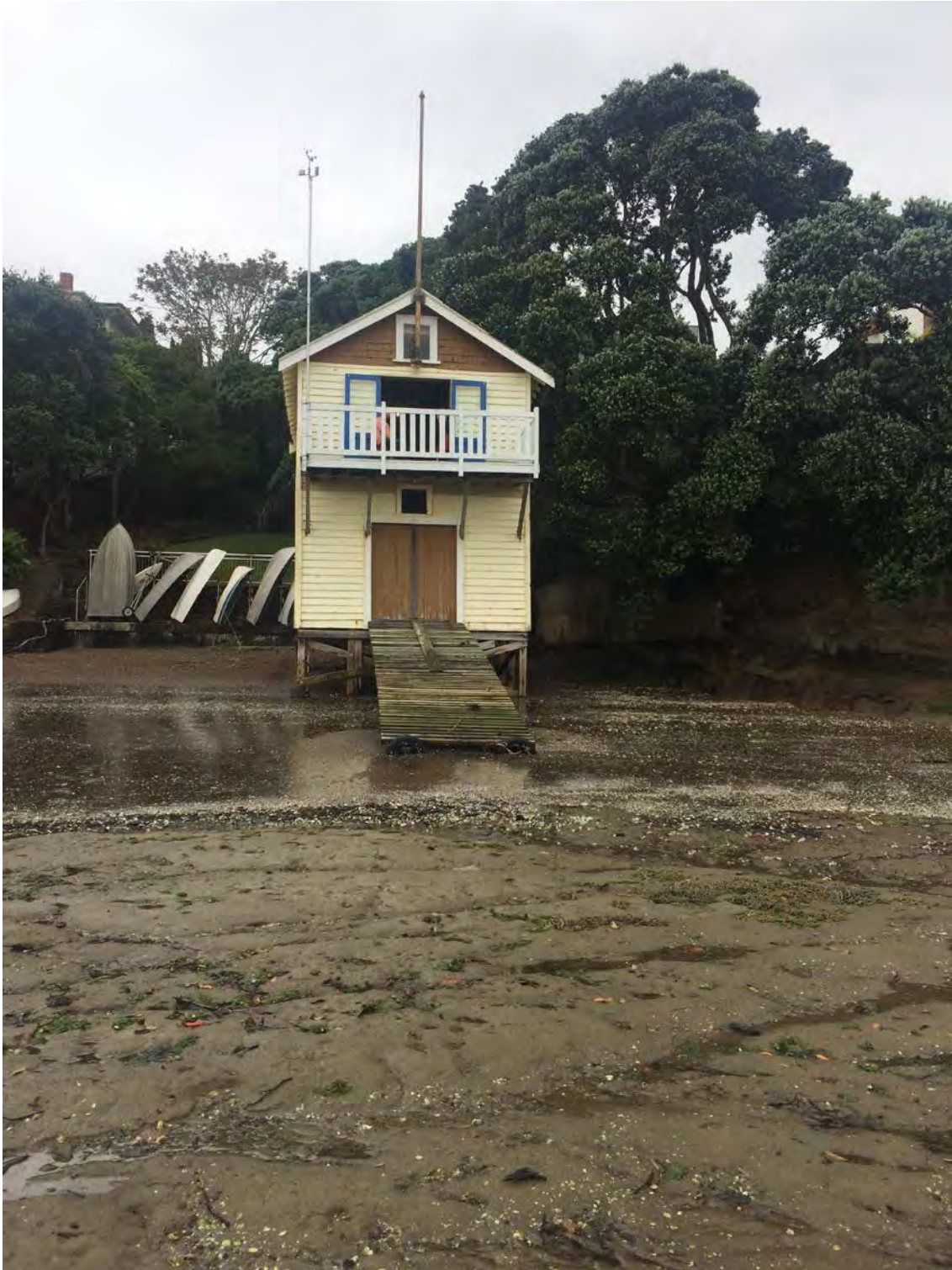
Figure 28: View of the north west elevation of the boatshed. 15 November 2016, Anna Boyer.
