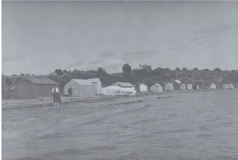
View of St Heliers Bay in 1911, showing boatsheds along the shoreline. These no longer remain, the foreshore having been modified by the construction of Tamaki Drive which opened in 1931. Auckland City Libraries 1-W127.
