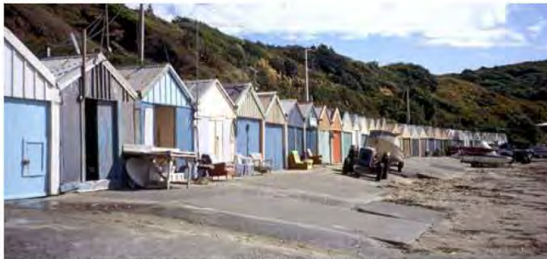
Boatsheds in Titahi Bay in Wellington are a local landmark. Image source: Te Ara
