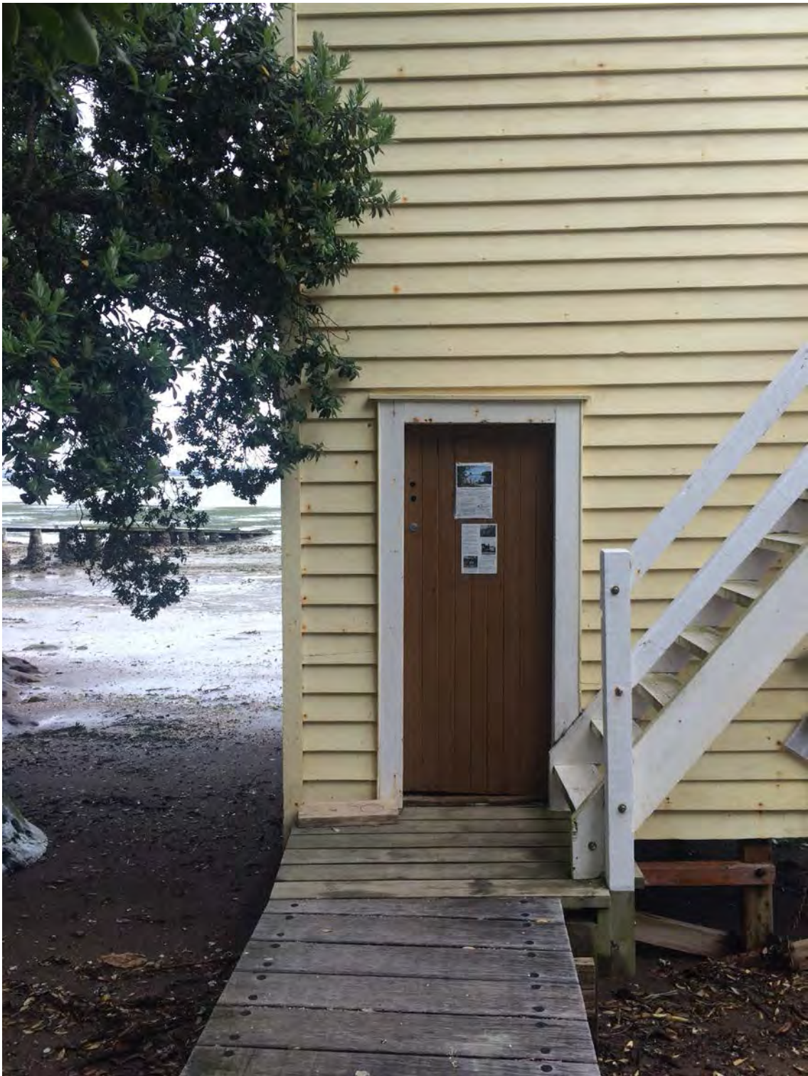
Figure 32: Front door and stairs. 15 November 2016, Anna Boyer.
