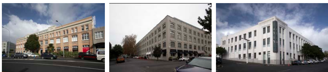
Figure 11: the former NZ Loan and Mercantile Wool Store, the NZSC, FCAC & NAFC buildings and the Axis Building.
