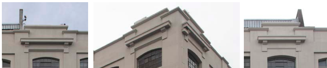
Figure 6: Shows decorative cornice elements on the North Auckland Farmers' Cooperative building (St Georges Bay Road, St Georges Bay Road/Faraday corner, Faraday Street)
