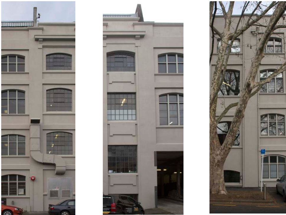
Figure 7: Shows party wall between buildings (St Georges Bay Road, Faraday Street, Kenwyn Street)
