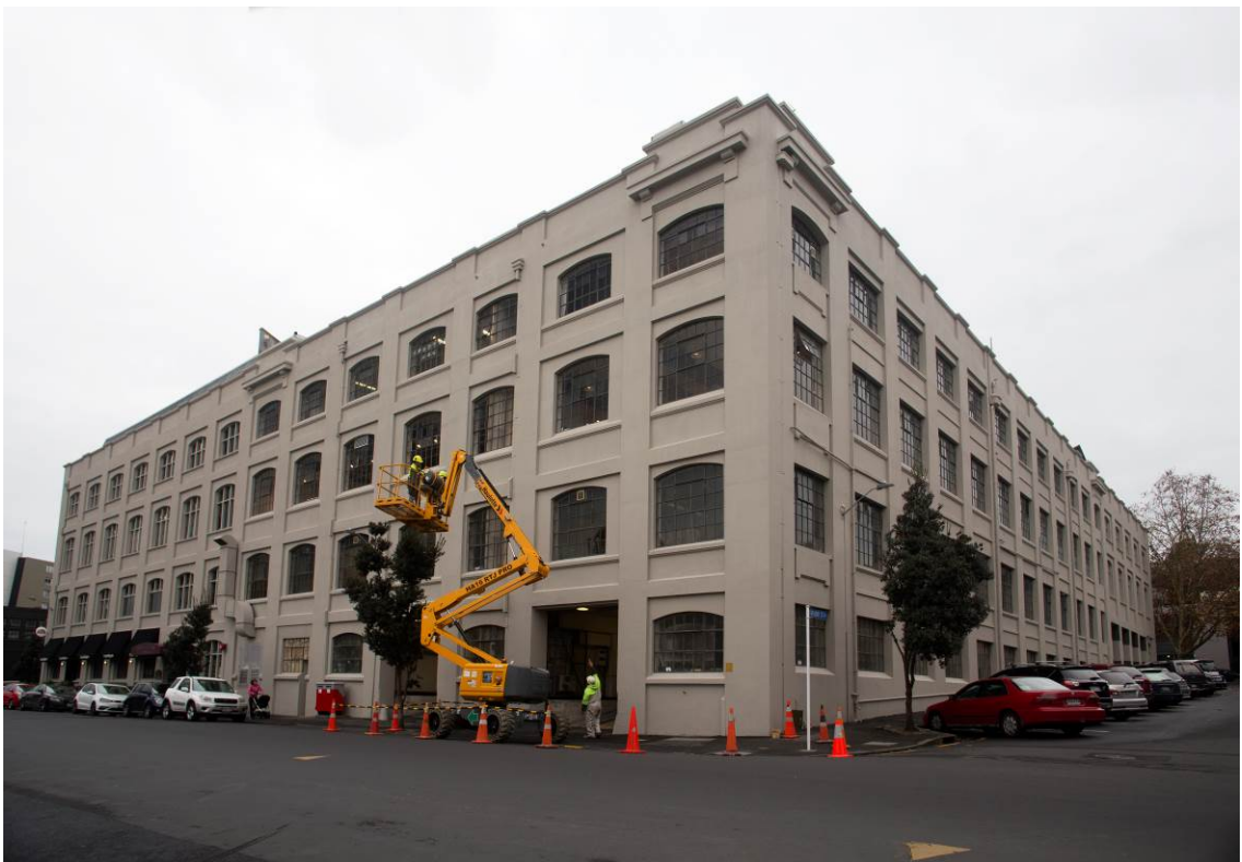
Figure 32: Southwest corner of the North Auckland Farmers' Cooperative building on the corner of St Georges Bay Road and Faraday Street
