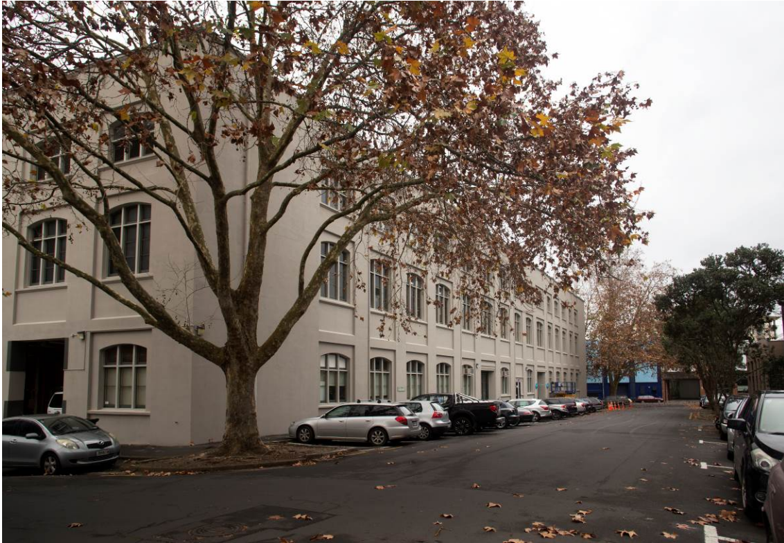
Figure 35: Eastern face of the New Zealand Shipping Company Building looking from Faraday Street up Watt Street
