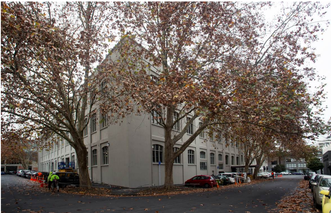
Figure 38: North-eastern corner of the New Zealand Shipping Company Building on the corner of Watt Street and Kenwyn Street
