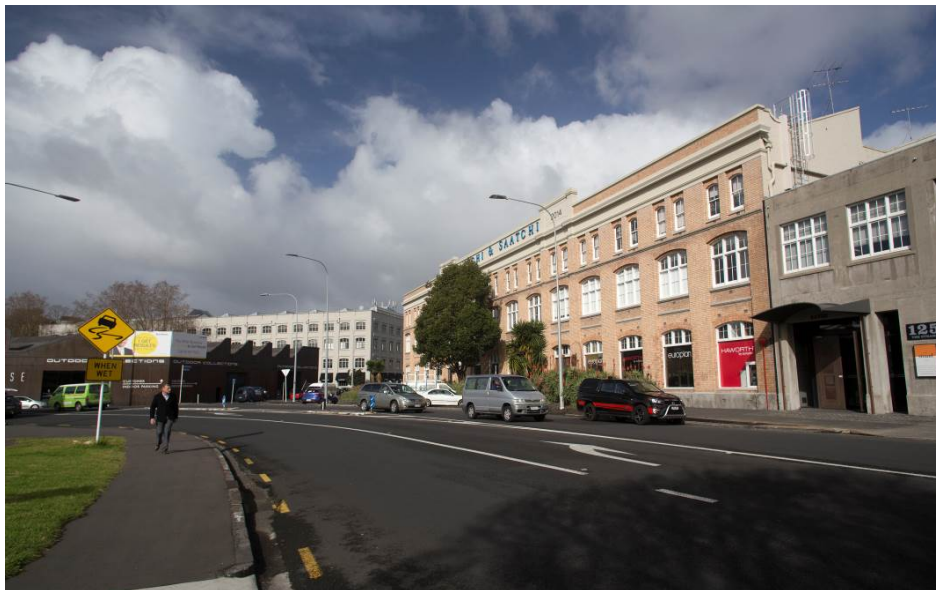
Figure 10: Shows the context of the site from The Strand. In the foreground is the former NZ Loan and Mercantile Wool Store, to the left the Design Warehouse building and in the background the NZSC, FCAC & NAFC buildings.
