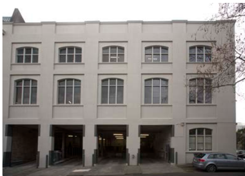
Figure 8: New Zealand Shipping Company Loading bay on Faraday Street
