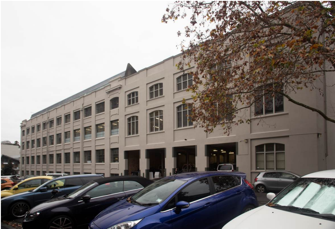
Figure 34: The North Auckland Farmers' Cooperative building on the left and the New Zealand Shipping Company building on the right on Faraday Street
