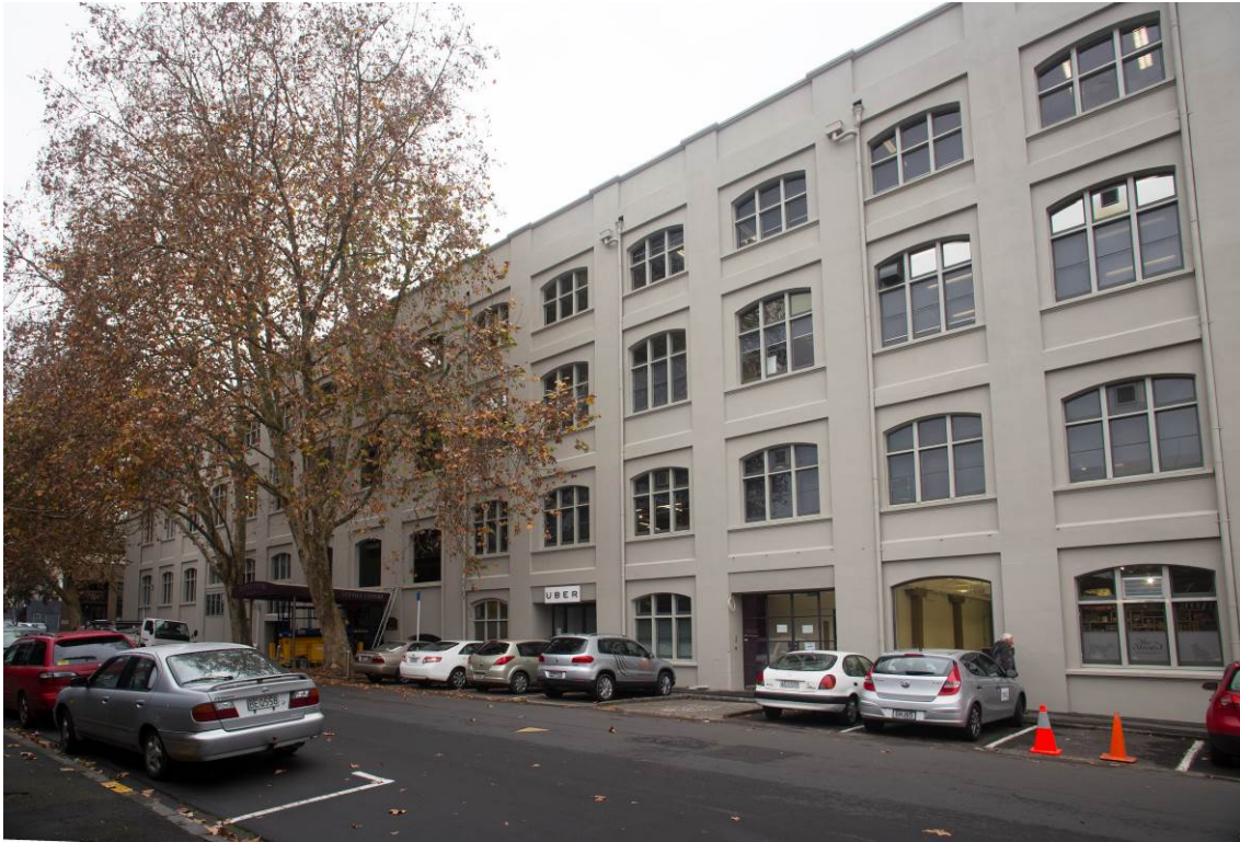
Figure 29: Northern face of the Farmers Auctioneering Company building on Kenwyn Street
