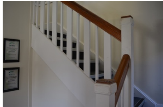
Figure 26: Timber dog-leg staircase in the original Caretaker's Flat portion of the pavilion (now used by Auckland Bowls) providing access to the first floor.
