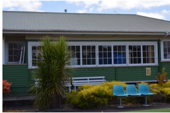
Figure 11: Windows originally inserted to the far left and right of the south elevation are combined to create a wide opening.
