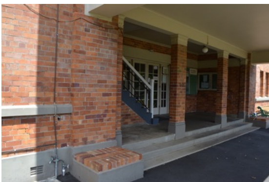
Figure 21: Ground floor porch, providing access into the original portion of the pavilion (1930). Note the staircase providing external access to the first floor, and the brick columns and pilasters.
