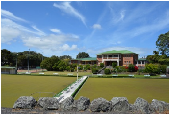
Figure 4: Looking south from the vicinity of Epsom Avenue across the bowling greens toward the Mount Eden Bowling Club Pavilion.
