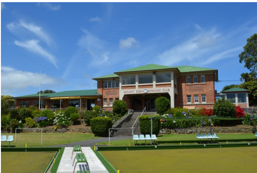
Figure 16: Northeast (front) elevation, facing the bowling greens and Epsom Road beyond.
