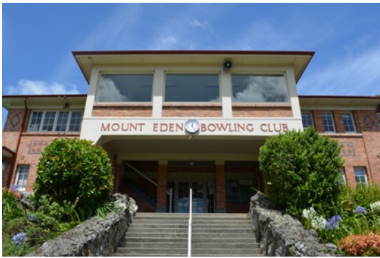
Figure 17: Front elevation of the original portion of the pavilion, showing steps up to the entry. The front bay was added in the c.1950s.
