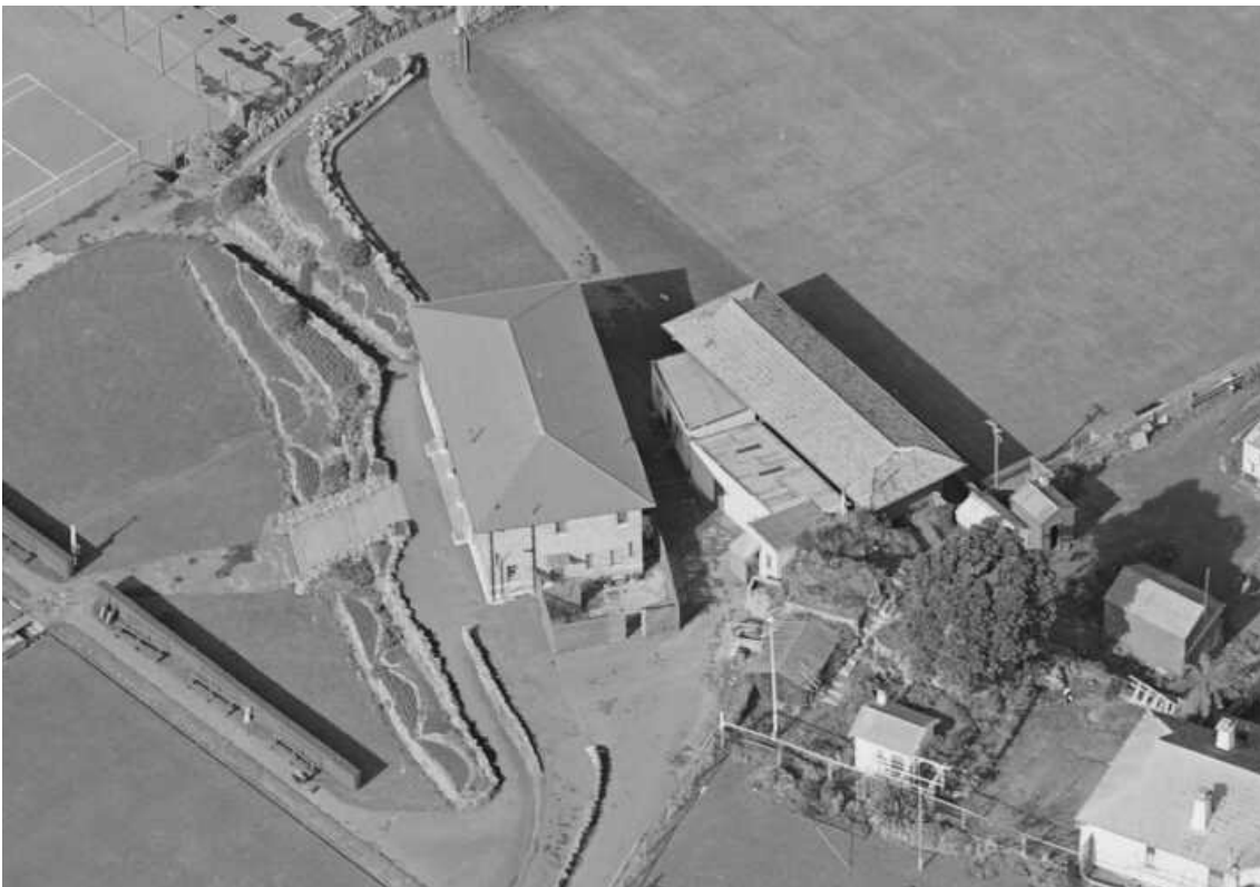
Figure 47: Aerial photograph overlooking the Mount Eden Bowling Club, and close-up of the pavilions, 28 June 1949. Note that a number of the buildings associated with the R.N.Z.A.F. occupation remain. Whites Aviation Collection, Alexander Turnbull Library, WA-20816-G
