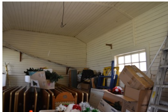
Figure 13: The interior of the central portion of the original pavilion (1925).
