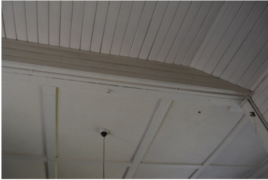
Figure 14: Showing the transition in the ceiling from timber panelling (1925 portion) to criss-cross battens (1928 addition), indicating the location of the pavilion's original end (eastern) wall.
