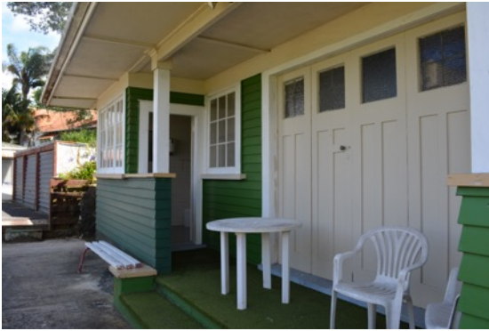
Figure 10: Recessed porch on south elevation.
