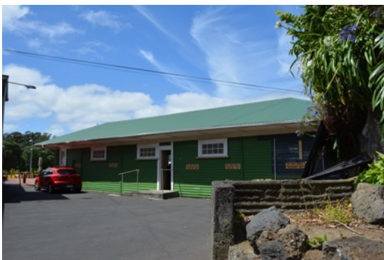
Figure 8: North (rear) elevation, which back onto the Bowling Club Pavilion.
