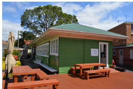
Figure 9: East and part south (front) elevations.
