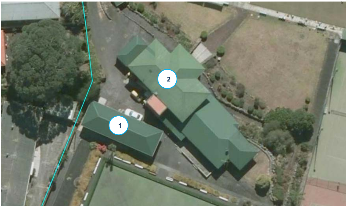
Figure 6: Close-up of the two subject buildings. The Mount Eden Croquet Club Pavilion (Former) (1) and the Bowling Club Pavilion (2) (Auckland Council GeoMaps).
