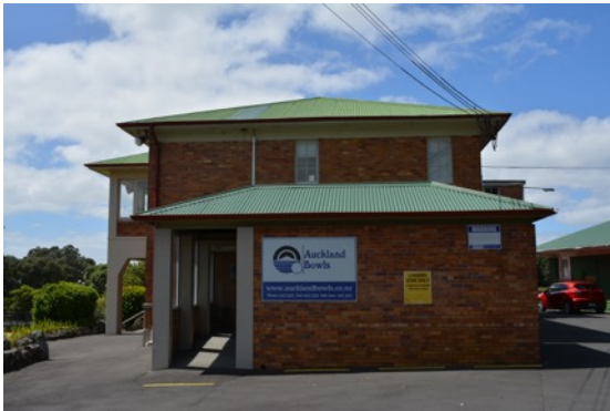
Figure 19: North-west elevation showing the carport addition.
