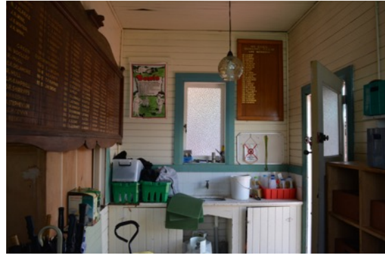
Figure 15: The kitchen with sink still in place, located in the eastern portion (1928) of the pavilion. This space was subsequently used by the Bowling Club as a locker room.
