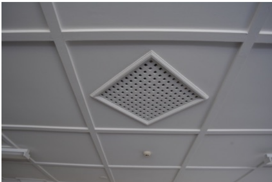
Figure 25: Timber batten ceiling with timber ventilation grille in the first floor meeting room.
