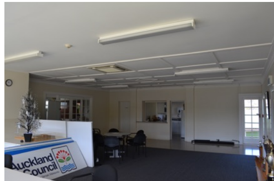
Figure 24: First floor meeting room, now used by Auckland Bowls. The change in ceiling finish marks the start of the front bay addition (c.1950s).
