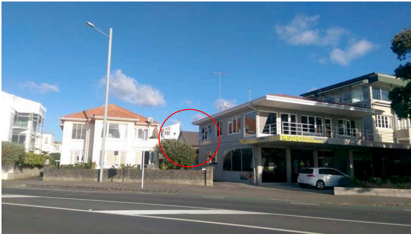
Showing the two-storey, 1950s structure built at the front of the site as a garage with accommodation overhead. It is now used as a pilates studio. The roof of the cottage is just visible (circled).
