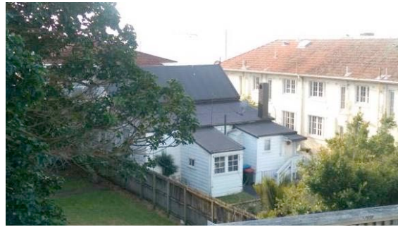
Figure 5: Rear elevation (The Heritage Studio Ltd., 2016).
