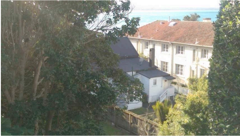
Showing the rear (south) elevation of the cottage, with multiple modest lean-tos. Note the proximity and orientation to the St Heliers beach.
