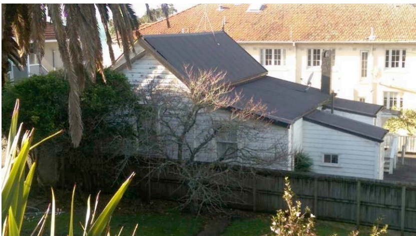
Auckland Road view of the cottage, showing the side (west) elevation. Two four-pane double-hung sash windows are visible.
