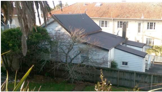
Figure 4: Side (west) elevation showing salt-box form and double-hung sash windows (The Heritage Studio Ltd., 2016).
