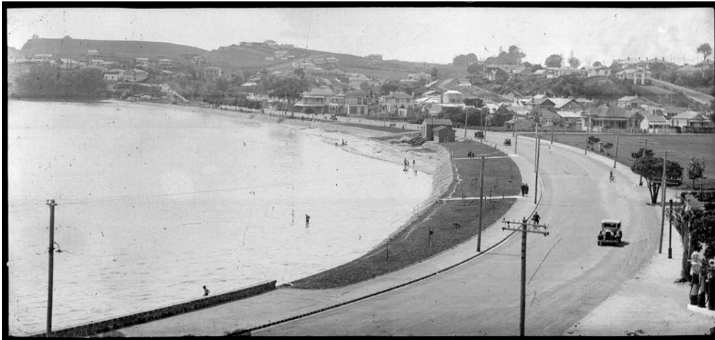
Figure 17: Looking east along the newly formed Tamaki Drive and St Heliers beach from the vicinity of Auckland Road. The seaside suburb had experienced a marked growth during the development boom of the previous decade. Note the fuel pumps of J. E. F. Laslett's garage (lower right), 1931. Sir George Grey Special Collections, Auckland Libraries, 4-5363
