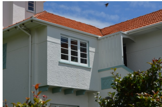
Figure 9: First floor porch with turned ballusters, decorative frieze and a partially cantilevered first floor.
