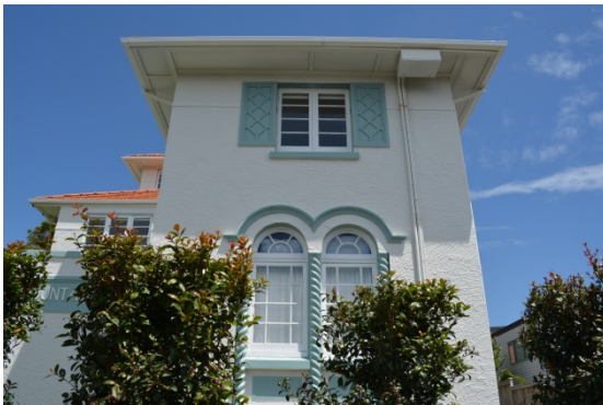
Figure 8: The double-arched window with hood-mould and barley twist columns – a notable feature of the building, and casement with shutters.
