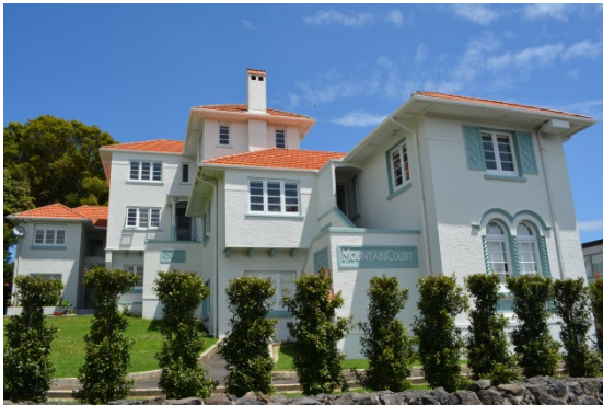
Figure 6: North (front) and partial east (side) elevations, showing how the prominent "stepping" of the building's rooflines.
