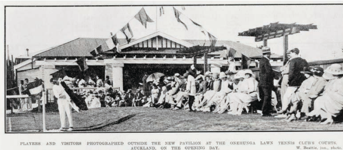
Figure 18: Onehunga Lawn Tennis Club's pavilion (1922), designed by Garrett.
