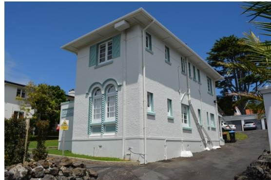
Figure 7: Note the dominance of the wall massing against the small windows on the west (side) elevation, typical of Spanish Mission architecture.
