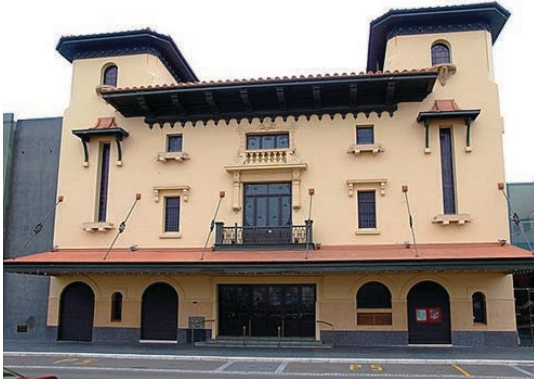
Figure 29: Hastings Municipal Theatre (Former). (CC Licence 3.0. Image courtesy of commons.wikimedia.org. Copyright: Ulrich Lange - Wikimedia Commons. Taken By: Ulrich Lange. Date: 10/03/2010).
