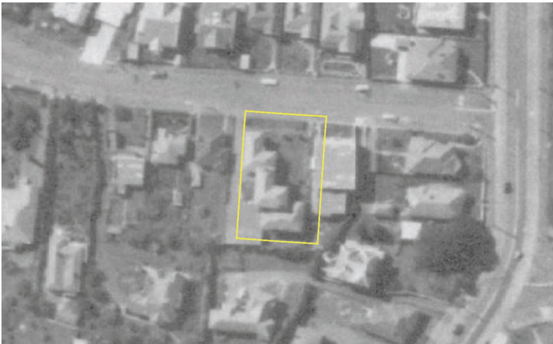
Figure 17: 1959 historic aerial showing Mountain Court, 4 View Road with its 'L'-plan rear addition (Auckland Council GeoMaps).
