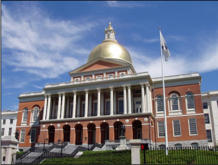
Figure 20: The Massachusetts State House in Boston demonstrating the arcade at ground level, similar to the arcade at the basement level on the northern side of the former St Patrick's School. ( www.commomns.wikimedia.org accessed 5 July 2016)
