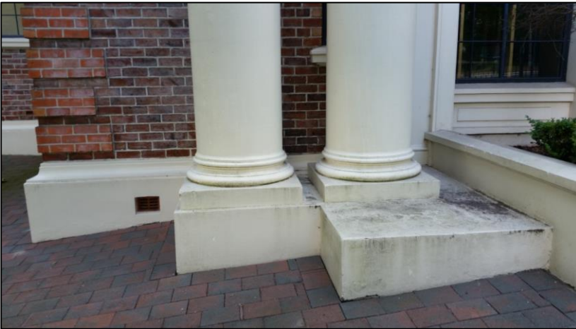
Detail of column base at former front entry
