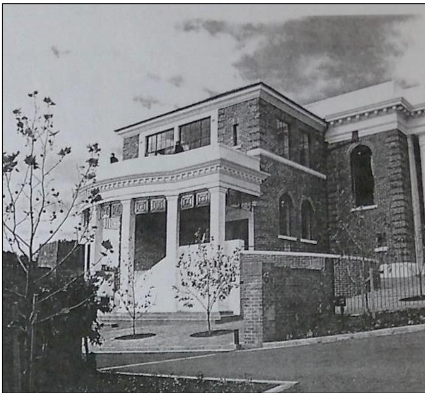
Figure 9: The new portico entry on the western side of the building which also provided an upper floor terrace. The new doors can be seen leading on to the terrace. The new entrance was accessed from the existing ramp on the southern side and steps on the northern side. (Architecture NZ, May/June 1992).
