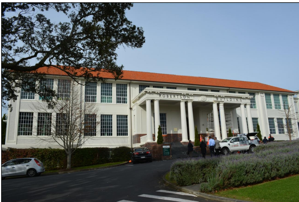
Figure 33: The Robertson Building at St Cuthbert's College. (Auckland Council July 2016).
