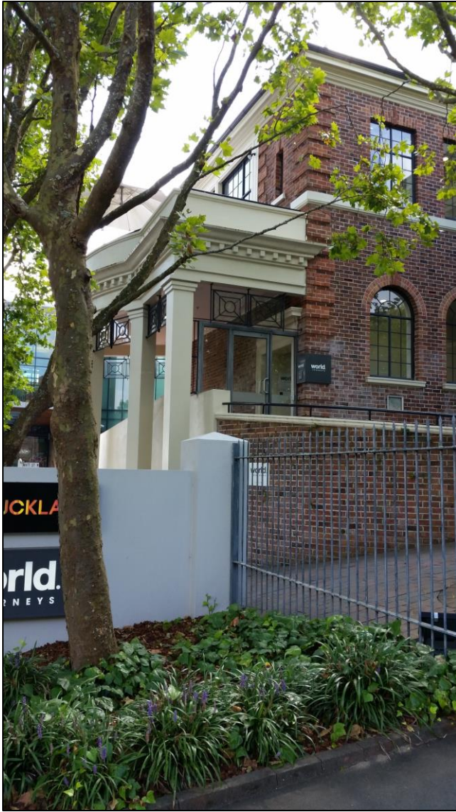
South western corner of building indicating new extension with new entrance
