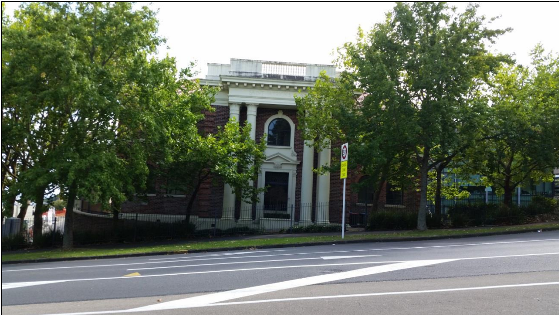
Wellington Street façade
