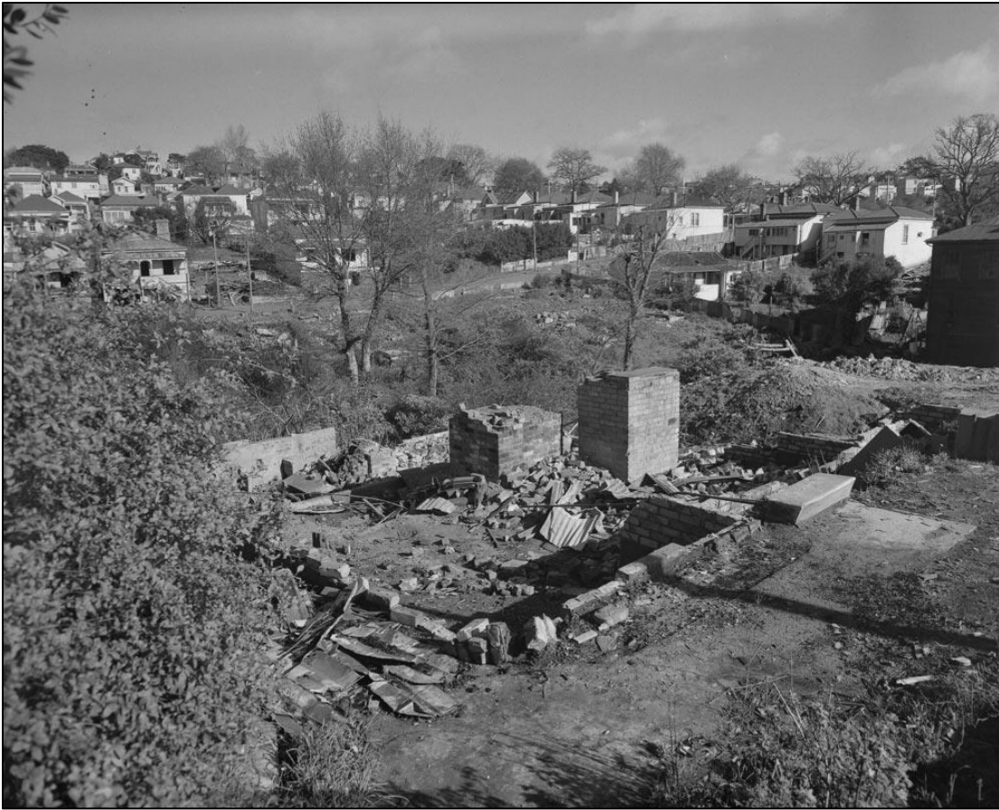
Figure 37: Demolition site looking southwest from Wellington Street to Hepburn Street in 1957-58. The area to the far left was soon to be demolished to provide room for what is now known as Freemans Park with the construction of the Star Flats. (Sir George Grey Special Collections, Auckland Libraries, 580-2216).
