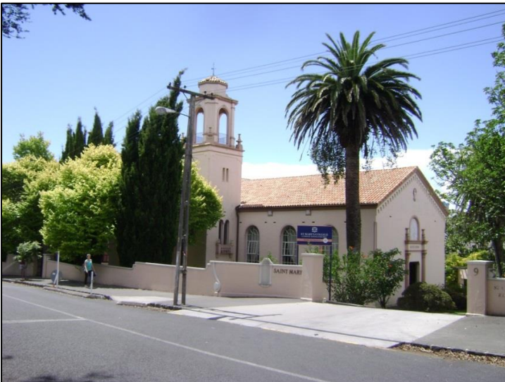
Figure 32: St Mary's College as seen from New Street. (Auckland Council February 2012).
