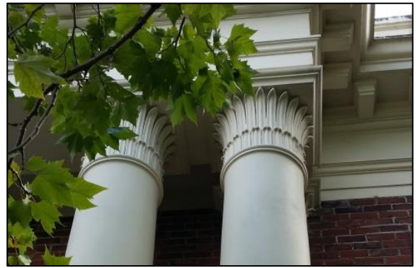
Detail of column decoration
