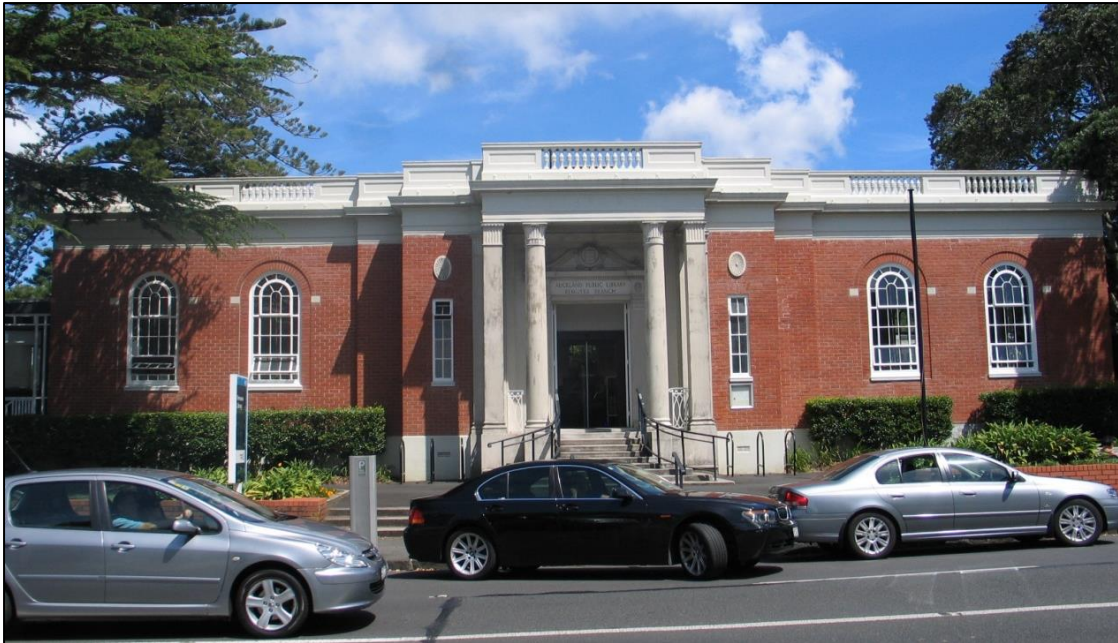
Figure 27: The Remuera Public Library designed by Gummer and Ford and constructed around the same time as St Patrick's Cathedral School. (Auckland Council, May 2015).
