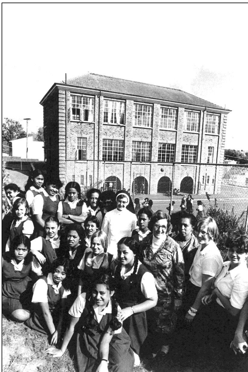
Figure 8: The students and teachers in 1979 at the rear of the school. At this stage the building was very much the same as when it was first constructed. (Auckland Catholic Diocesan Archives).
