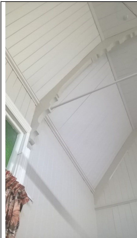
Figure 65. Timber support brackets with decorative detailing. Timber match stick ceiling.
