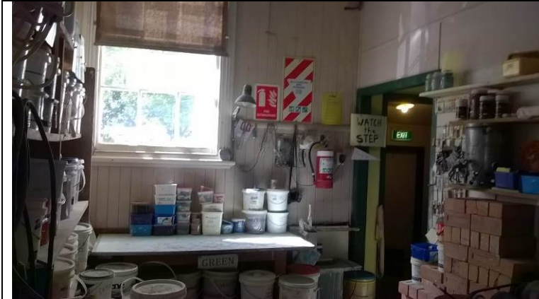
Figure 59. Interior of Potters Club premises. Match stick wall lining, with paint finish.
