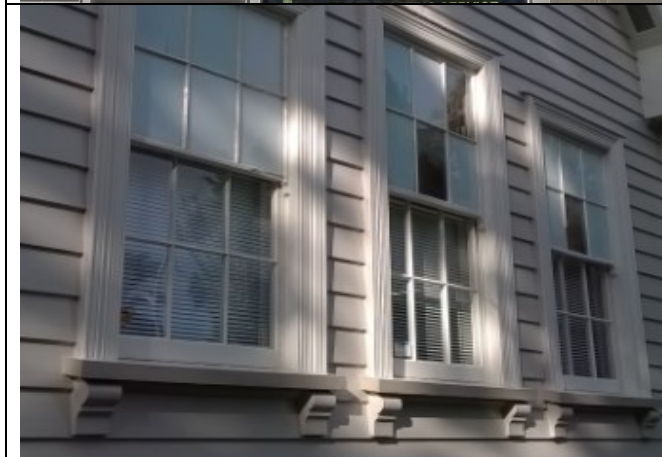
Figure 50. Details of windows, with 12 panes. Note the bracketing beneath the sills.
