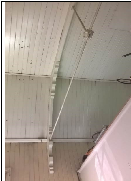
Figure 63. Timber support brackets with decorative detailing. Timber match stick ceiling.
