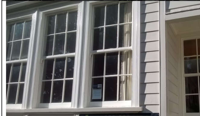
Figure 49. Examples of double hung timber windows in a row on the front elevation (central axis).
