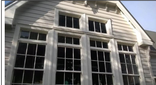
Figure 48. The front elevation of the building generally contains timber framed, double hung windows in sets. This is often a distinctive feature applied to education facilities in the early twentieth century.
