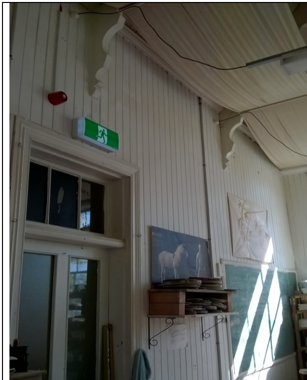
Figure 69. Vertical timber walls in the potters workshop.
