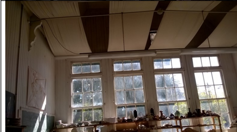
Figure 60. Windows as seen from the interior of the Potters Club premises. Cloth has been hung from the ceiling to create a feeling of a semi-lowered ceiling. The condition of the ceiling paintwork is peeling in areas.
