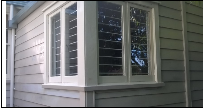
Figure 51. Later timber framed casement windows on the rear addition to the building.
