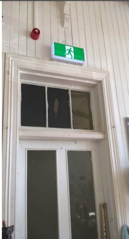
Figure 78. Fanlights above door as part of door framing (in potters workshop)
