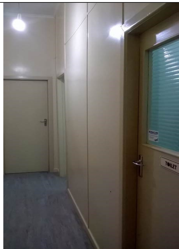
Figure 72. Hardi plank walls, linoleum floor surface and hollow core doors at rear area of building.
