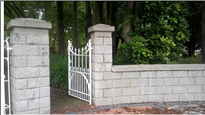
Figure 82. Brick/stone and wrought iron gates leading into the site, on the corner of Wood Street and Great South Road.
