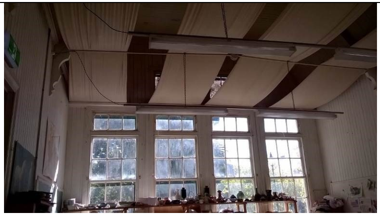
Figure 66. Cloth forms a partial false ceiling in the potters workshop (easily removable and of little intrusion to historic ceiling and wall fabric).
