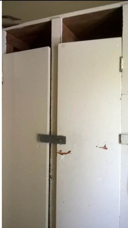
Figure 81. Lockers, possibly from later years of the school. May be of some wider interest in relation to the former use of the place (cupboards on bottom left are clearly later, but likely still from when the building was a school and therefore are of some general interest).
