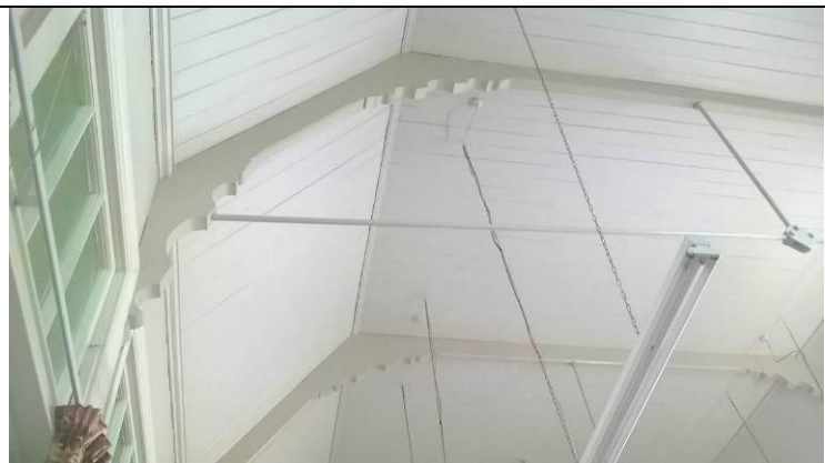
Figure 64. Timber support brackets with decorative detailing. Timber match stick ceiling.
