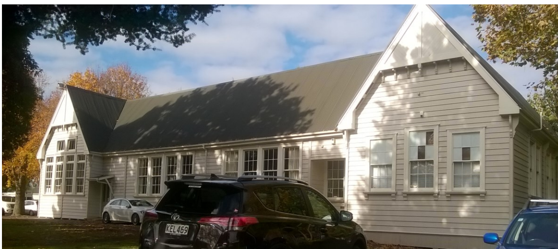
Figure 1a. View of front elevation of building as seen from edge of site on Wood Street. AC, June 2017.
