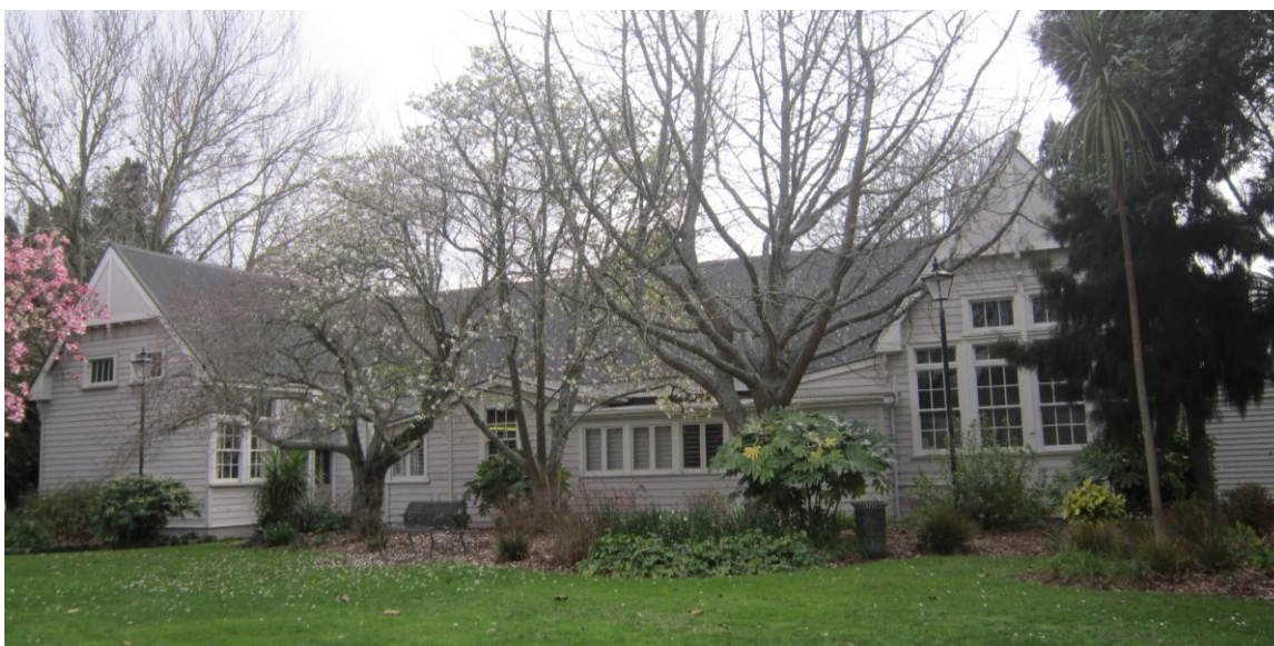
Figure 1b. Rear elevation of building as seen from green open space within Central Park. AC, August 2015 (pre-1944 field survey).
