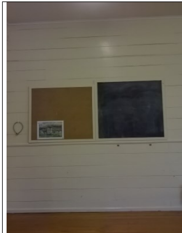
Figure 67. Vertical timber wall lining in central hall. This is where elements of the oldest fabric may be as it is the core of the original building.
