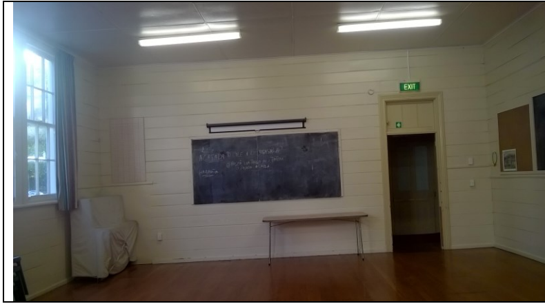
Figure 62. Blackboard in the former classroom that remains (now central hall room). Walls are horizontal timber boards.
