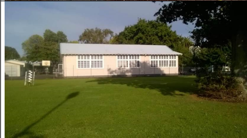
Figure 84. Side elevation of the former Infant Block, located on the adjoining site as the school (59R Wood Street). The 1924 Infant Block is one of the few other buildings remaining from the occupation of the site by the school (other than the main school building).
