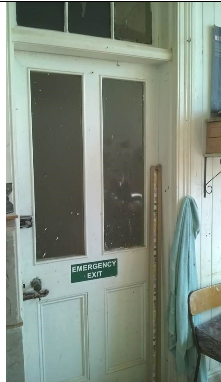
Figure 77. Glazing and panel solid timber door and associated hardware (in potters workshop)
