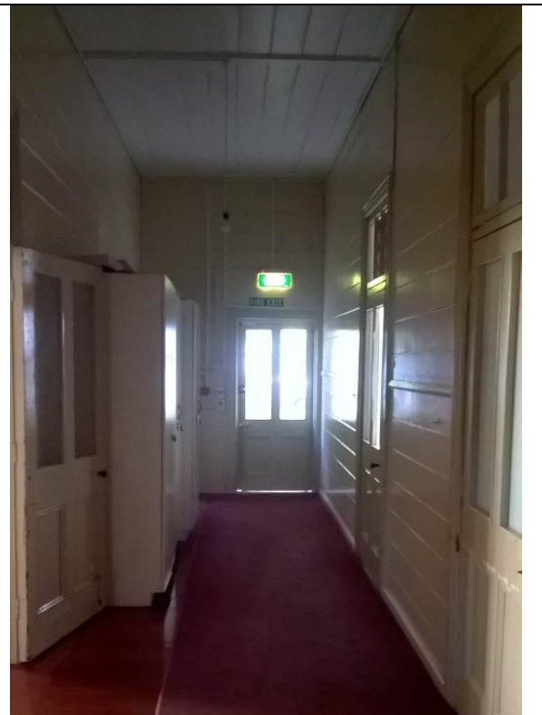
Figure 70. One of two front entrances with horizontal timber walls.
