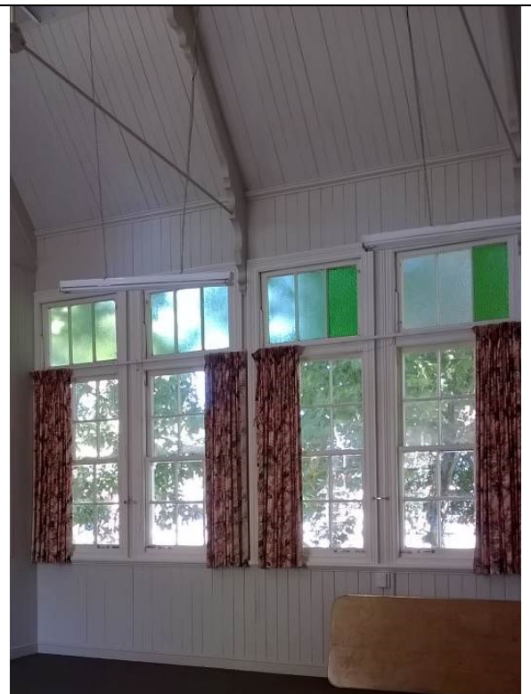
Figure 68. Vertical match stick/tongue and groove timber walls, with paint finish.
