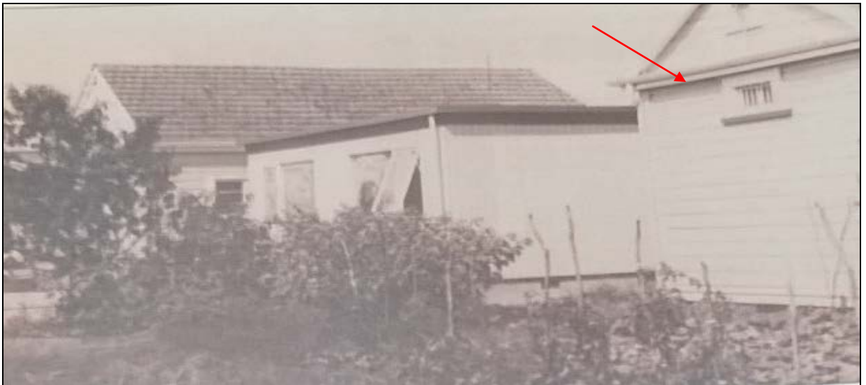
Figure 35. The extensions are shown with the Lock-up on the right and the garden of the residence in the foreground. Brewer, K. p 38.
