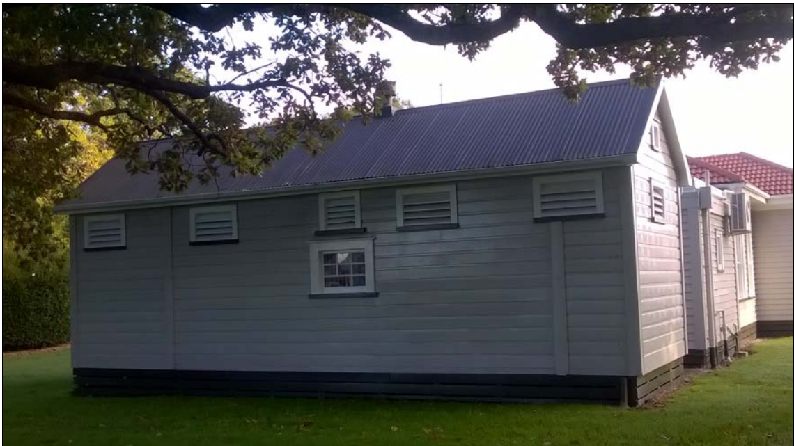
Figure 63. Side profile of the lock-up. Note the ventilation shutters.
