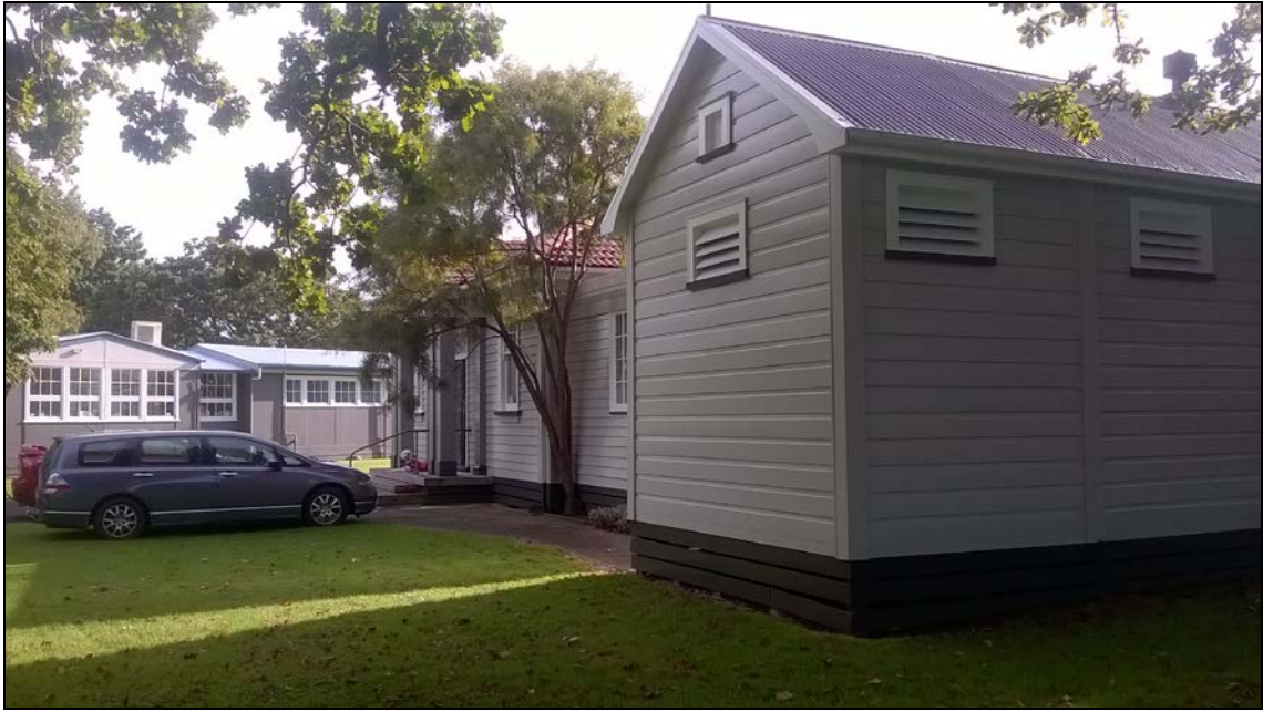
Figure 62. Side elevation of Lock up, with front entrance to Courthouse also in view.
