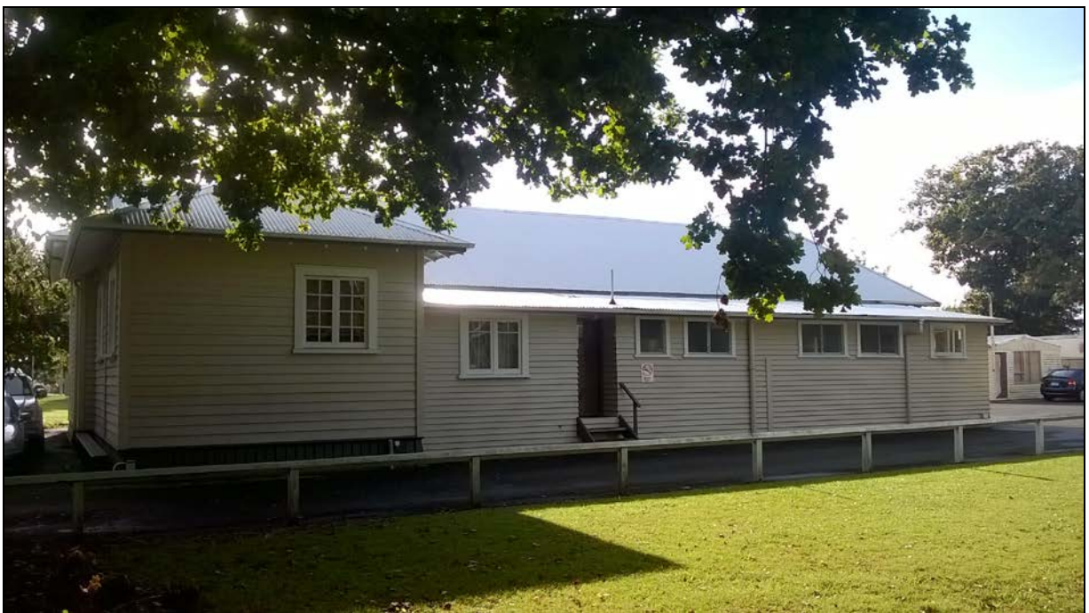
Figure 71. Side elevation of former Central School Infant Block. Now owned by the Ministry of Education.
