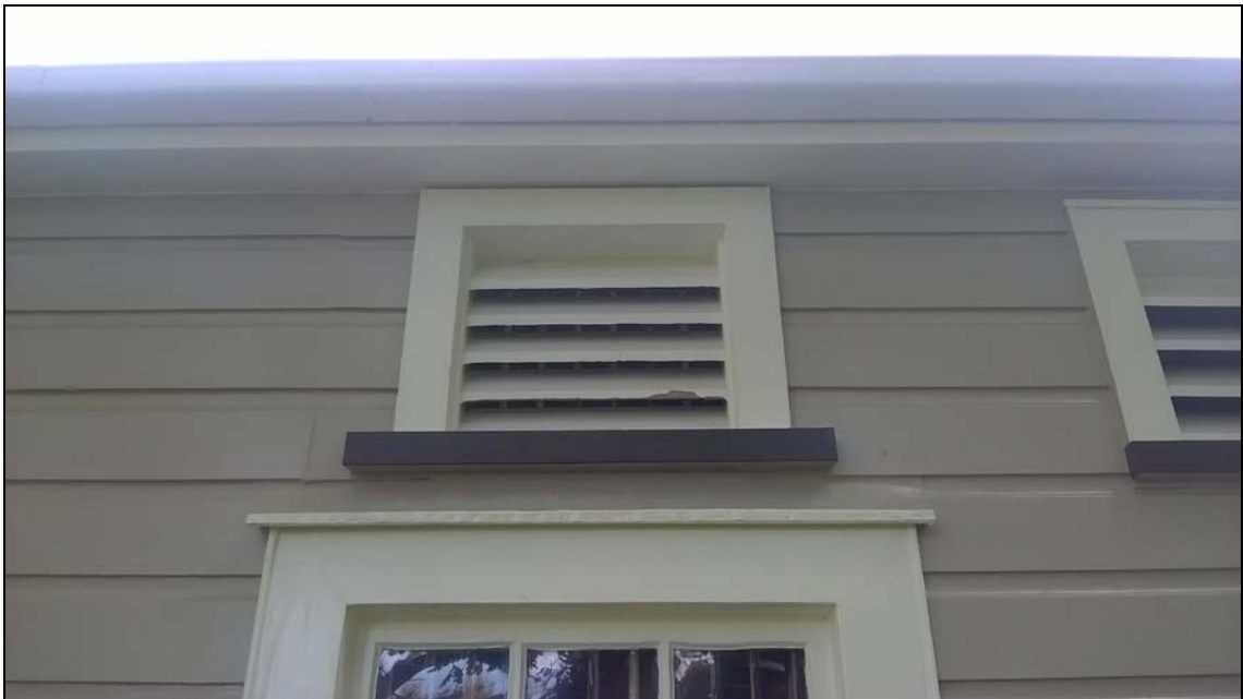
Figure 65. Example of one of the vents on the upper side elevation of the Lock-up building.
