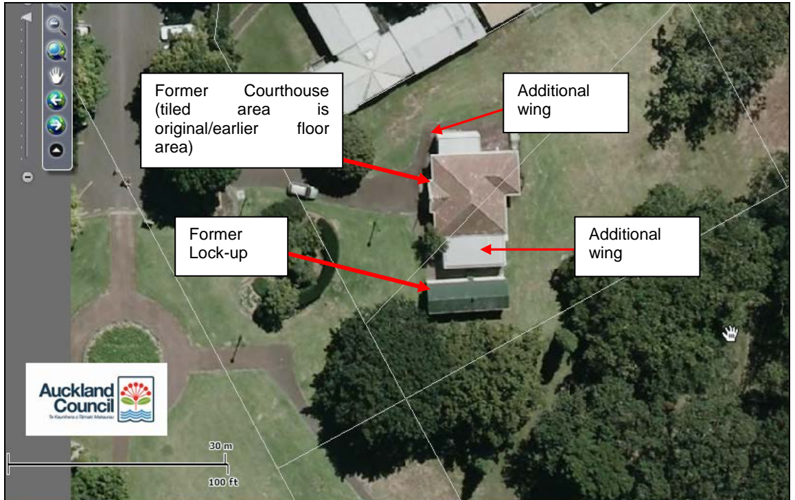
Figure 3. Aerial of former Papakura Courthouse and Lock-up. The brown teracotta roof is the outline of the original building footprint, and the grey areas are later side wings. AC GIS, aerial 2011.
