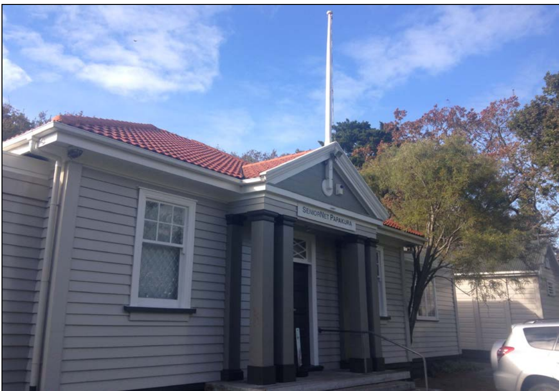
Figure 49. Front elevation of the former courthouse – side on. May 2017.
