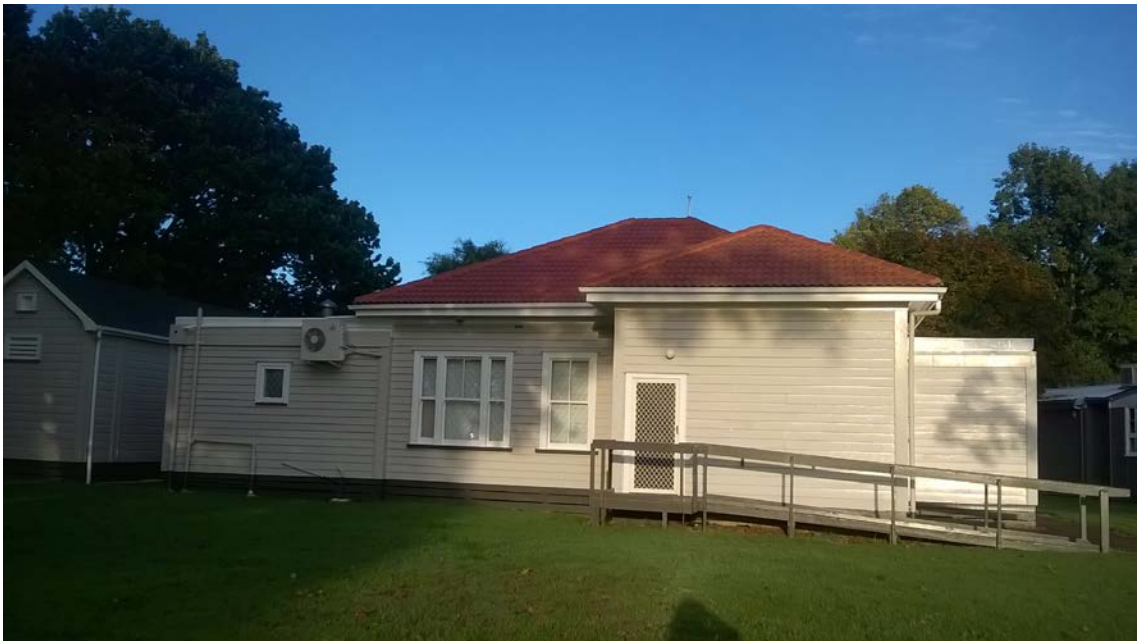
Figure 53. Rear elevation of former Courthouse.
