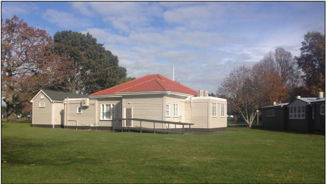
Figure 51. Rear and northern rear elevation of the courthouse. Additional wings are clearly disenable from this perspective; lock-up also in the frame. May 2017.
