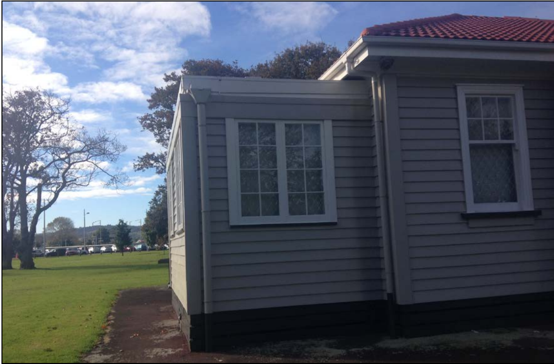
Figure 50: Front of Northern side wing. May 2017.
