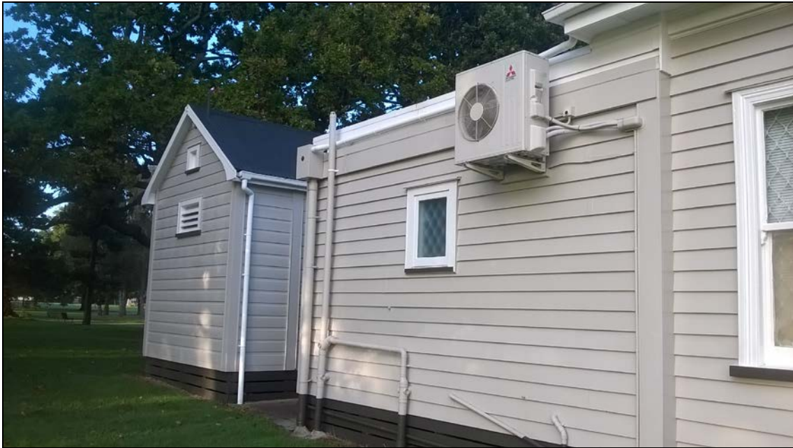
Figure 60.Lock-up in the context of the Courthouse very close by.
