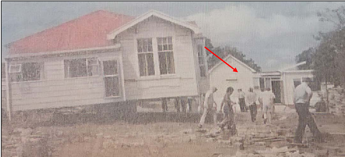
Figure 38. Relocation and removal of the police complex buildings in 1987. (The Lock-up is indicated with an arrow). Brewer, K. p 64. – Book cites the image is courtesy of Patsey Flavell.
