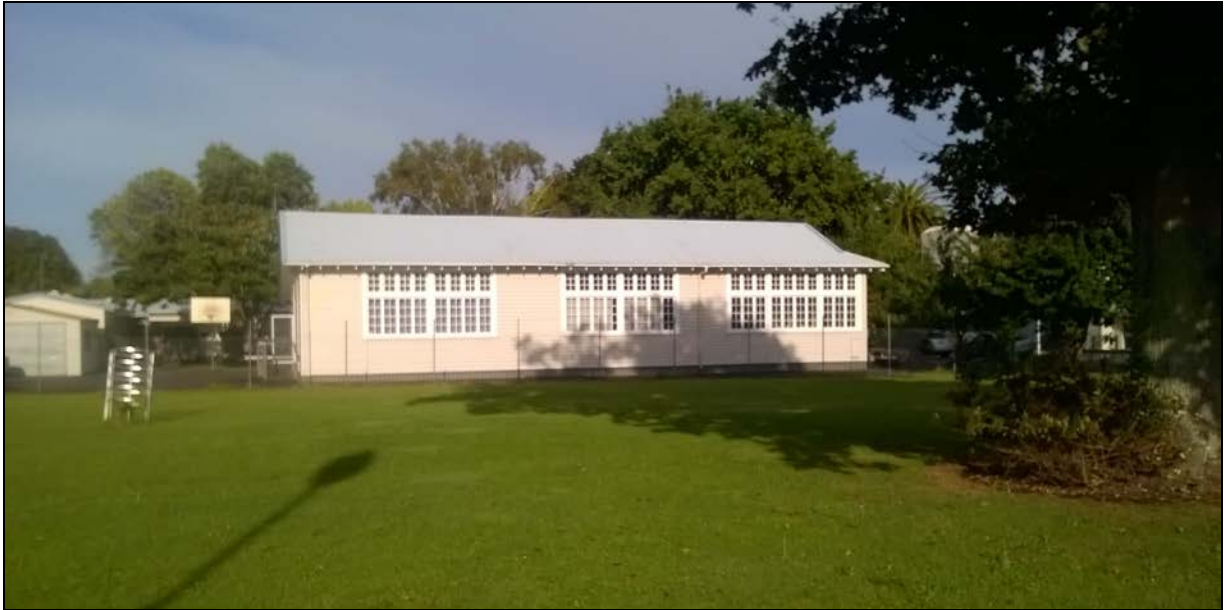
Figure 70. Side elevation of former Central School Infant Block. Now owned by the Ministry of Education.
