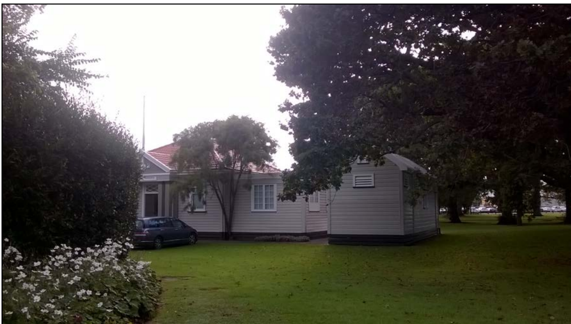
Figure 61.Lock-up in the context of the former courthouse very close by.
