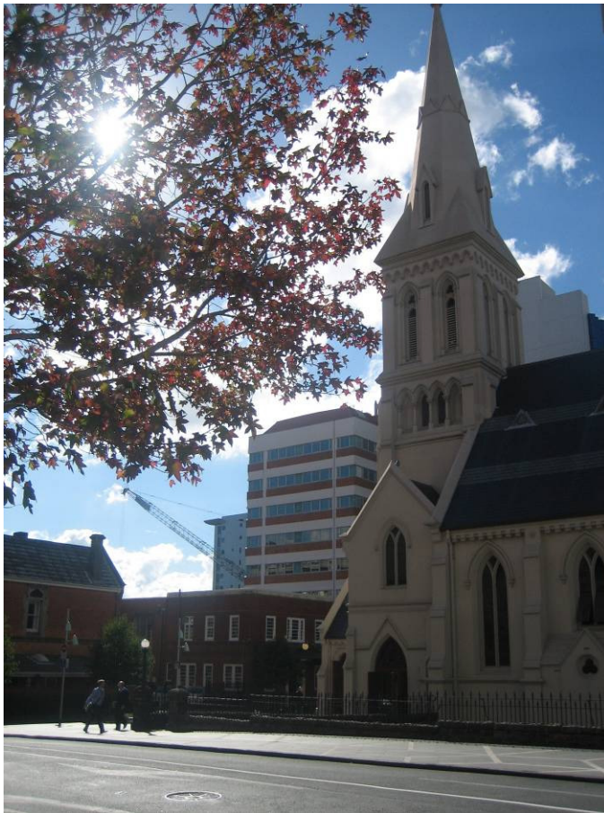
View towards 1938 portion, in context of St Patricks Cathedral.
