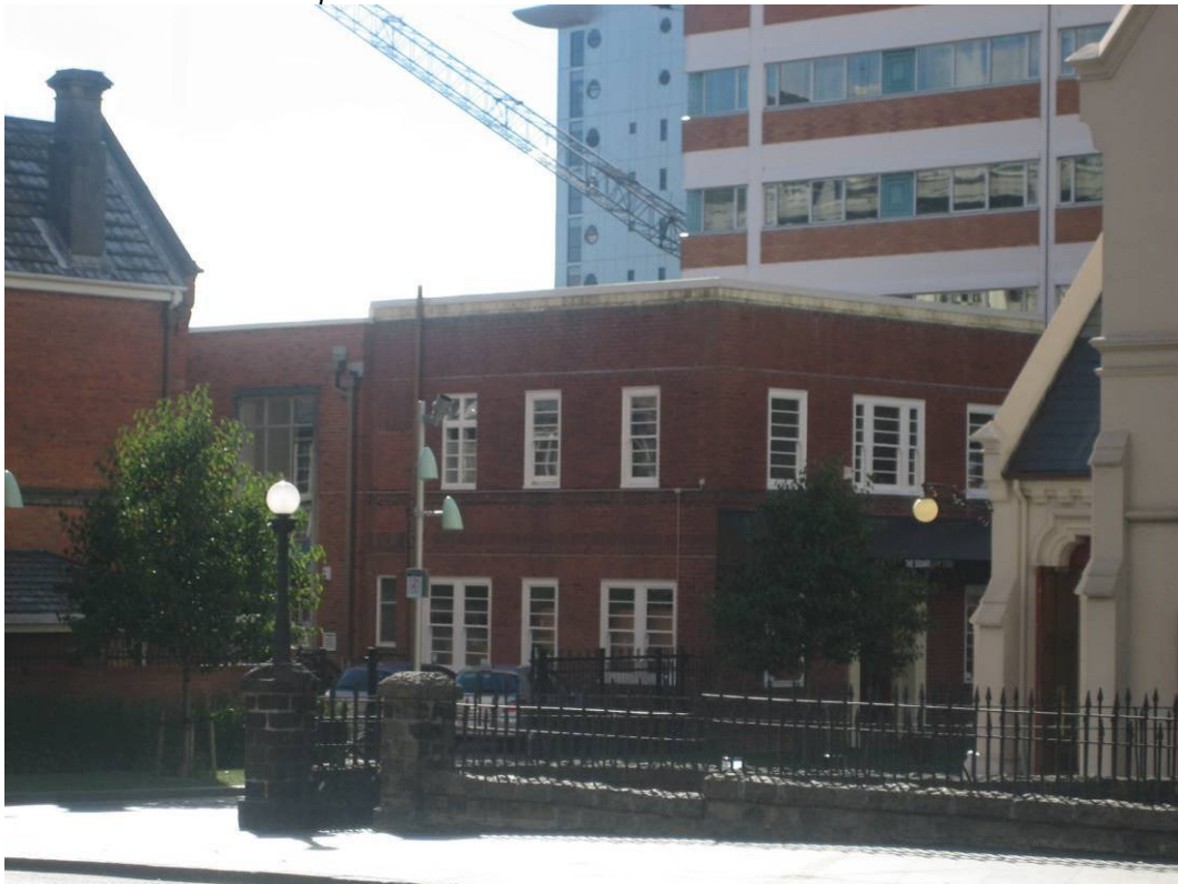
View towards 1938 portion from Wyndham Street
