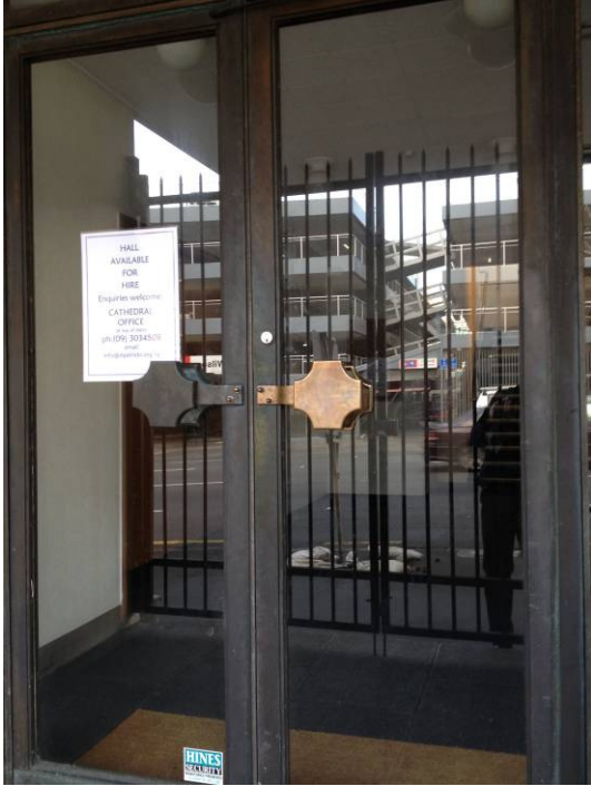
Entrance doors, Hobson Street
