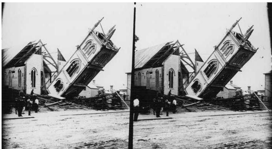
Re-erecting the tower on old St David's Church, Khyber Pass, shortly after its removal from Symonds Street, 27 September 1902, Image: Sir George Grey Special Collections, Auckland Libraries, NZG-19020927-808-1
