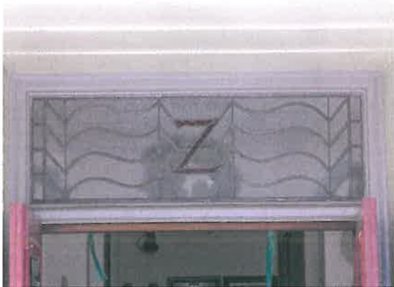
Fanlight above doorway
