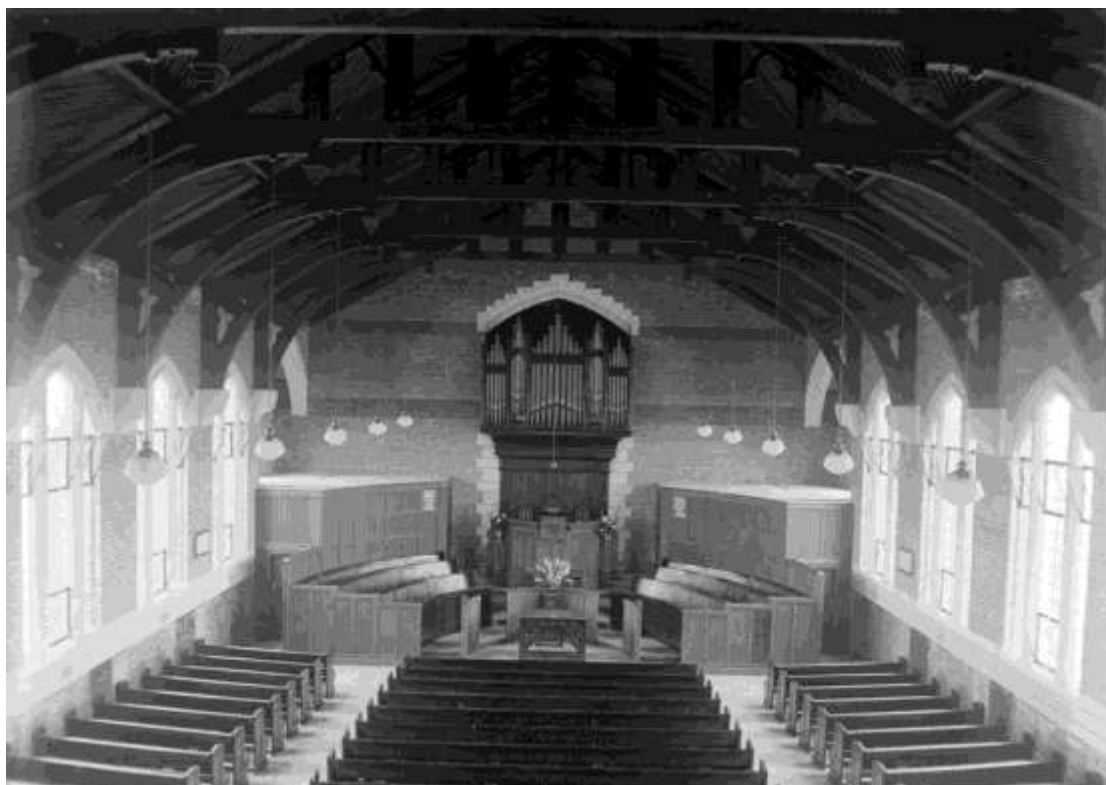
Interior view of St David's Church in Khyber Pass Road, 1927, Image: Sir George Grey Special Collections, Auckland Libraries
