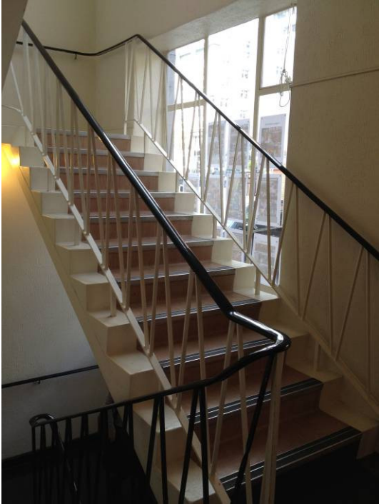
South west stairwell
