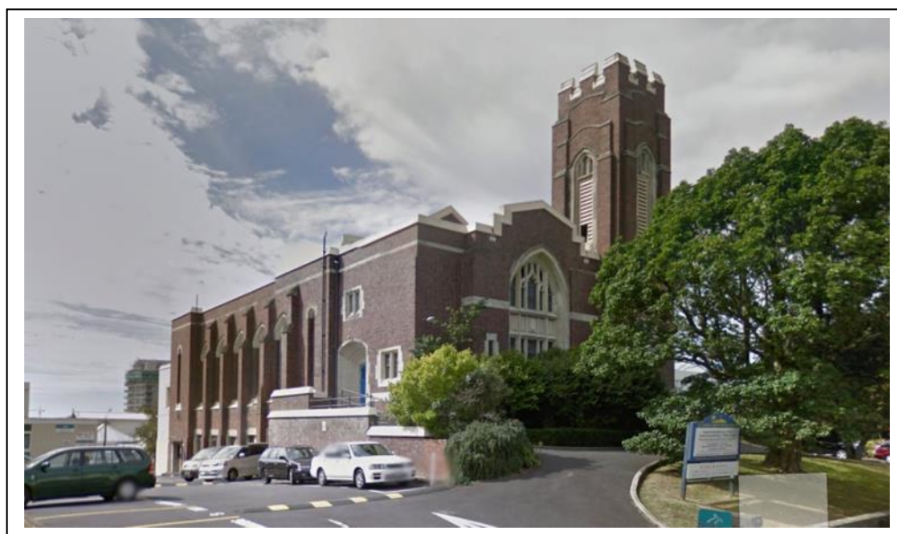
St David's Church (Presbyterian), viewed from west April 2014 (Google Earth Street View).
