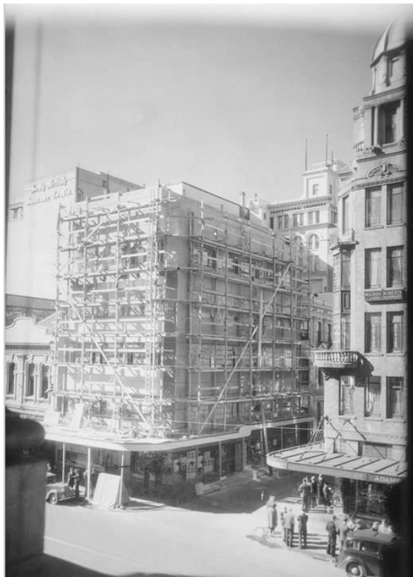
Arthur Eady Building (Former): Under construction, looking northeast, 1939. (Sir George Grey Special Collections, Auckland Libraries, 34-T7B, Clifton Firth).
