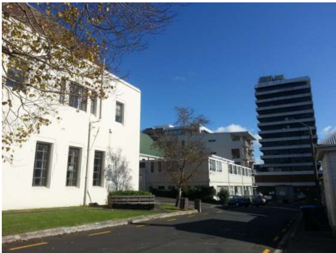
Showing the rear of the site, Image: B&T Architects 2015
