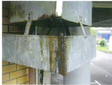
Figure 4 - Grease oozing out of a ducting outlet.
