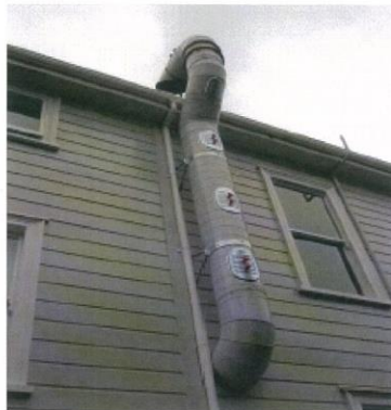
Figure 5 - Exhaust ducting from kitchen with service hatches.
