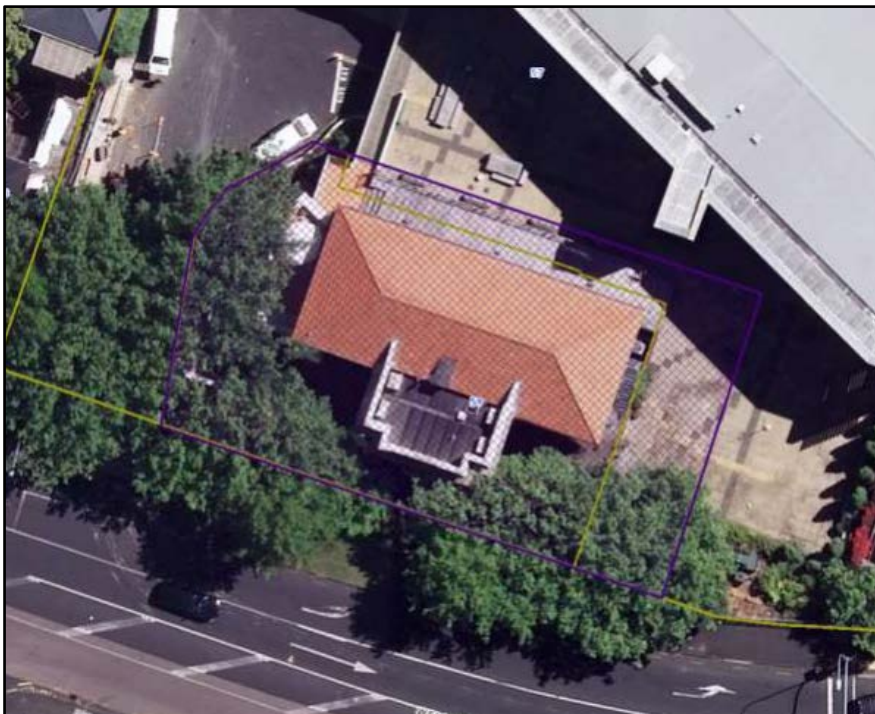
Figure 1: Proposed extent of place for 59 Wellington Street (represented by purple hatching). Extent of property boundaries around the building is represented by the yellow line.
