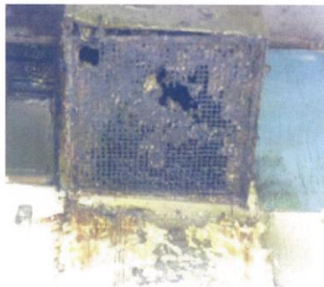
Figure 6 - Grease build up in filter exhaust.
