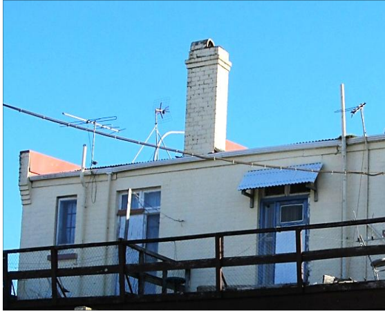
Building has chimney height 1.2m approx.
