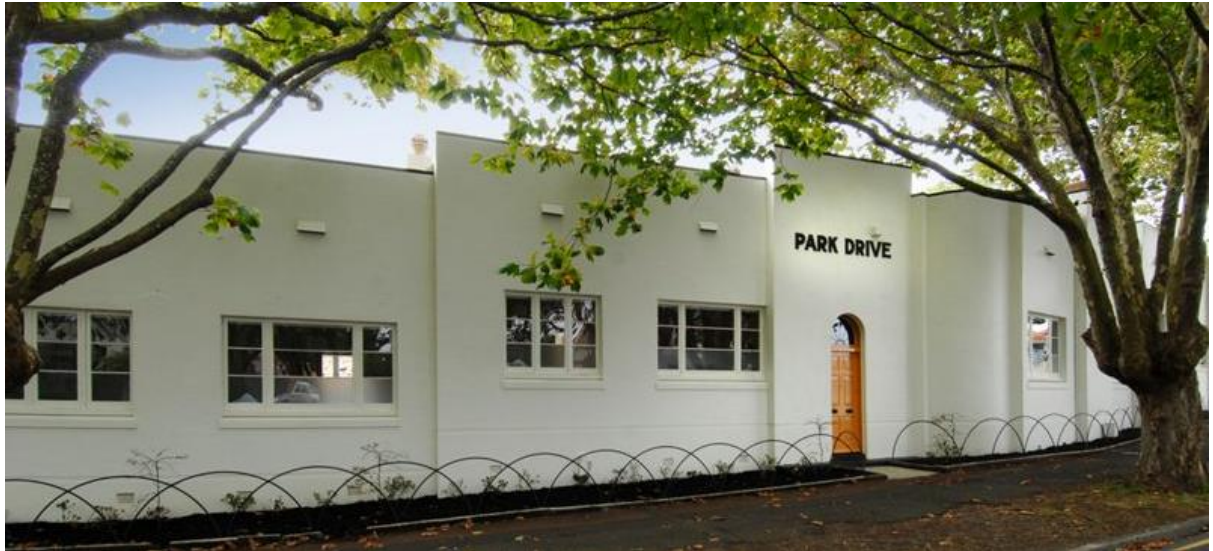
Above is a Block of Art Deco Flats on the corner of Domain Drive and Parnell road with both horizontal and vertical stepping
