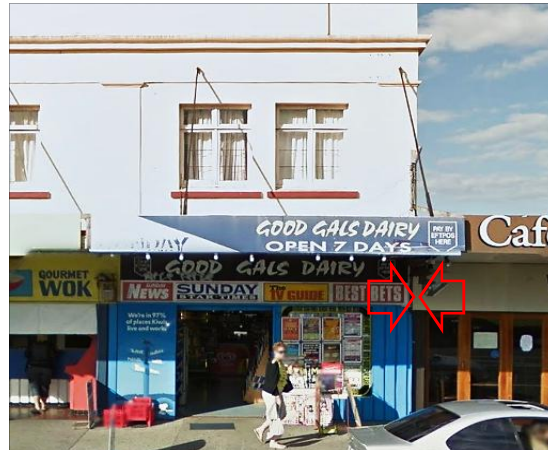
No seismic gap at transverse direction
