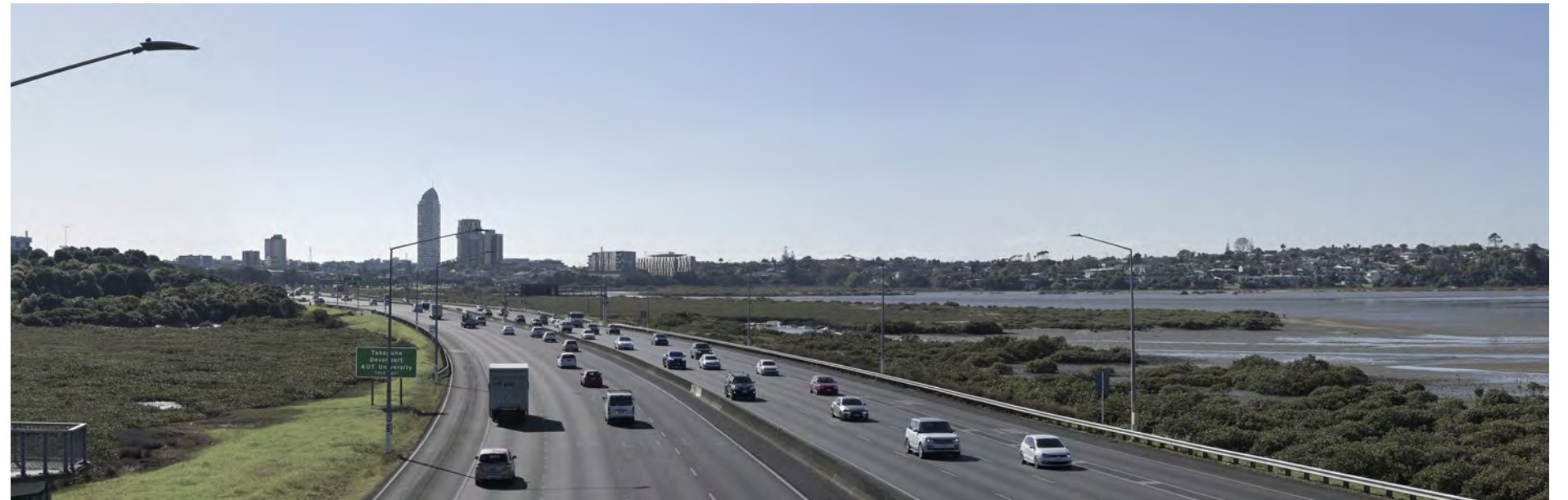
Buildings already received Resource Consent
