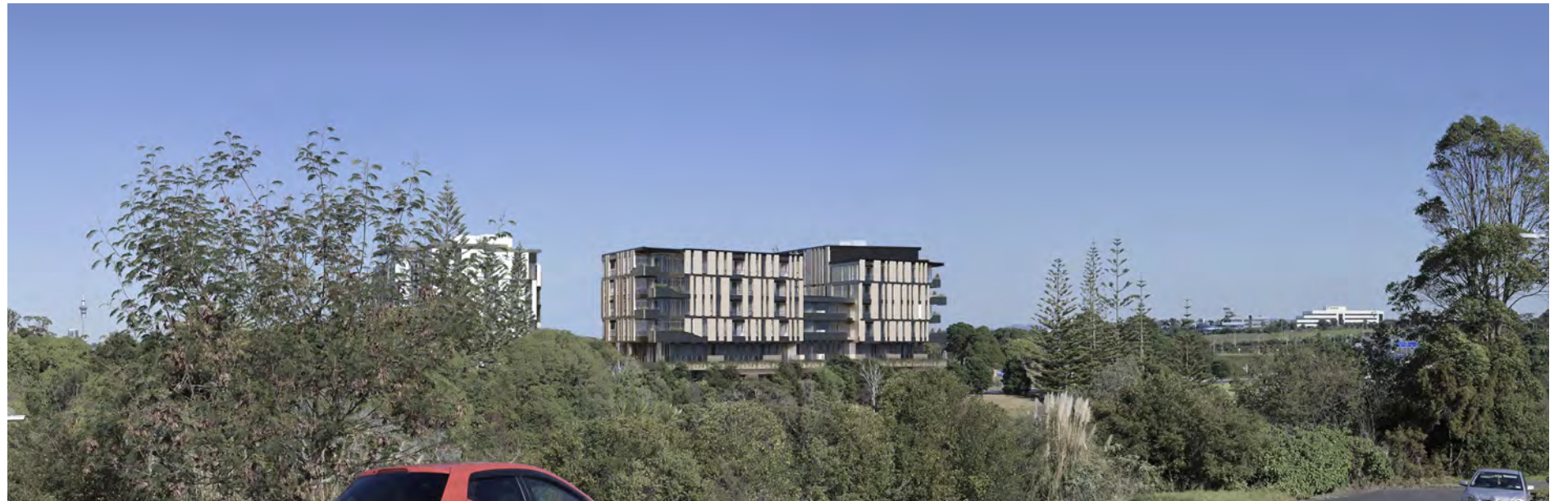
Buildings already received Resource Consent
