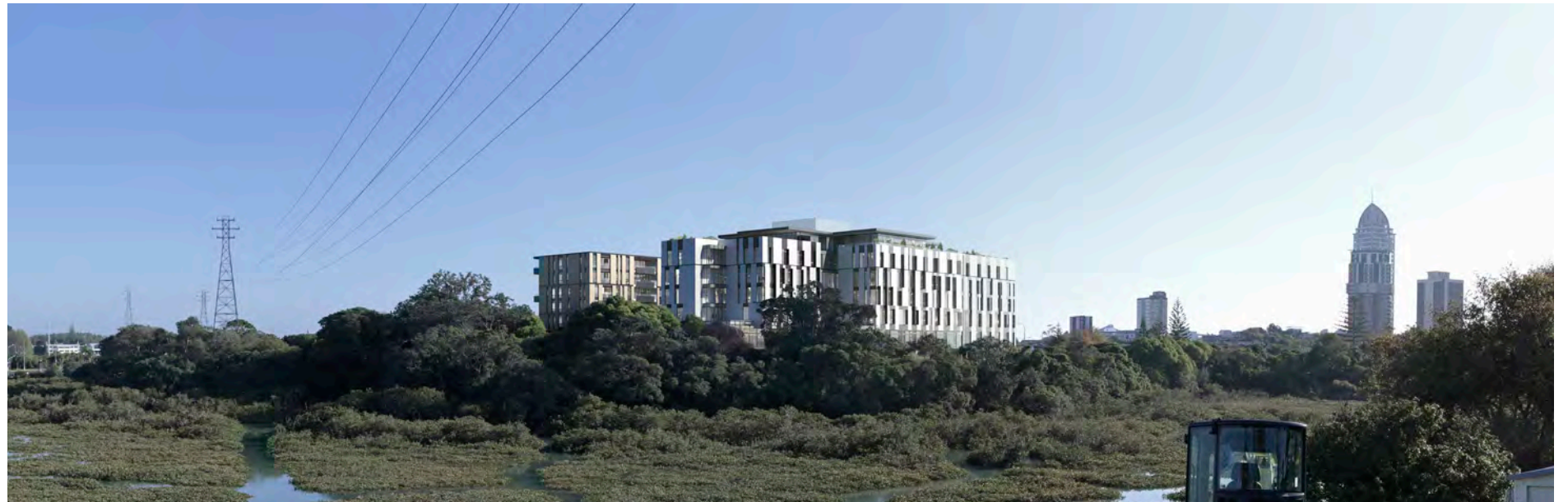
Buildings already received Resource Consent
