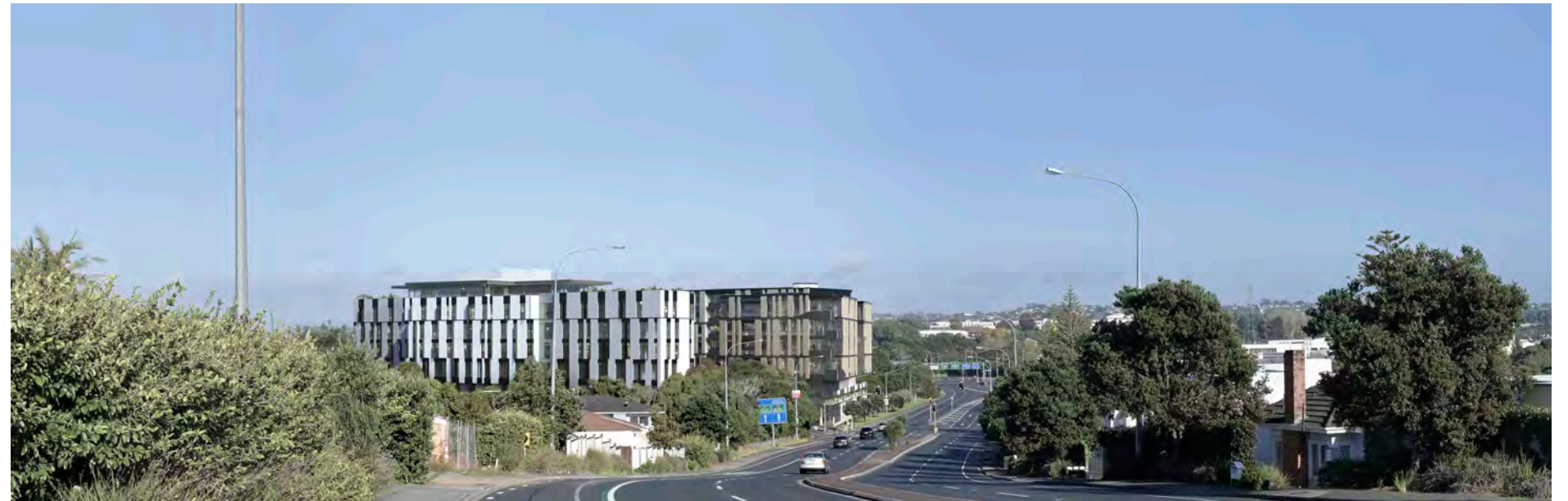
Buildings already received Resource Consent
