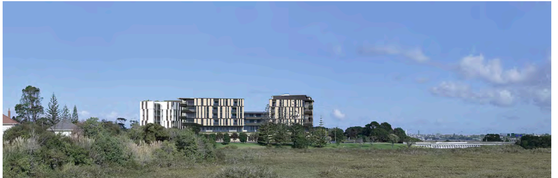
Buildings already received Resource Consent
