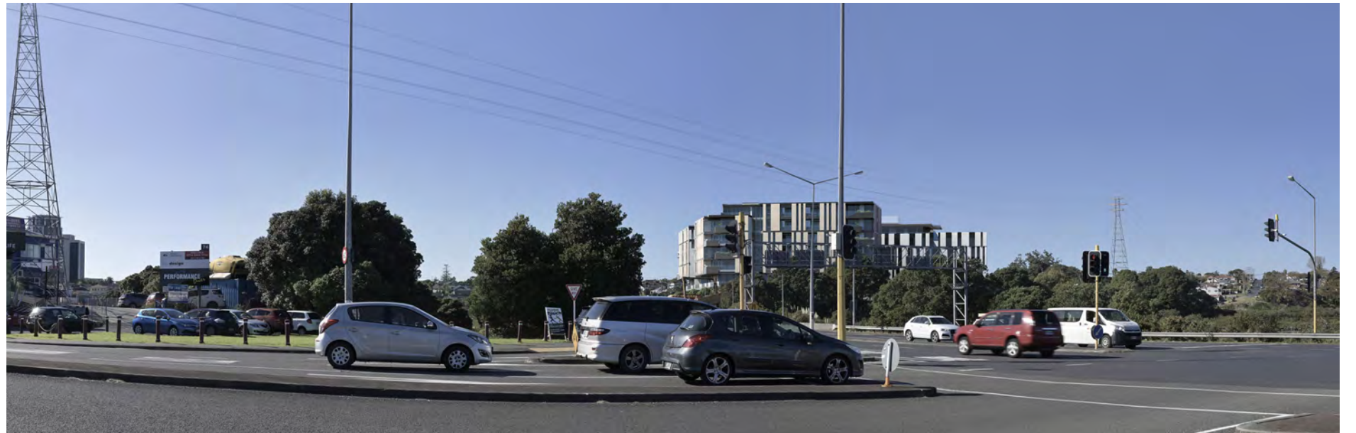
Buildings already received Resource Consent
