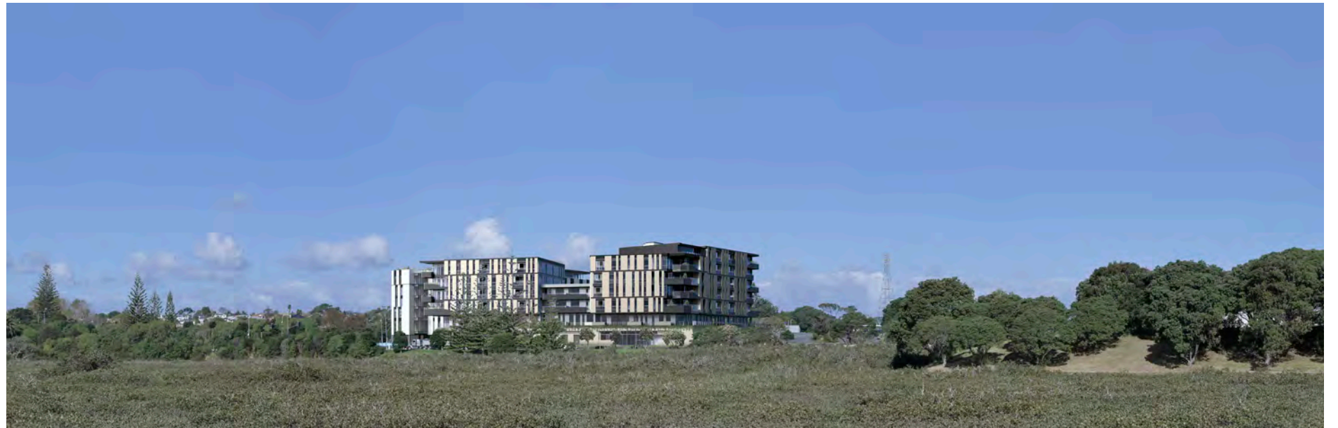
Buildings already received Resource Consent
