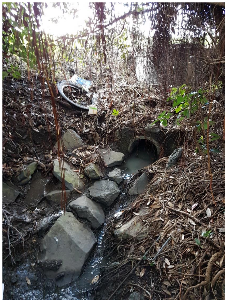
Existing Stormwater Outfall (SW 3)
