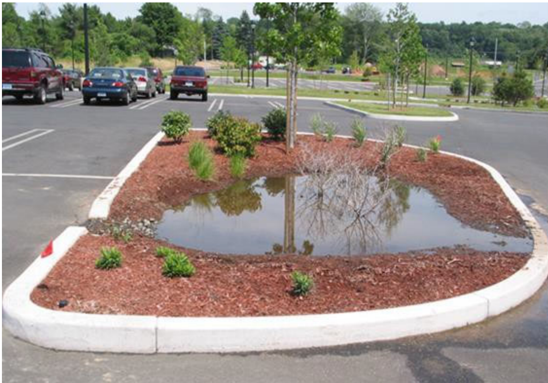
Figure 2. Rain garden media and inlet chamber may be blocked, ponding should not be visible after 1 day of dry weather. Maintenance overdue.
