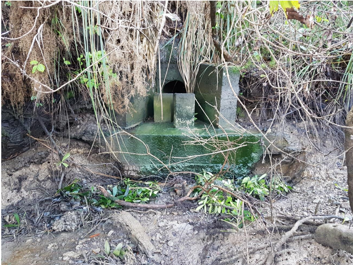
Existing Stormwater Outfall (SW 2)
