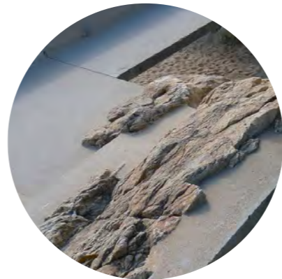
WALL TYPE 1 - RAISED PLANTERS CUSTOM IN-SITU STONE/ CONCRETE PLANTER (STONE SALVAGED FROM SITE)
