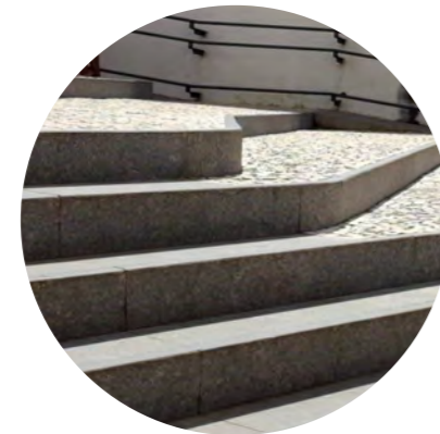
STEPS IN-SITU CONCRETE/ STONE PAVING
