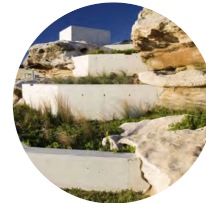
WALL TYPE 2 - RETAINING WALLS (OPTION 1) IN-SITU CONCRETE
