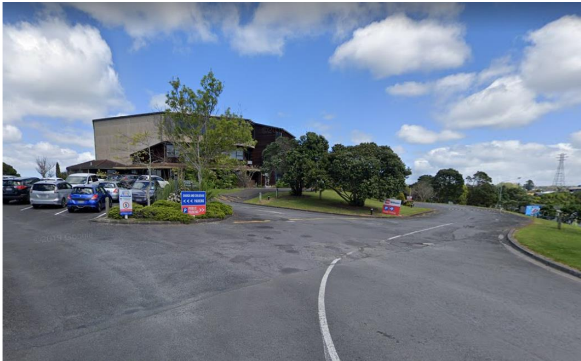
Photo 4: Photo of existing Church, 48 Esmonde Road, Takapuna (prior to construction)
