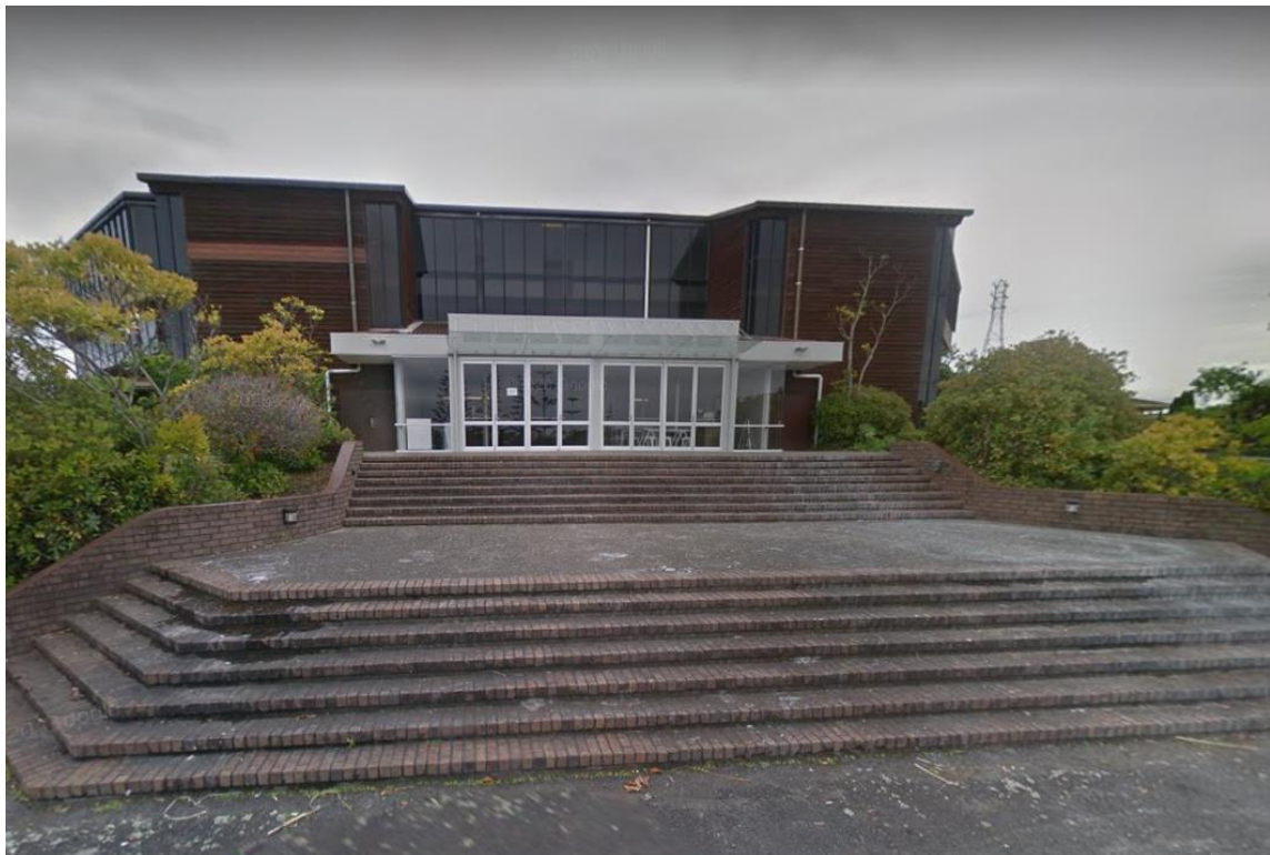
Photo 3: Photo of existing Church, 48 Esmonde Road, Takapuna (recently Demolished)
