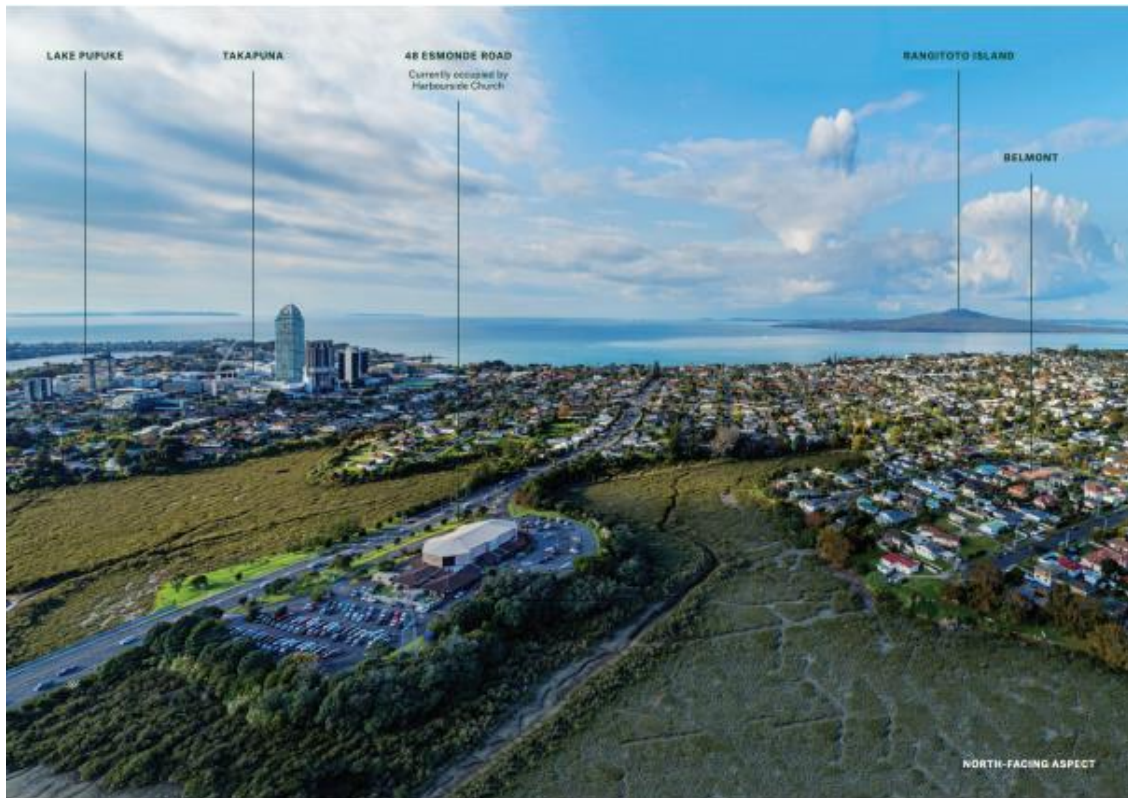
Photo 2: Aerial photo of site, 48 Esmonde Road, Takapuna (Prior to construction)
