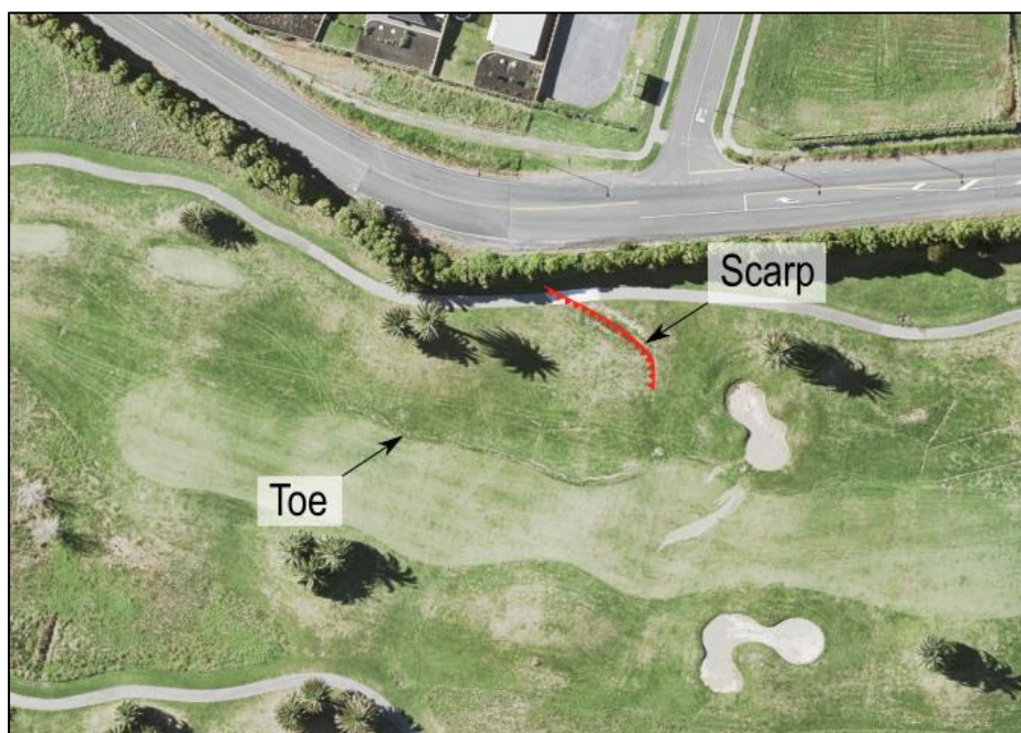
Figure 5: Aerial photo of slope failure adjacent to Jack Lachlan Drive
