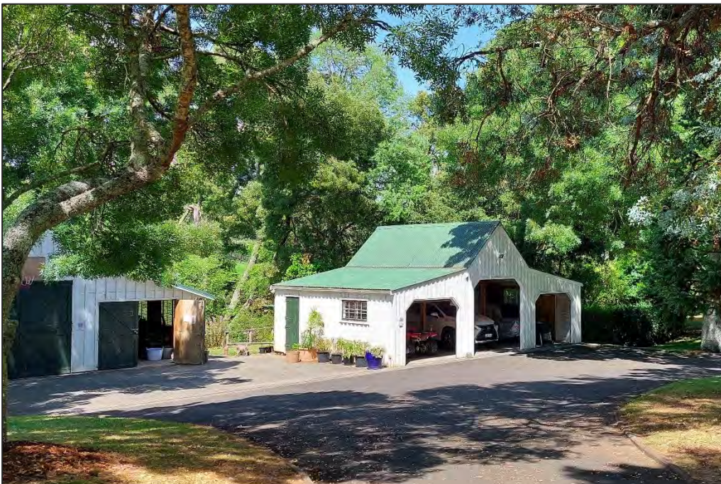
Photograph Appendix B.10: View south-west towards the storage shed and garage. Building materials were timber weatherboard and tin roof.
