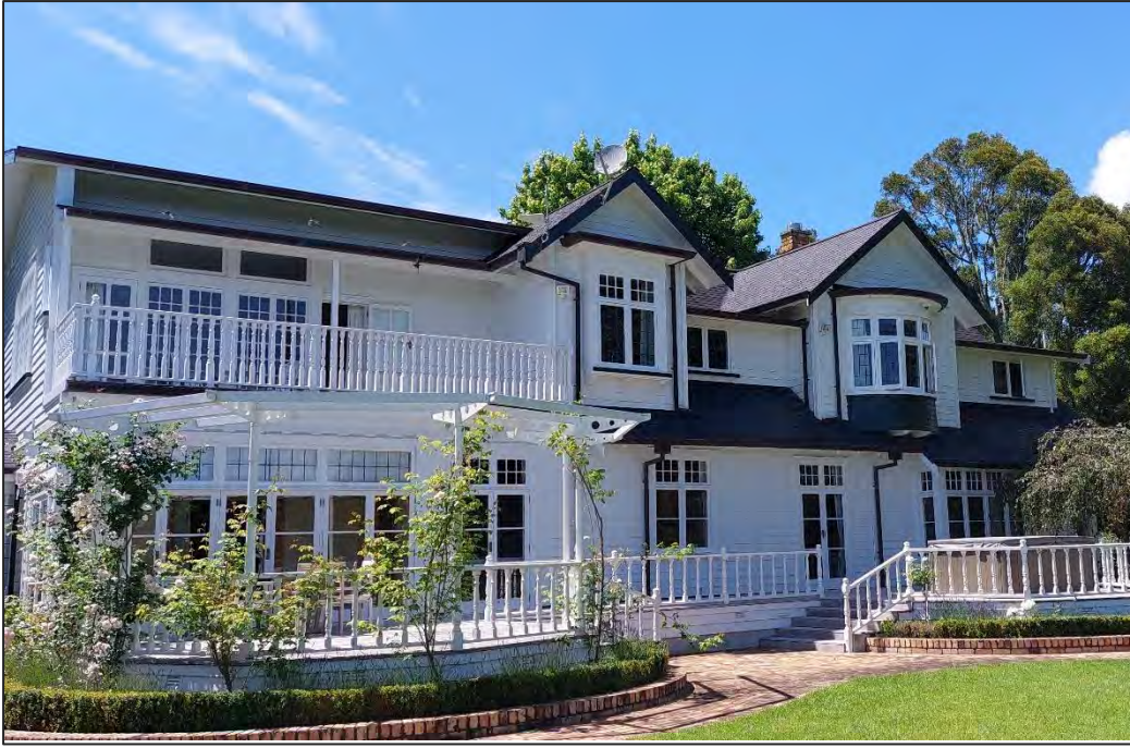
Photograph Appendix B.15: View south-east towards the residential dwelling. Building materials consisted of timber weatherboard, tin, brick and copper.
