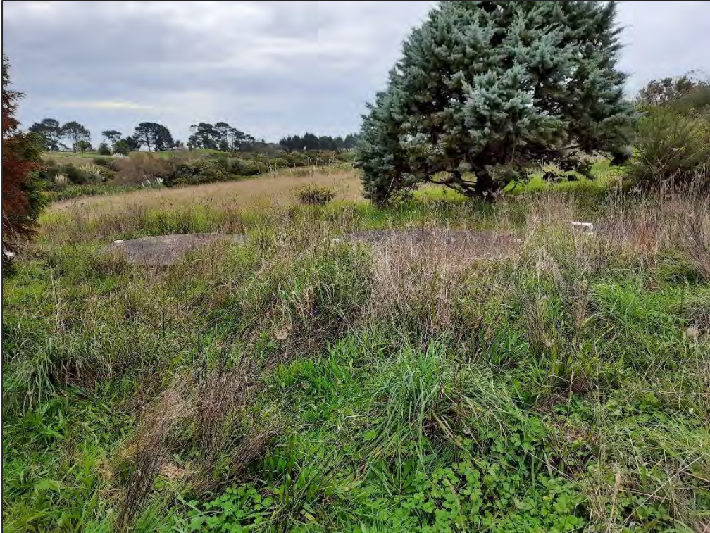
Photograph Appendix B.6: Close up of concrete settling tanks observed at the wastewater treatment station.
