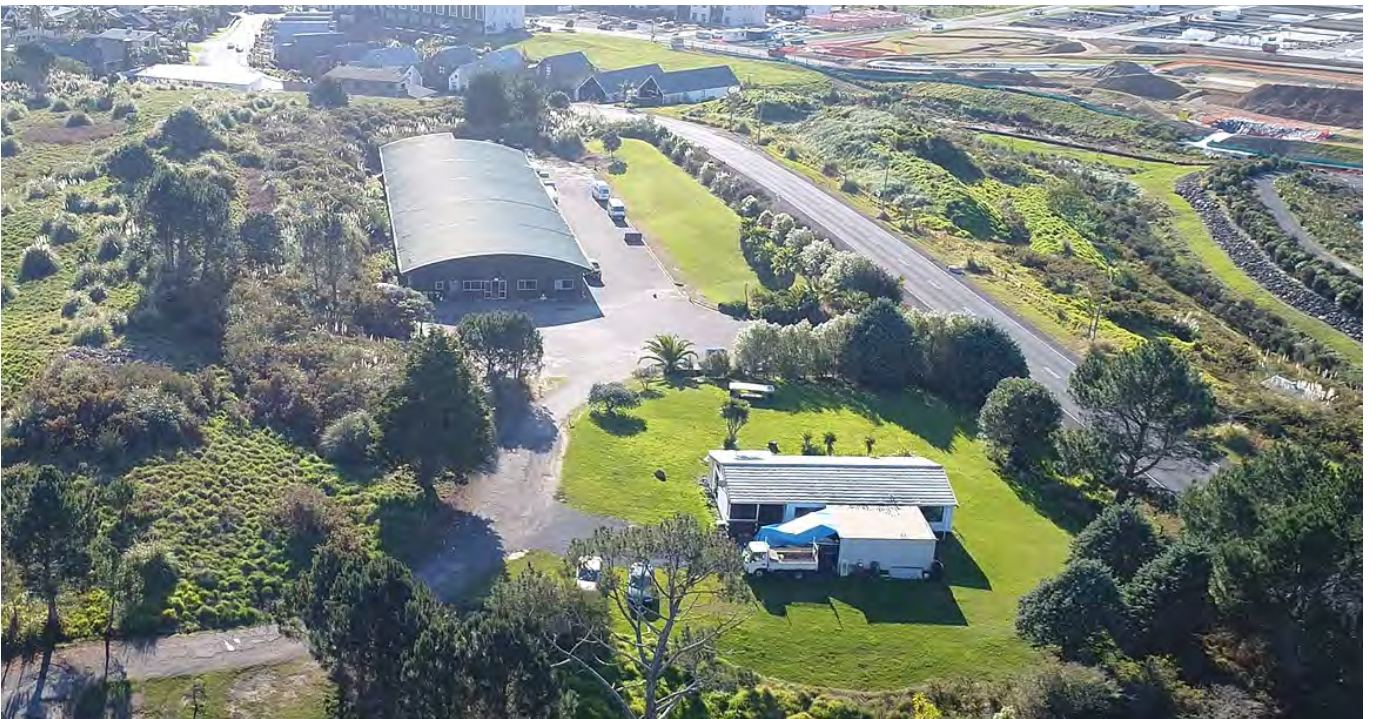
Figure 10. Existing golf maintenance buildings and single house
