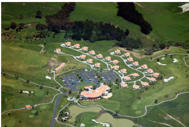
Figure 8. Existing golf club house building and adjacent visitor accommodation villas
