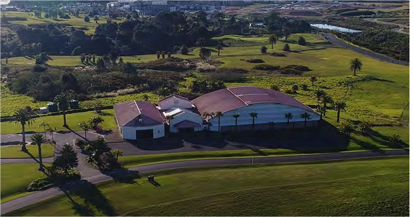
Figure 9. Existing sports and recreation building
