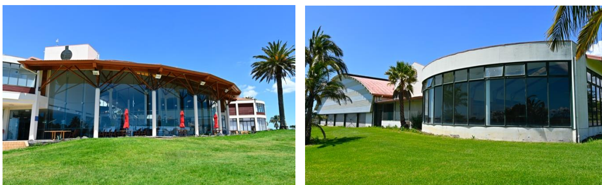
The current golf course 'clubhouse' (left) and recreation centre (right)
