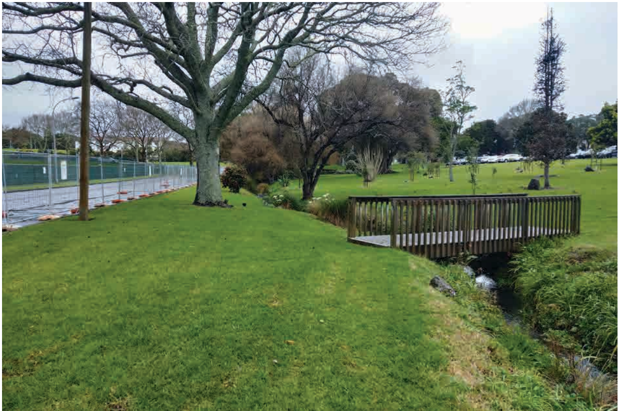
Figure 16. View southeast along Farm Road and stormwater trenching alignments to Wairaka Stream.
