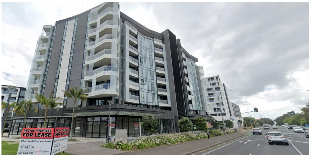
Figure 6: 9 storey apartment buildings with retail ground floors on Greenlane West.
