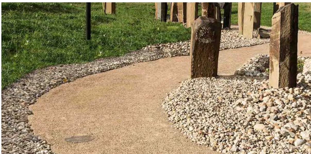
Constructing a 1.8-meter-wide path along the existing alignment of approximately 33m with Organic-Lock (exclusive of all works till subbase level) will have an estimated cost of approximately \$6000 (100/m<sup>2</sup>).
