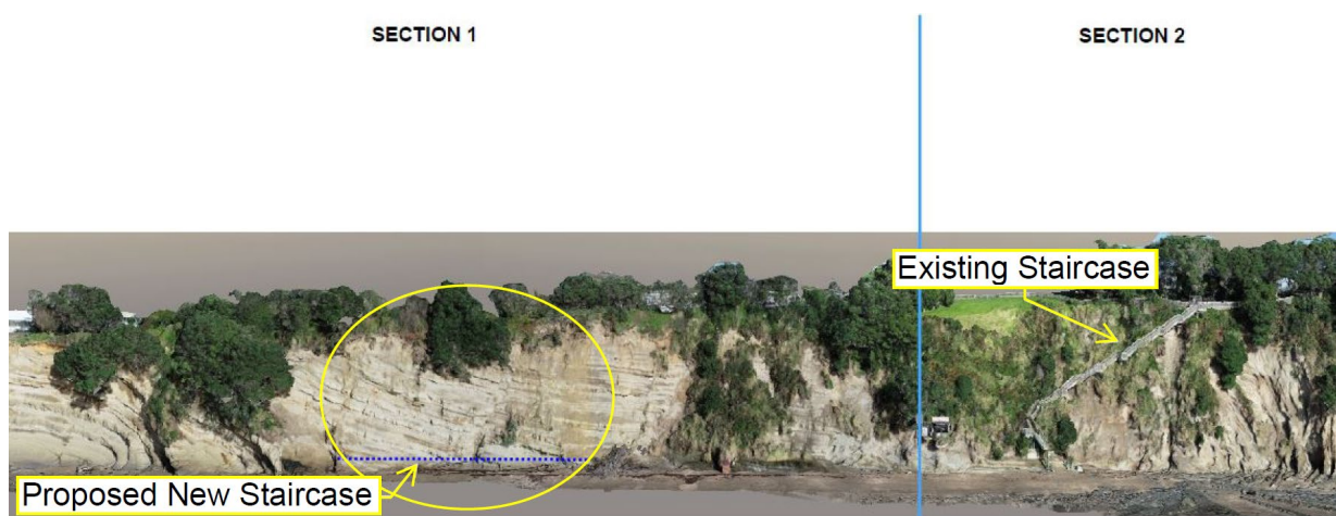
Figure 7: Kennedy Park potential location to relocate and rebuild a new staircase
