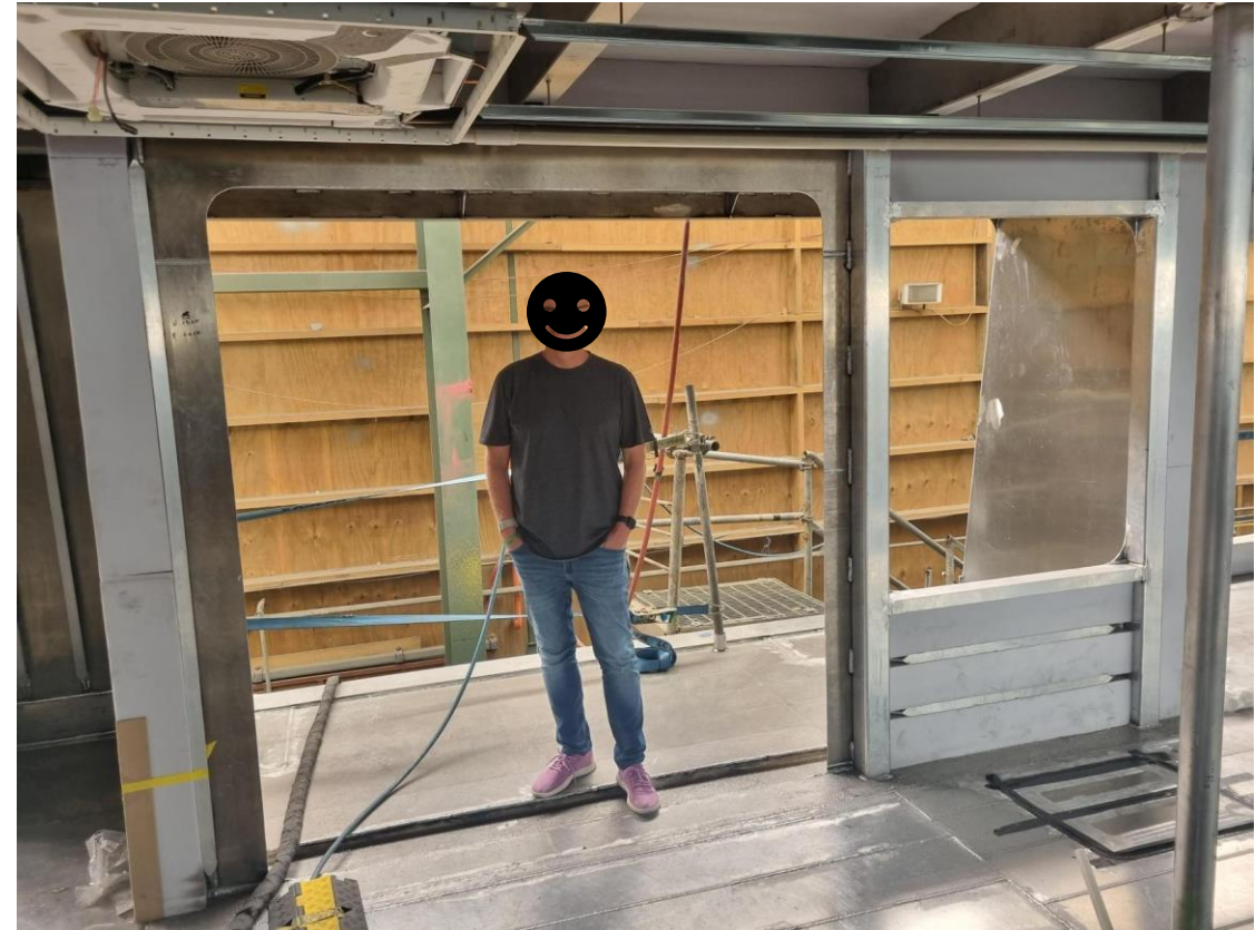
Wide central boarding door framing
