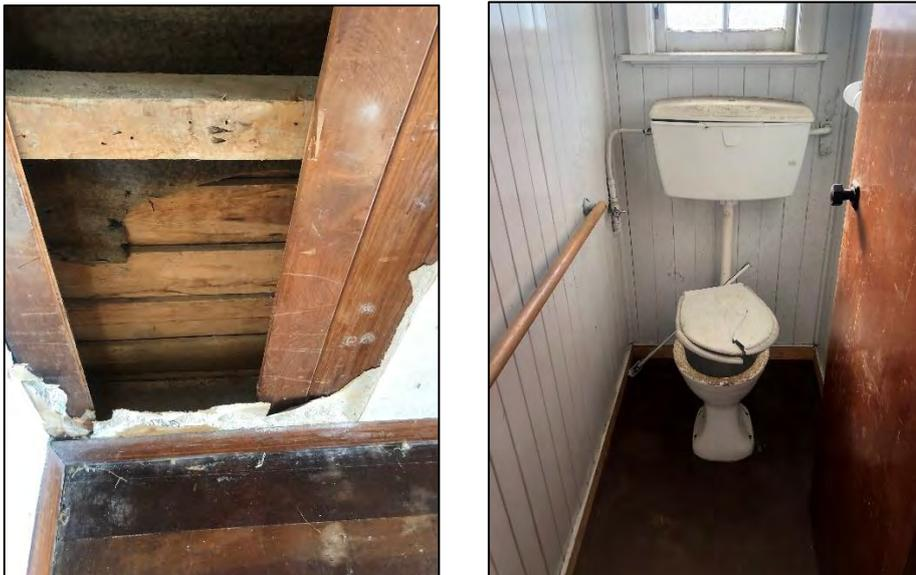
Area where plasterboard has been removed, exposing original tongue and groove linings (left) and toilet with tongue and groove boards still in place (right).
