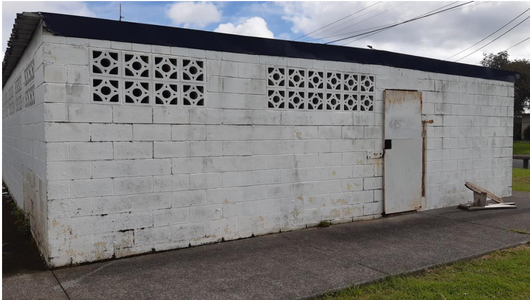
Image 6: Masonry building – requires further earthquake investigation if renewed
