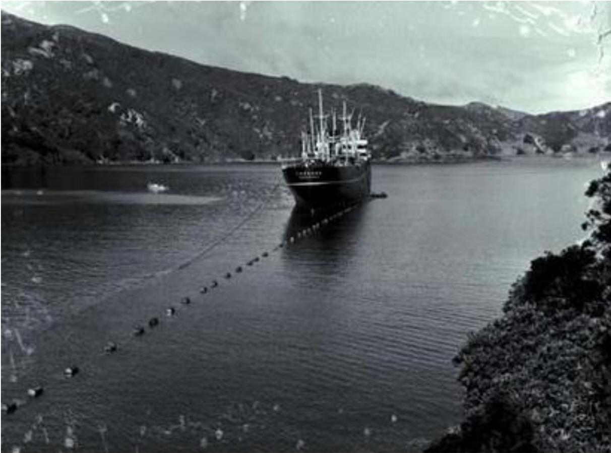
Figure 122. Whale oil being pumped to the vessel *Tirranna* in Whangaparapara Bay. The pipeline is supported by a combination of 44-gallon drums and reused harbour defence buoys. (AWMM/L PH-NEG-H51).
