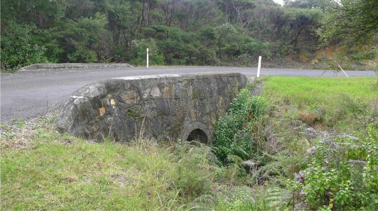
Figure 32. One of the stone culverts built by stone mason relief workers in the early 1930s. (Auckland Council July 2017).
