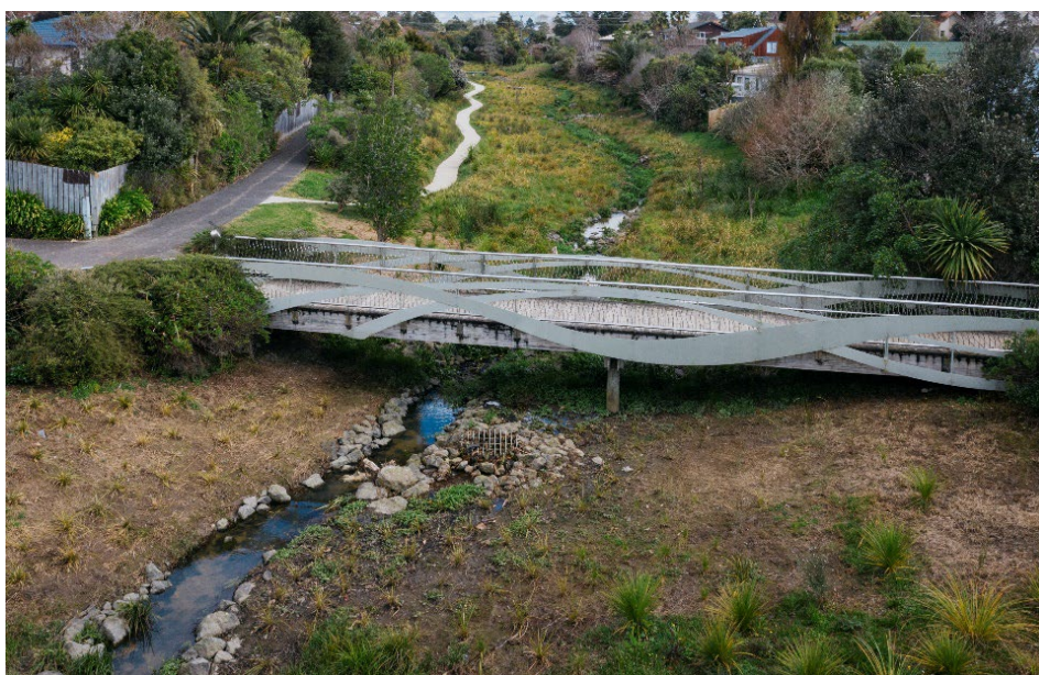
Daylighted/naturalised stormwater infrastructure - Whenua-roa / D'Oyly Reserve
