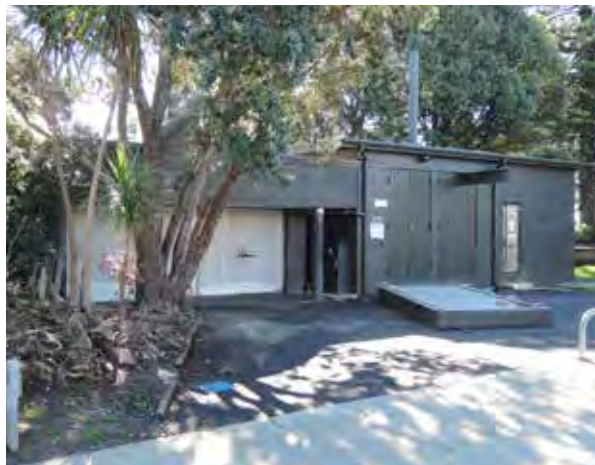
⑦ The existing Watercare wastewater pumping station on Sidmouth Street
