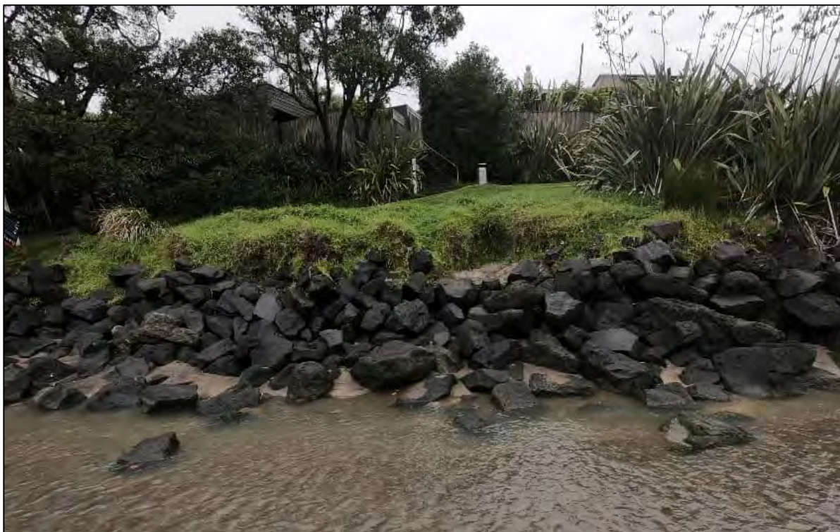
Figure 3.4: Haphazardly placed rock armour
