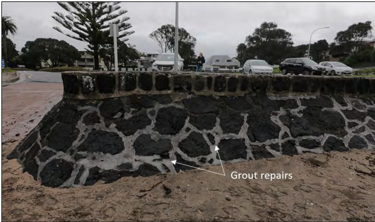
Figure 3.2: Example of grout repairs
