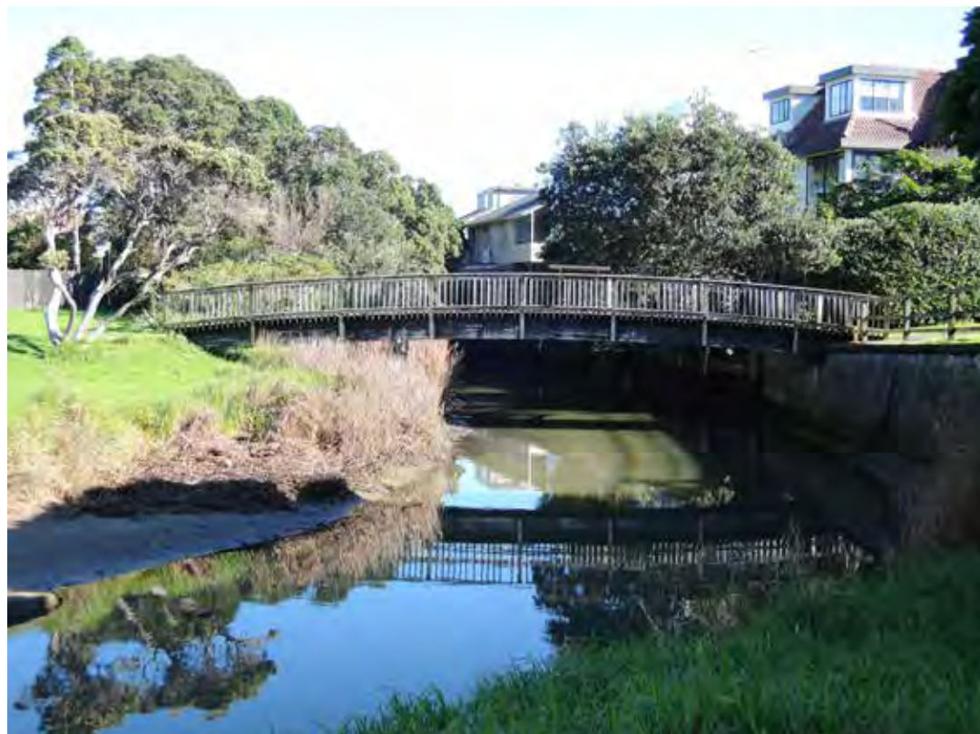
Fig 19 Existing bridge connection between Mairangi Bay Reserves and Whitby Crescent walkway
