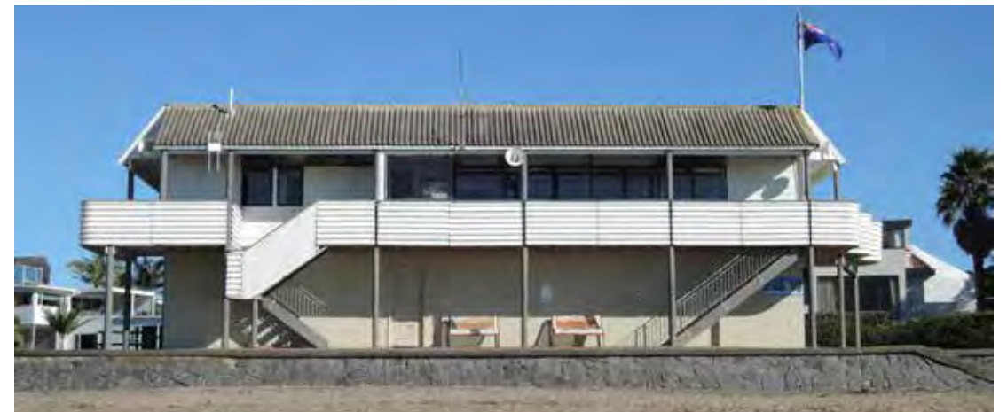
⑥ Mairangi Bay Surf Lifesaving Club current facility
