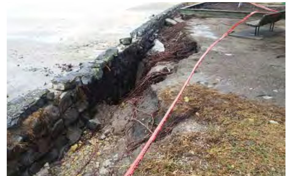
Fig 6 Sea wall damage as a result of onshore storm surge and high tide (5th January 2018)
