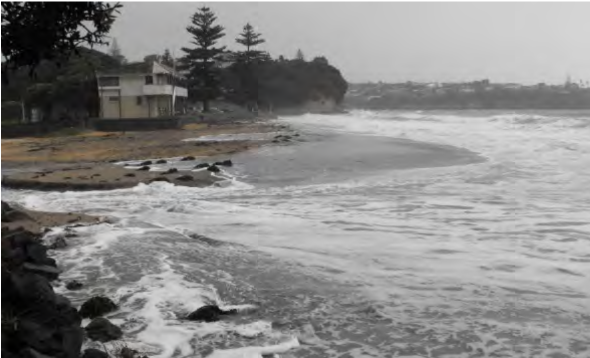
Figure 1 above – the surf club during a 2016 storm event (source: Matt McNeal, Auckland Council)
