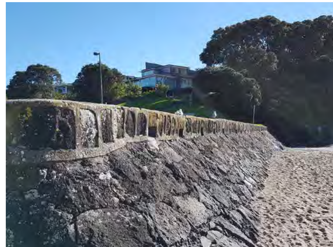
Fig 22 Seawall by the Mairangi Bay boat ramp
