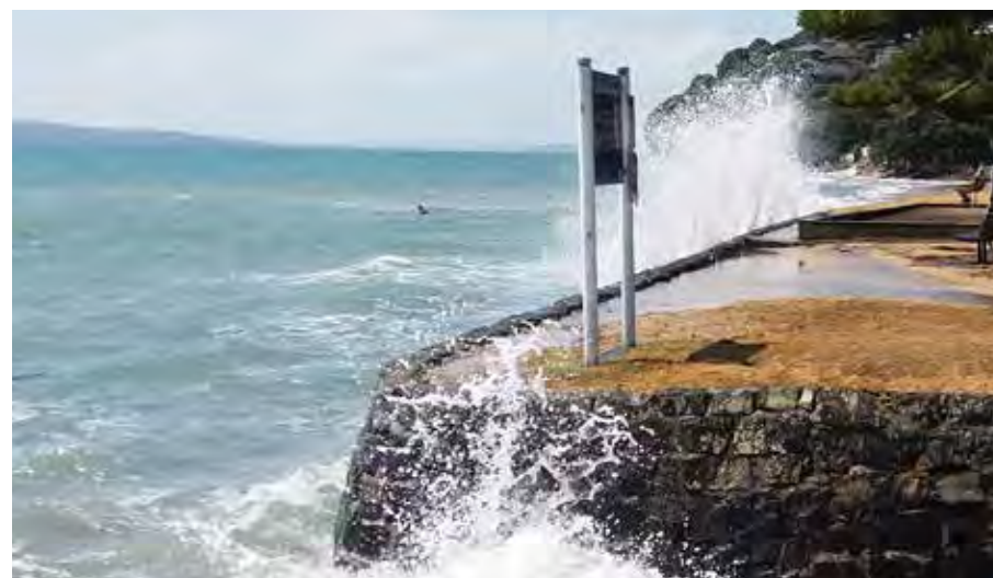
Fig 8 King tide overtopping sea wall (7th December 2017)
