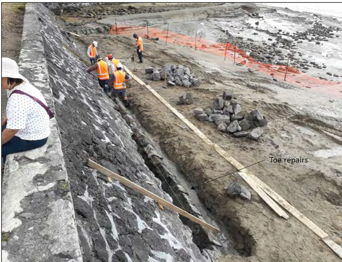
Figure 3.3: Example of toe repairs to the seawall
