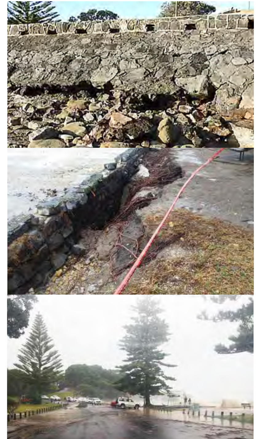
Fig 13 Examples of coastal erosion and damage following storms/king tides
