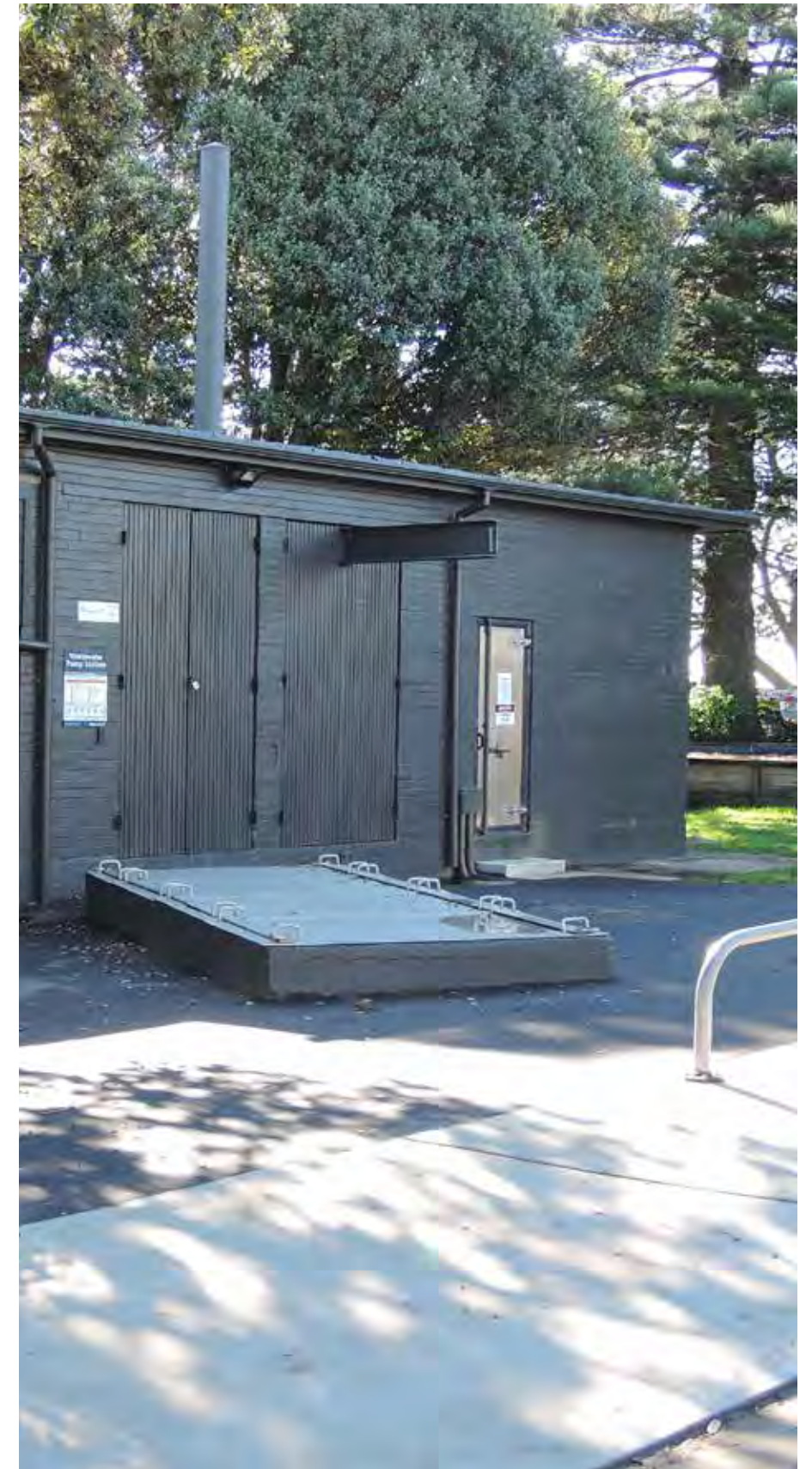
Fig 11 Sidmouth Street Watercare pump station
