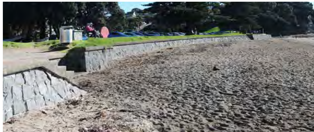
⑤ Existing coastal seawall with steps inserted for beach access
