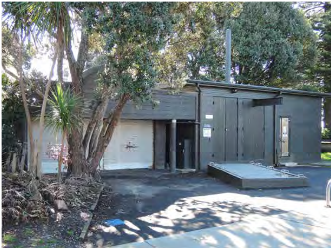
Fig 21 Existing Watercare Pump station on Sidmouth Street
