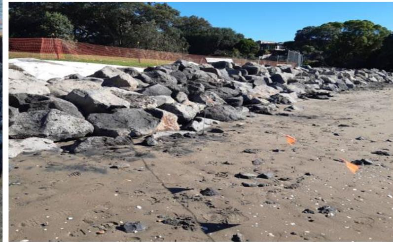
Placing rocks over geotextile membrane
