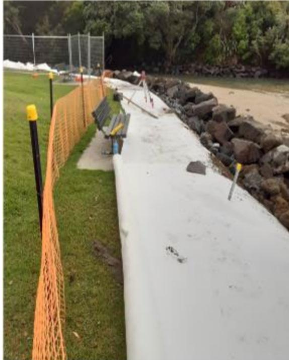
Placing rocks over geotextile membrane
