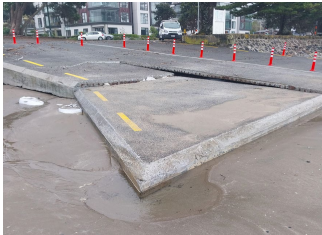
Fig. 1 – Collapsed section of ramp.
