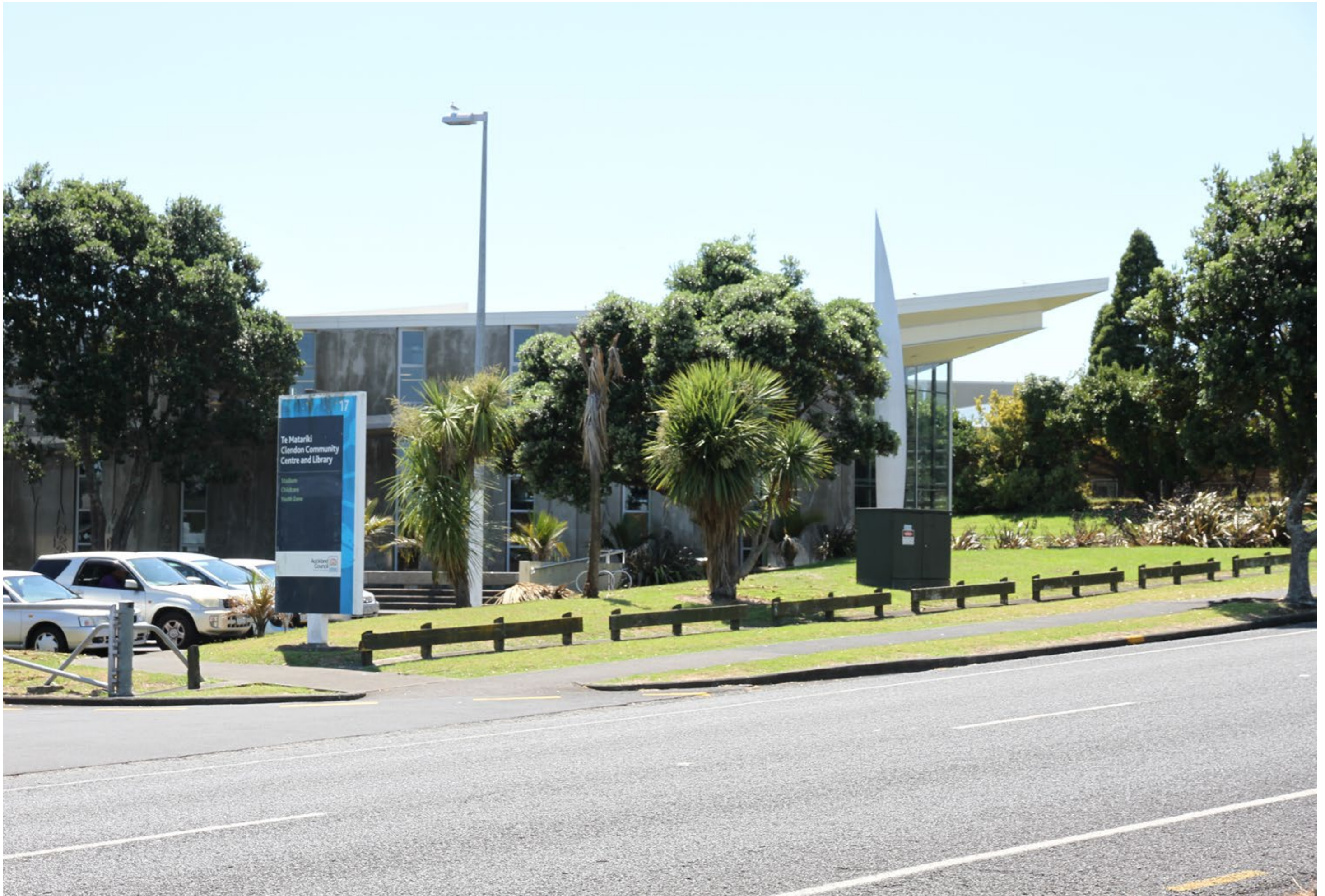
Te Matariki Clendon Community Centre and Library
