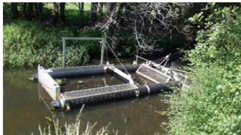
*Litter trap before and after debris removal*
