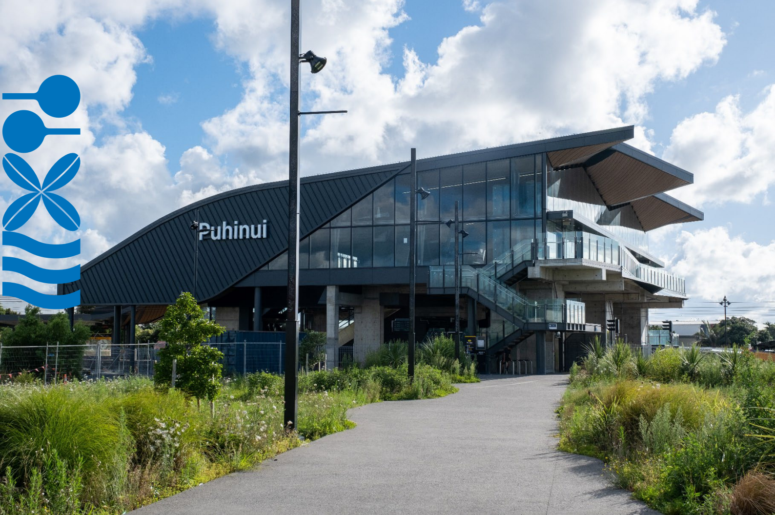
Puhinui Train Station
