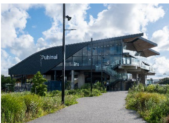
Puhinui Train Station
