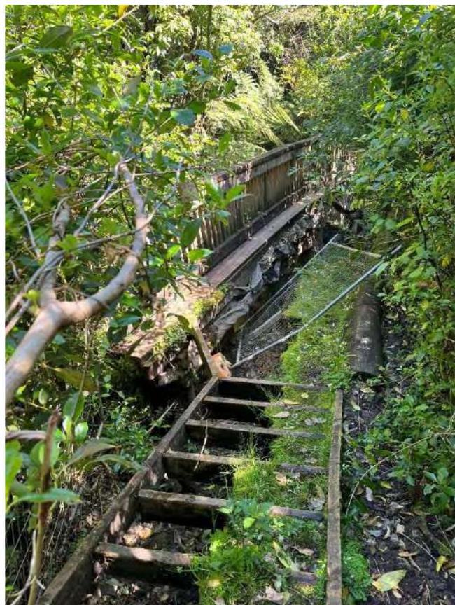
Figure 29: Belfast Reserve - Failure of retaining wall from stream scour
