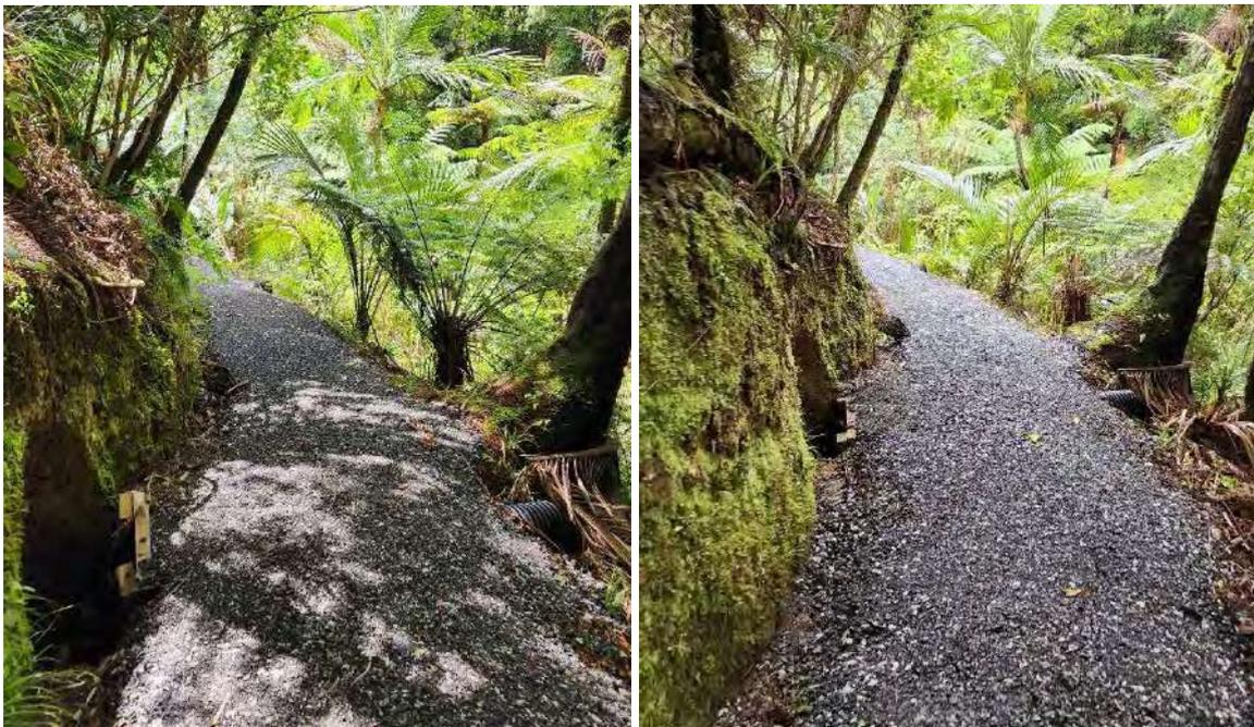
*Figure 32: Aggregate track with side drain and culvert*
