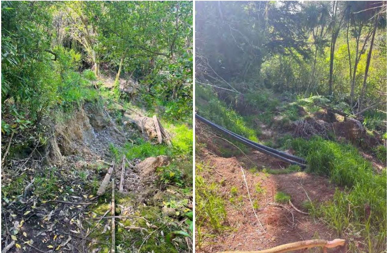
Figure 28: Belfast Reserve - Slip through track alignment
