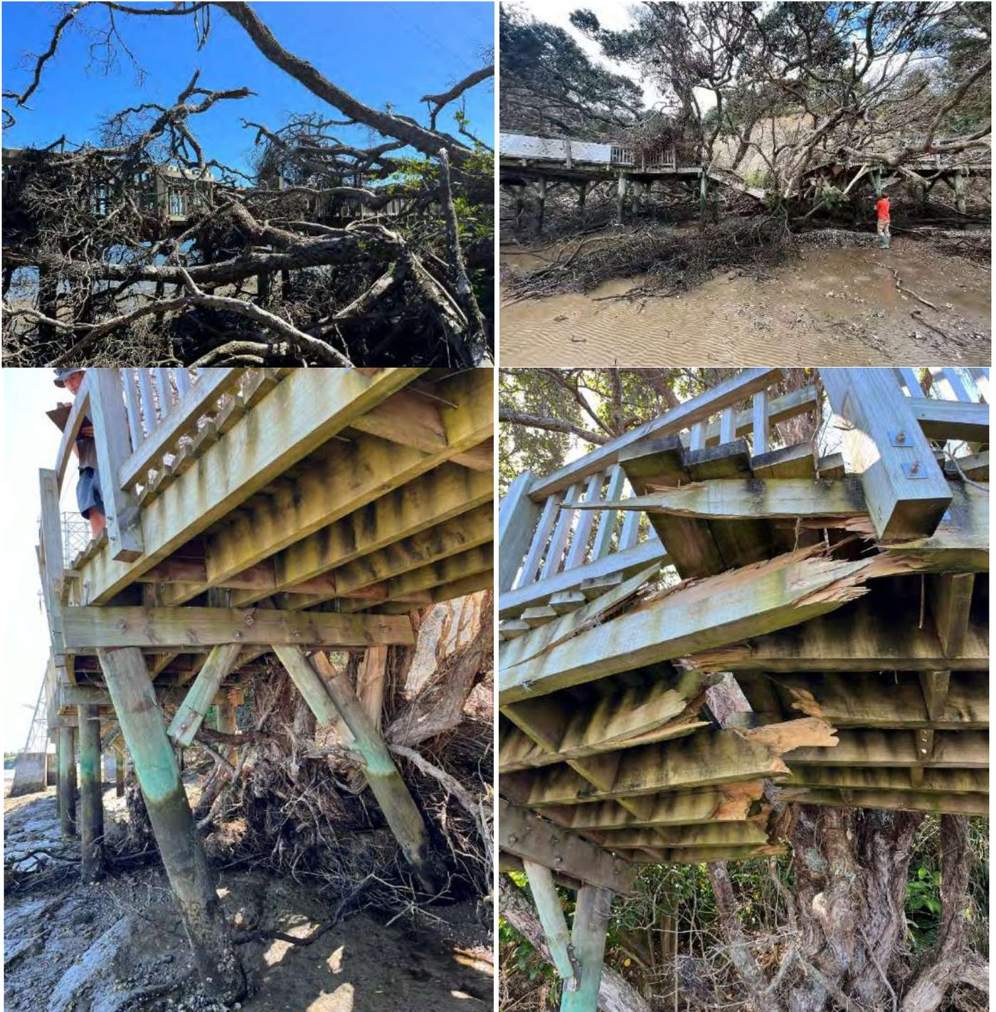
Figure 31: Manukau Coastal Walkway - Slip damage to coastal walkway
