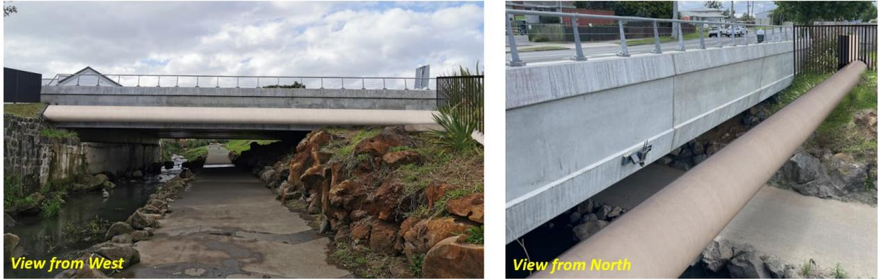
19. The presence of the pipe crossing over the stream may have a visual impact on the surroundings. Mitigation is proposed by painting the pipe and potential planting screening on both sides of the pipe to make it sympathetic with the surrounding landscape.
