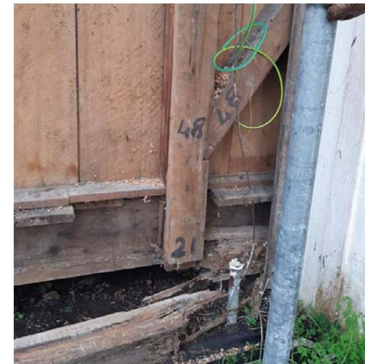
**Above:** Completely decayed bottom plate, unsupported by floor joists. Numbered timber indicating relocation
