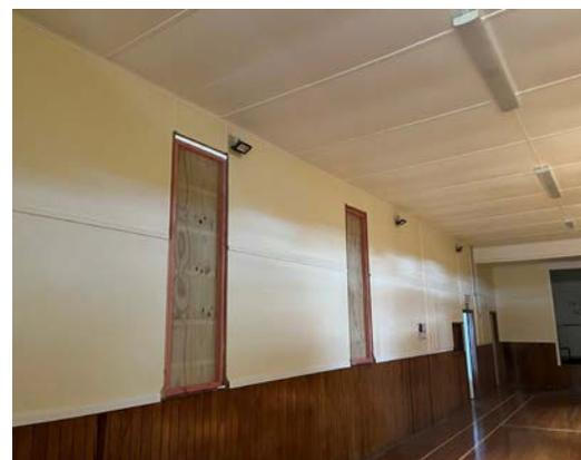
Left: Rotten windows have been removed and will be replaced with new windows.
