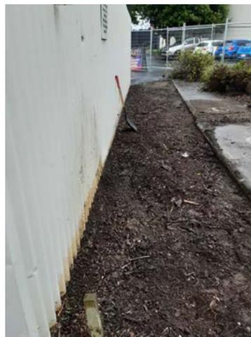
**Above:** Previously covered exterior metal cladding exposed for treatment and repainting
