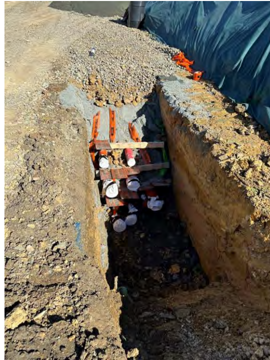
• CST installation Phase A
