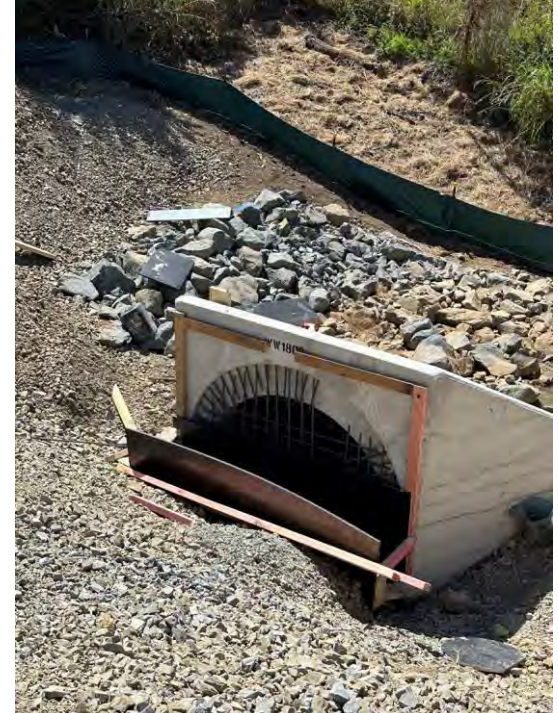
• Headwall installation
