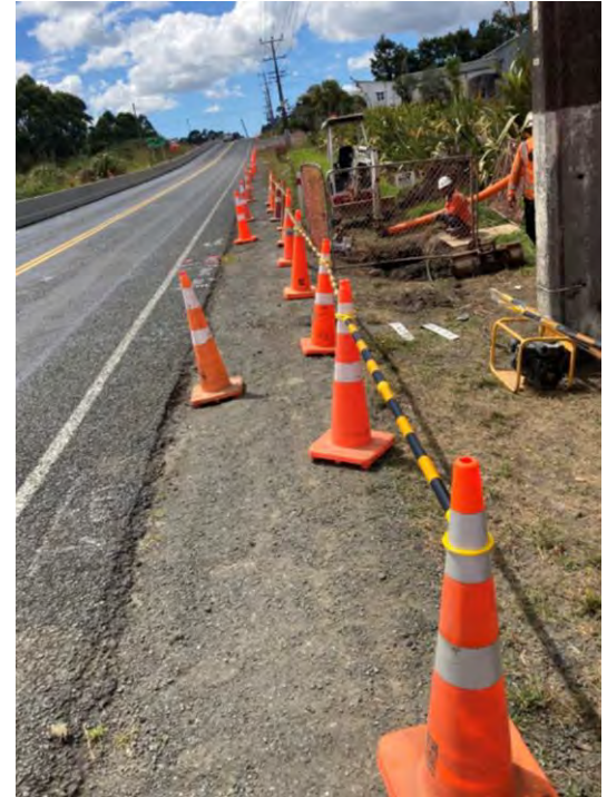
• Drilling beneath road
