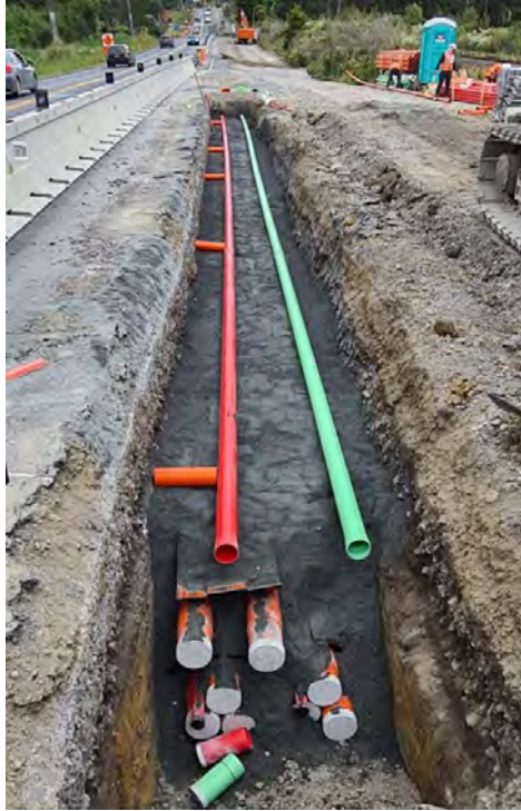
• CST installation in Phase B
