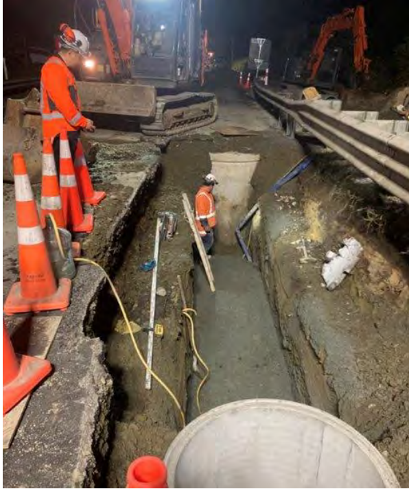
• Night-time drainage installation
