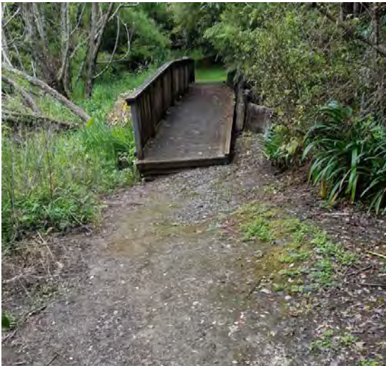
Photos Below: Pre renewal work
