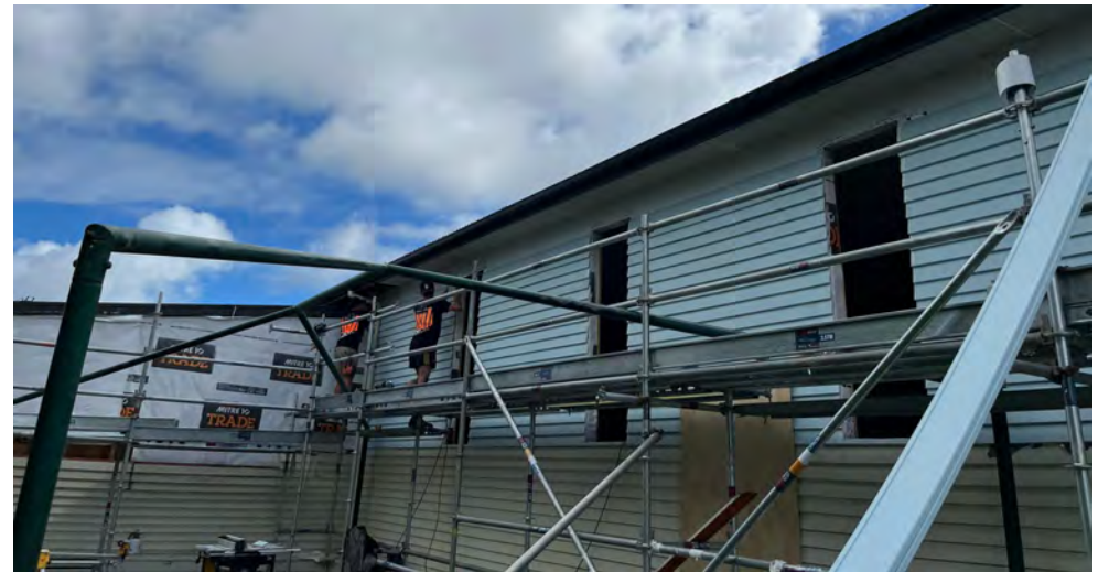
Above: Asbestos removed and reclad underway
