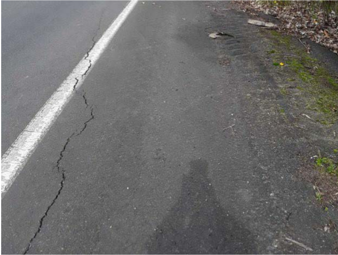
Figure 2: Cracking present on SH16 due to landslip
