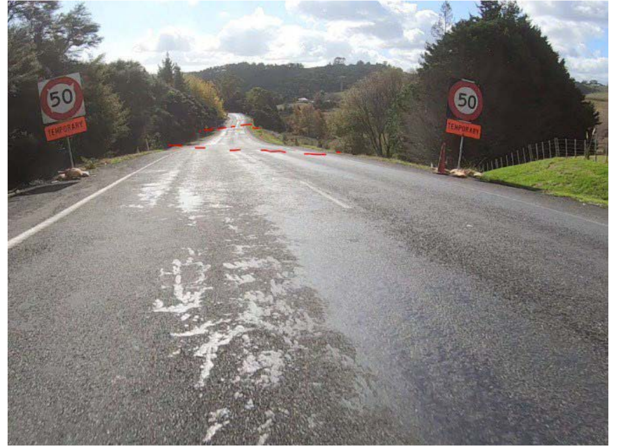
Figure 3: Subsidence present on SH16 due to landslip
