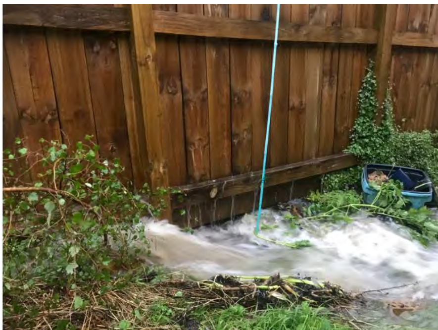
Overland flow blocked by a fence
