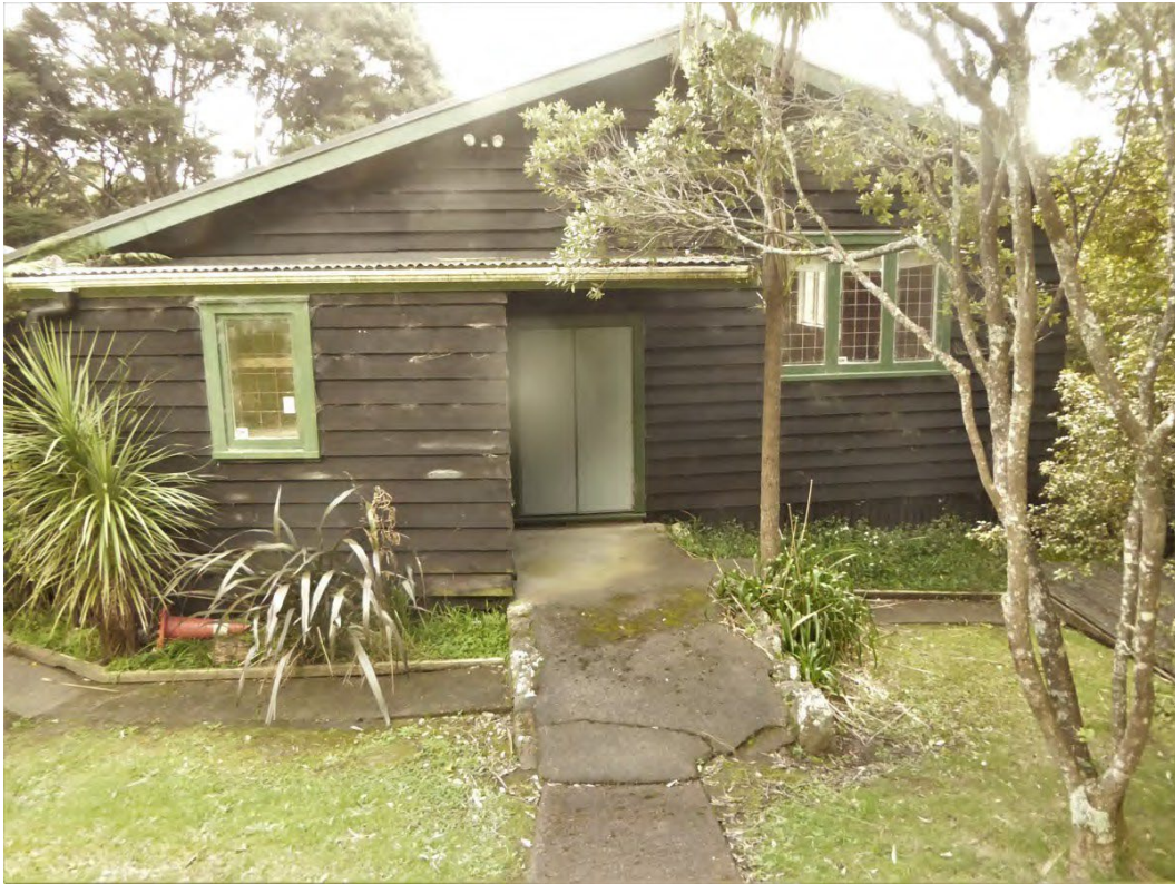
Redundant scout den on Atkinson Road needs repurposing.
