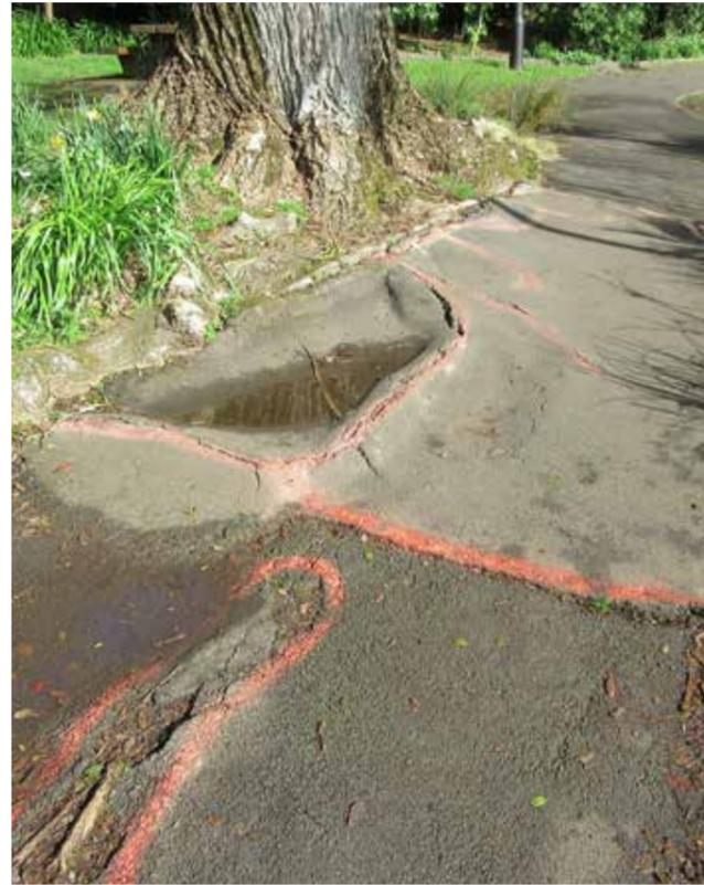
Cracks on some sections of main pathway due to tree roots
