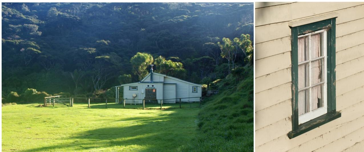
**Image on Left:** Liebergreen Cottage, Whatipu. Heritage building in Auckland Council ownership and part of the built heritage survey carried out by DPA Architects. **Image on right:** shows breakdown of the exterior paint system on the window frame. (Source: DPA Architects)
