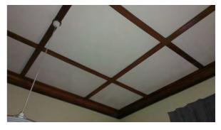
Figure 6: Timber batten ceiling (Auckland Council, 2013)
