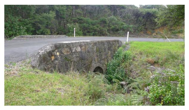
Figure 32. One of the stone culverts built by stone mason relief workers in the early 1930s. (Auckland Council July 2017).
